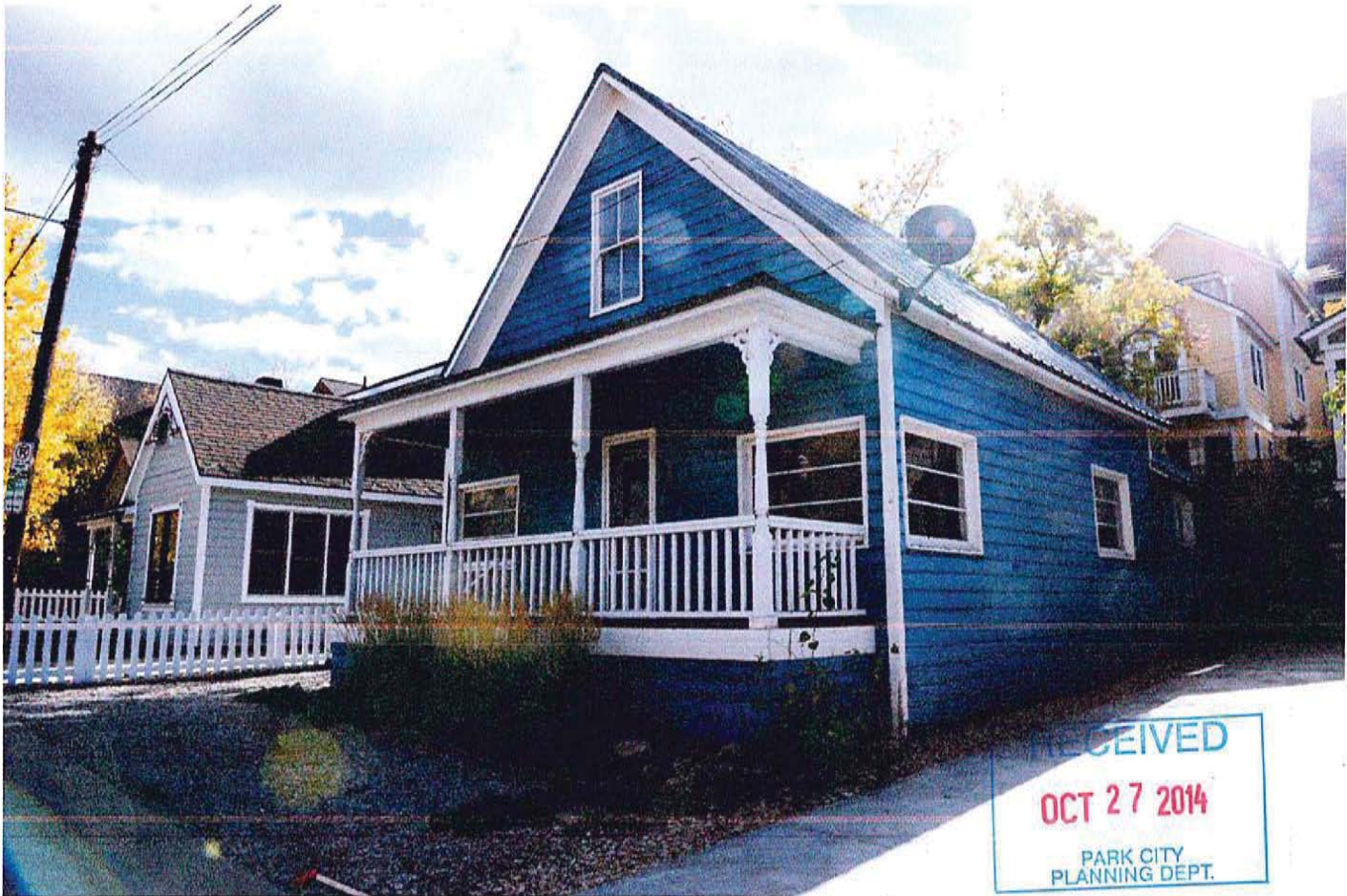
923 Park Avenue – Facing Southwesterly
