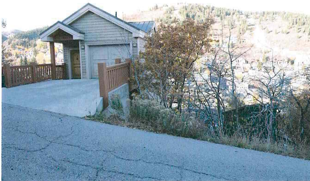
347 & 355 Ontario Avenue looking west
