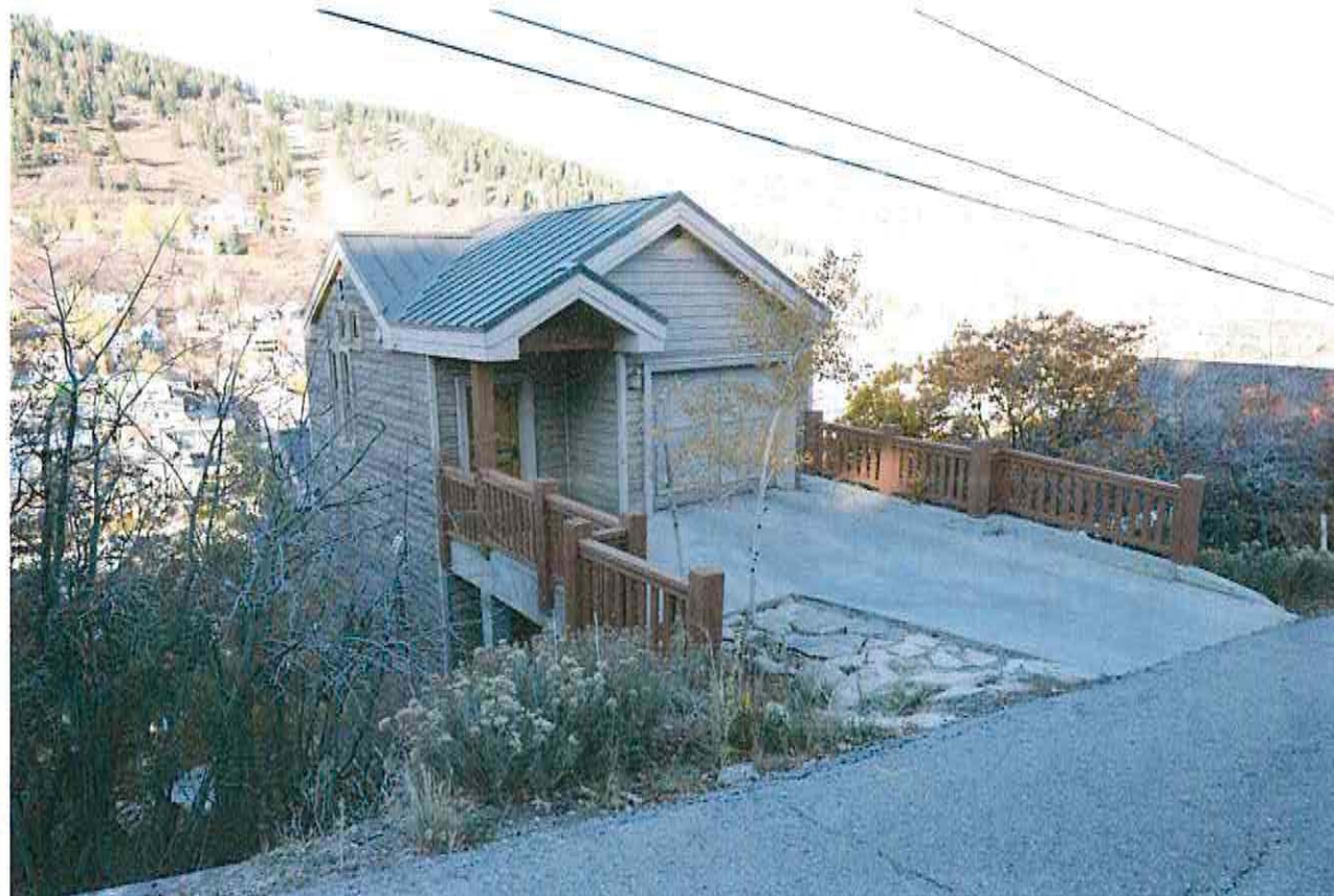
347 Ontario Avenue looking west
