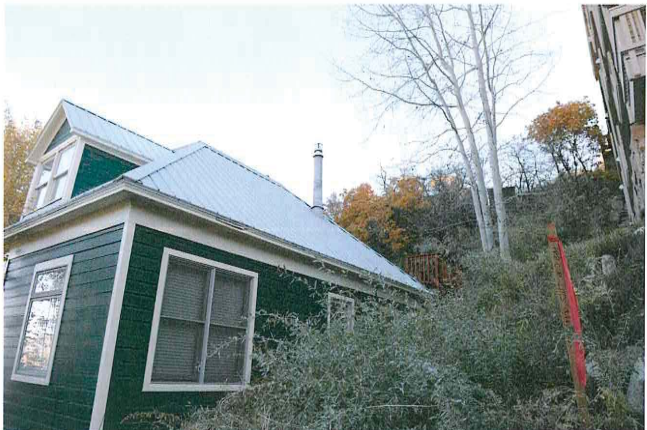
355 Ontario Avenue looking east
