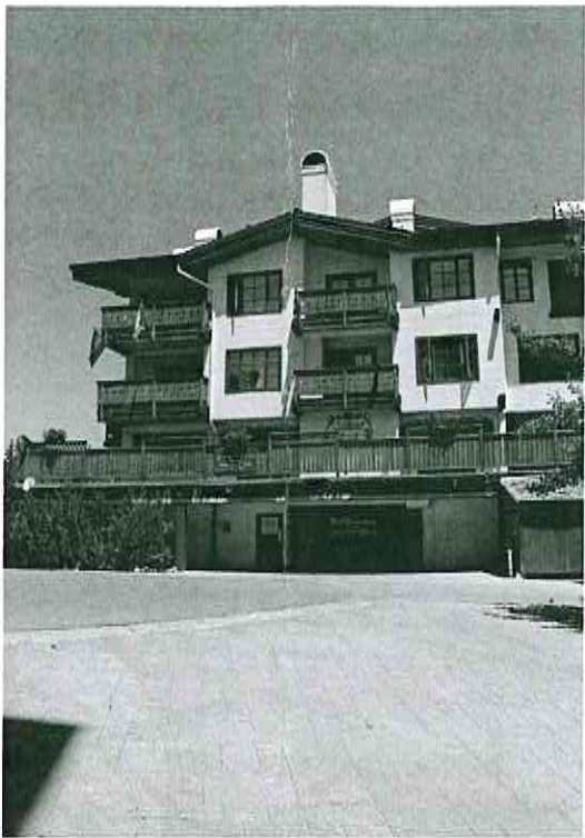
02_Hirsch garage entrance at Sterling Ct
