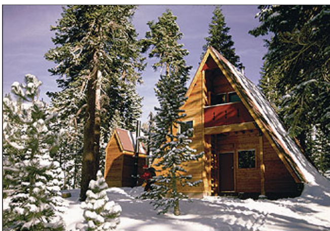
The Sierra Club was an early adopter of the A-frame—a house form that fit snow as well as shore. The Bradley hut, built in memory of past Sierra Club president Josephine Crane Bradley, was dismantled in 1997 and reconstructed four miles from its original site.
