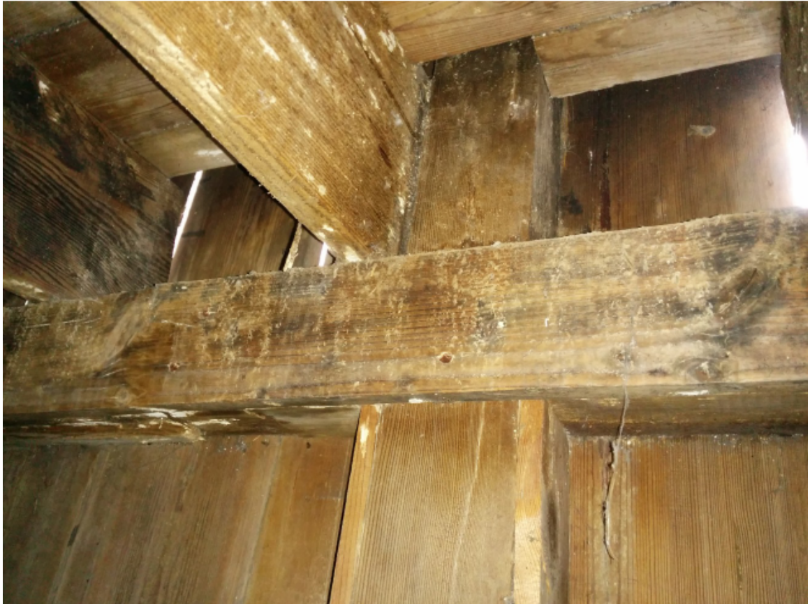
Figure 4. Column to beam connection
