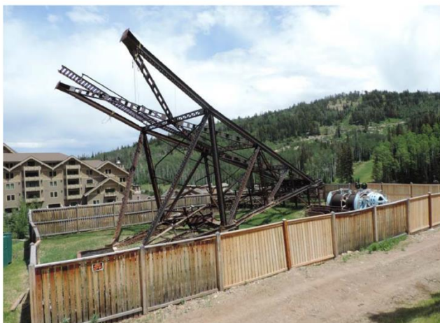
2: Collapsed Daly West Headframe
