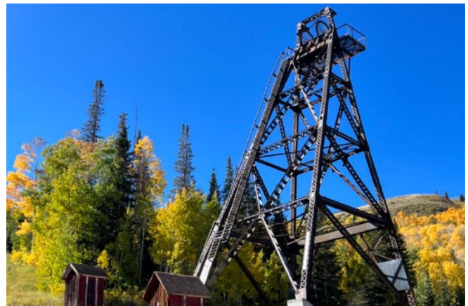
1: Restored Daly West Headframe
