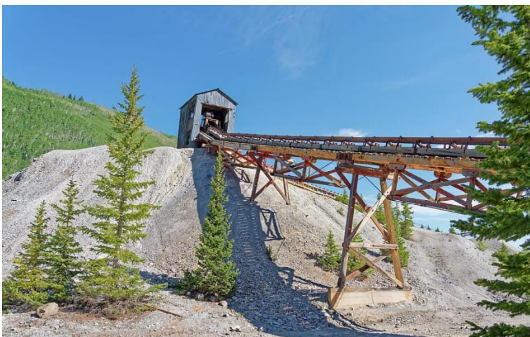
Figure 6. Thaynes Conveyor Gallery, 2021
