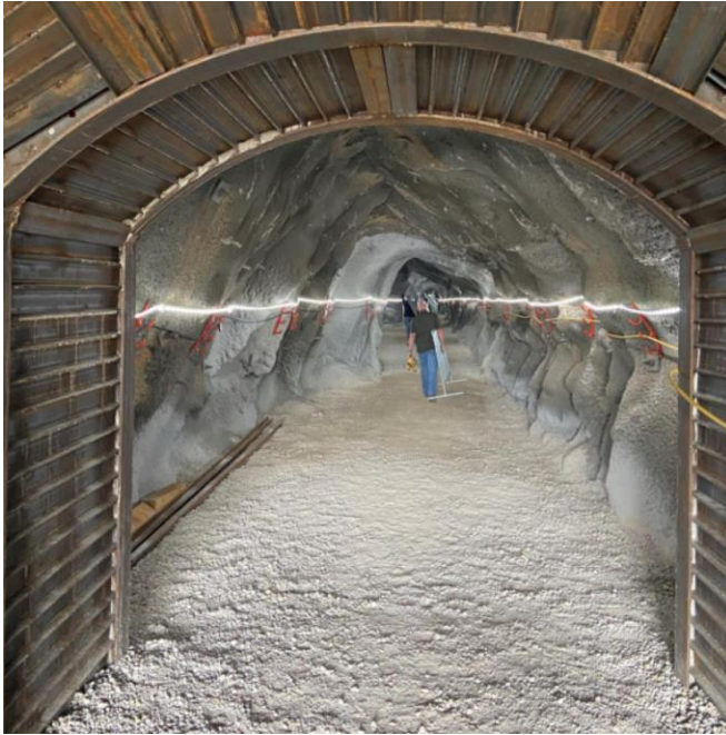
Figure 2. Inside the Spiro Tunnel, October 2021
