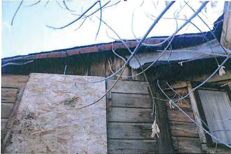
Northeast window fixed 2'-8"W X 2'-2"H 3'-8" off floor-casing unknown Northwest window fixed 1'-5"W X 2'3"H 4'-4" off floor-casing 1X4 wood
