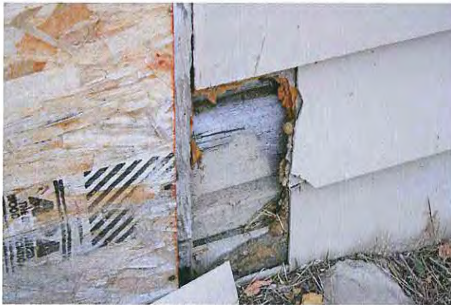
6. Siding detail-northwest gable north elevation
