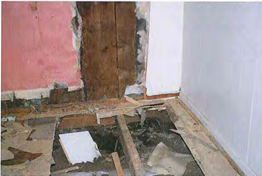
1.Look at interior excavation north wall
