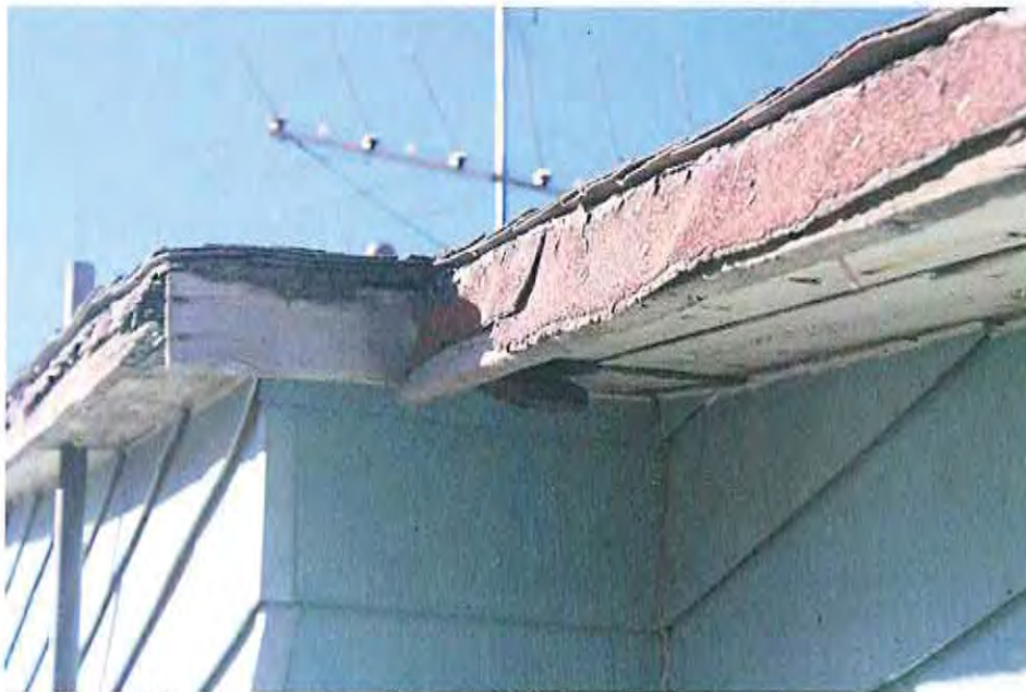
Soffit and fascia southeast corner kitchen/bathroom
