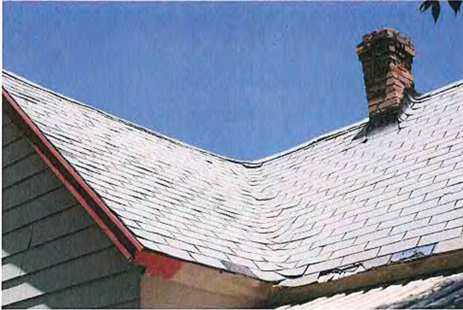
4.Original roof valley and chimney
