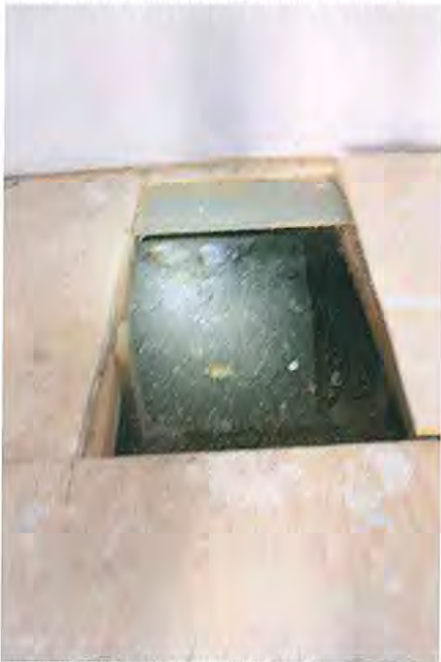
Foundation-floor joist on rubble stone
