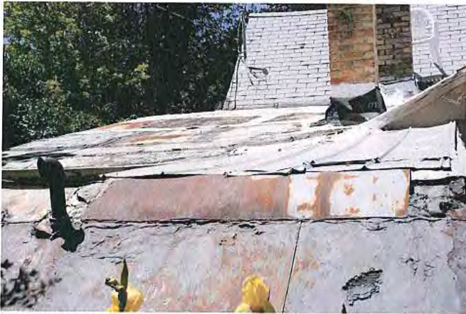
Root cellar roof in foreground.
