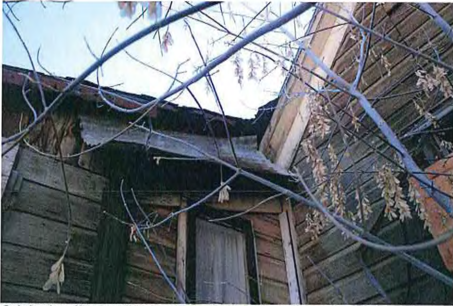
Original soffit and fascia on east side of north-south gable. Intersecting shed roof and soffit and fascia has water damage and layers of makeshift repairs.
