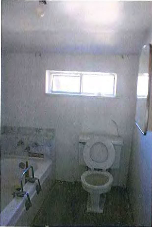
East bathroom window-modified casing
