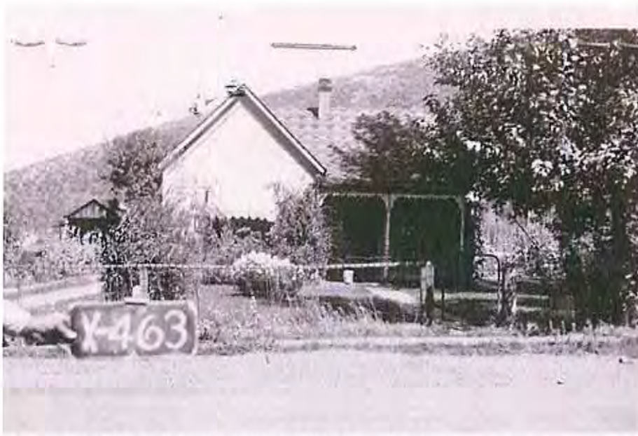
Historic front porch structure on 1450 Park Ave.
