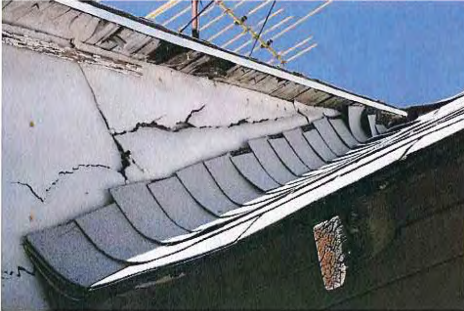
6. East elevation overbuild at bathroom
