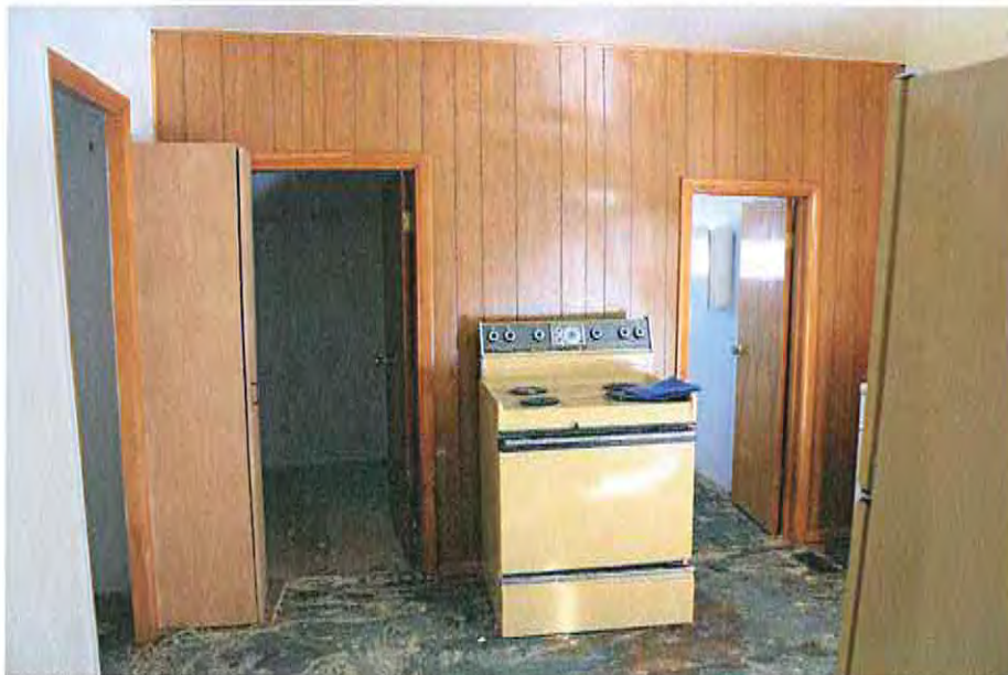
Typical interior door and casing
