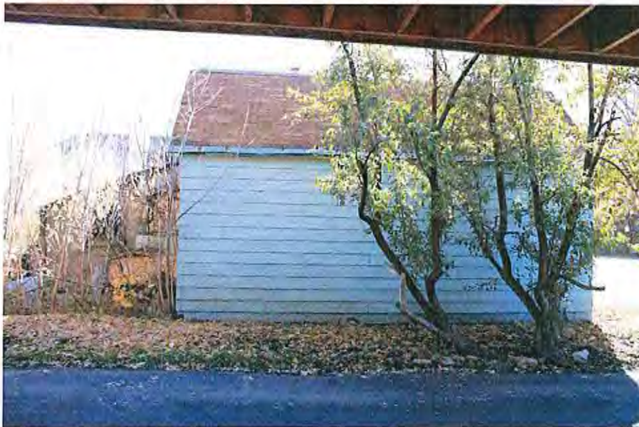
East-west gable roof
