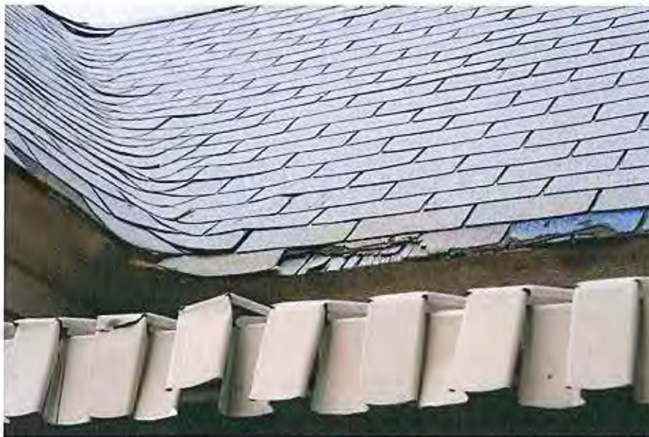
1. Original wood shingle
