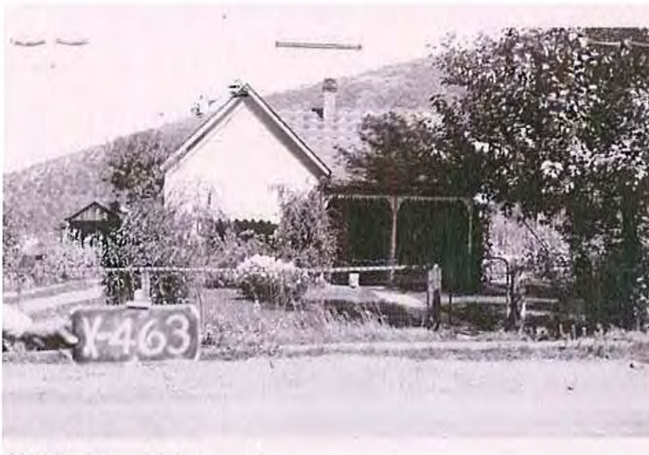
1450 Park Ave. Historic porch
