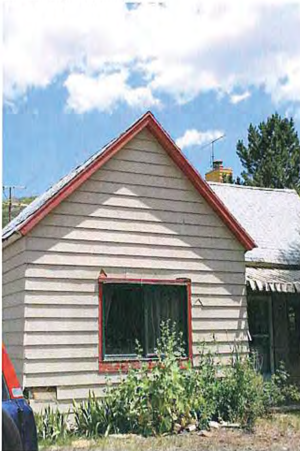
3.Original west gable
