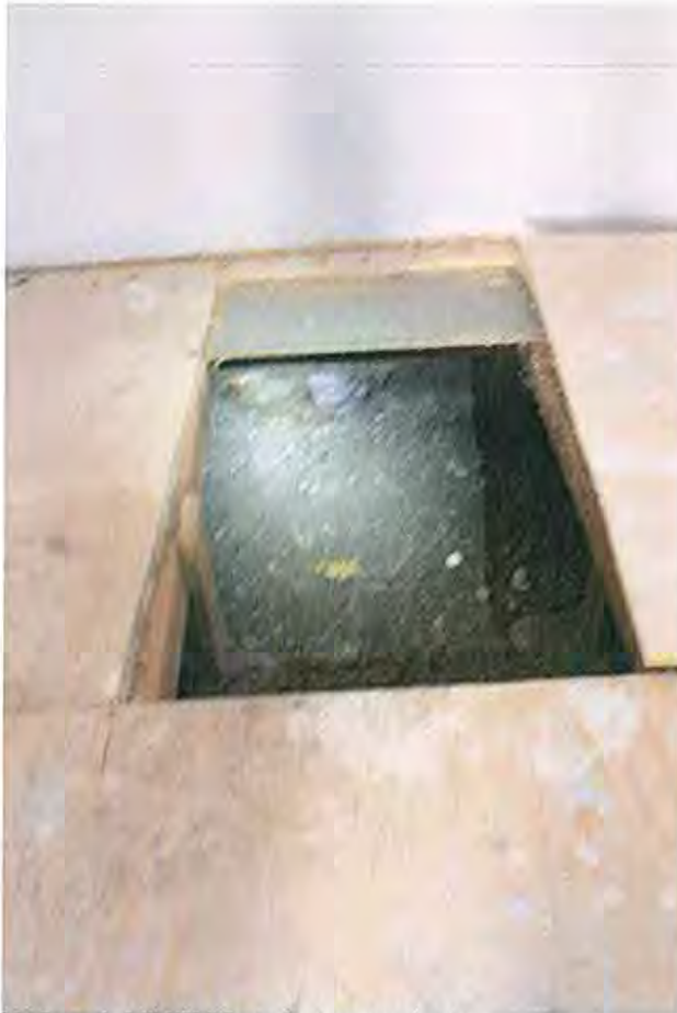
Dirt and rubble foundation-typical
