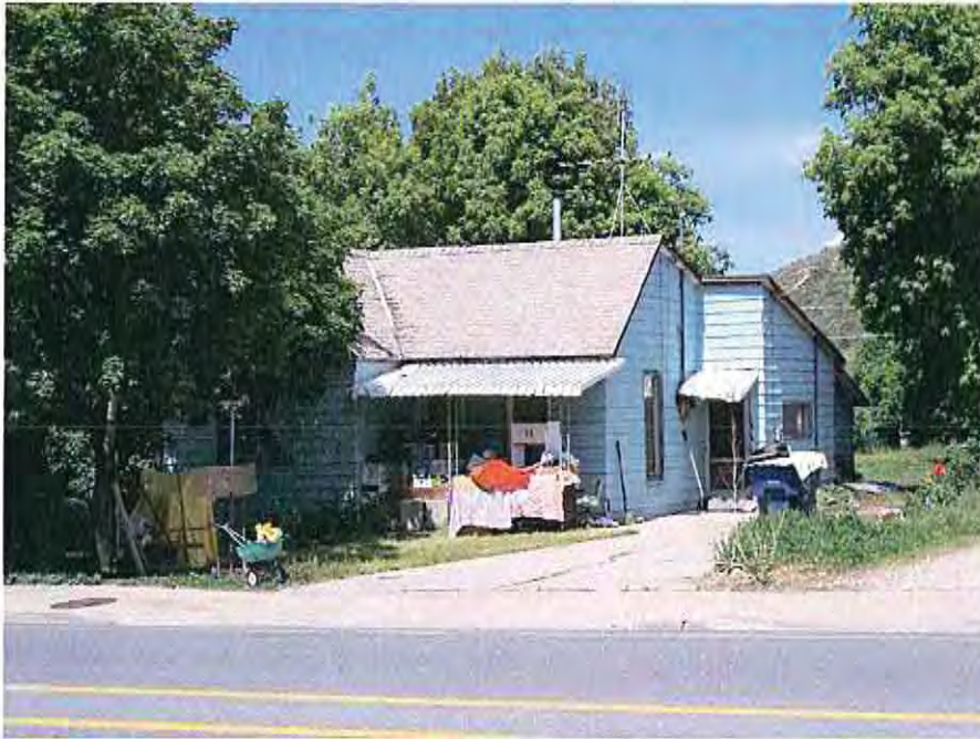
West primary façade 2006 photograph
