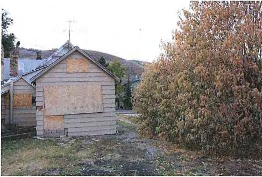
5. Northeast gable-north façade
