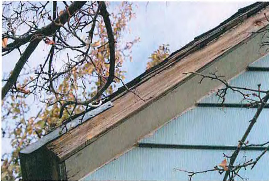
Typical soffit and fascia-functional and simple
