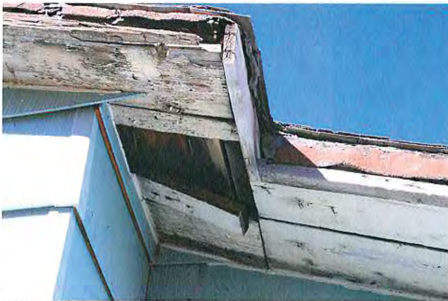
Detail soffit and fascia corner southeast 10"
