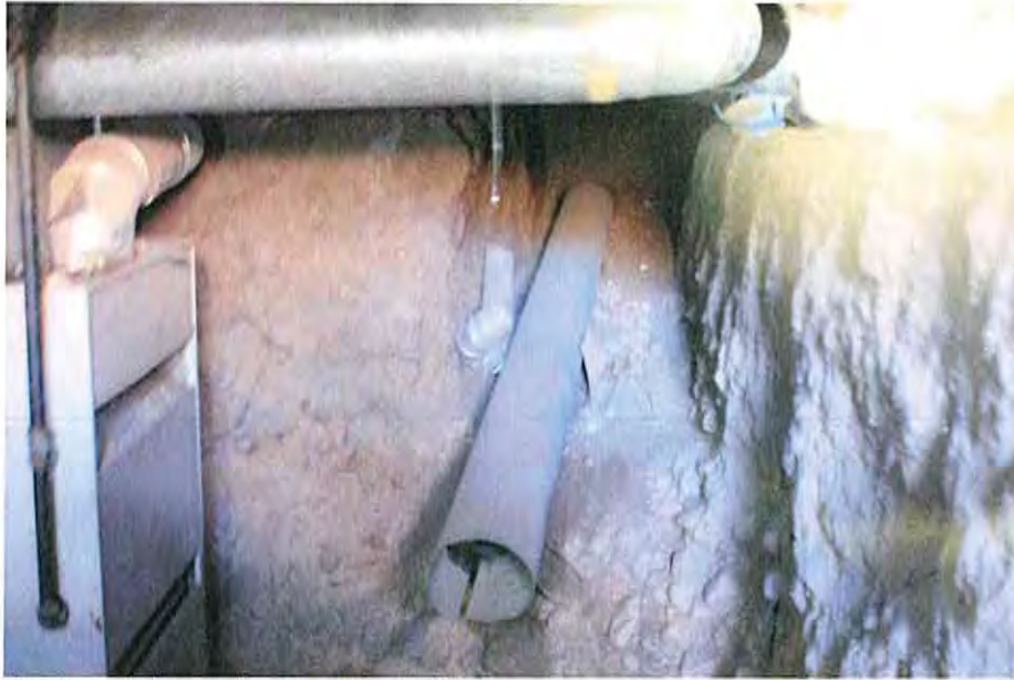
Duct work through excavated dirt
