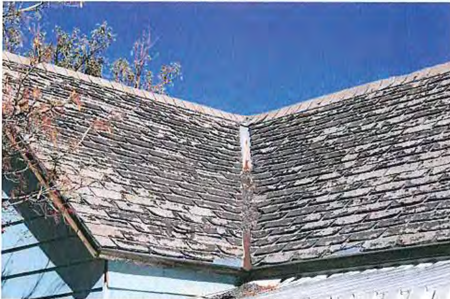
Intersection-valley east-west gable and north-south gable
