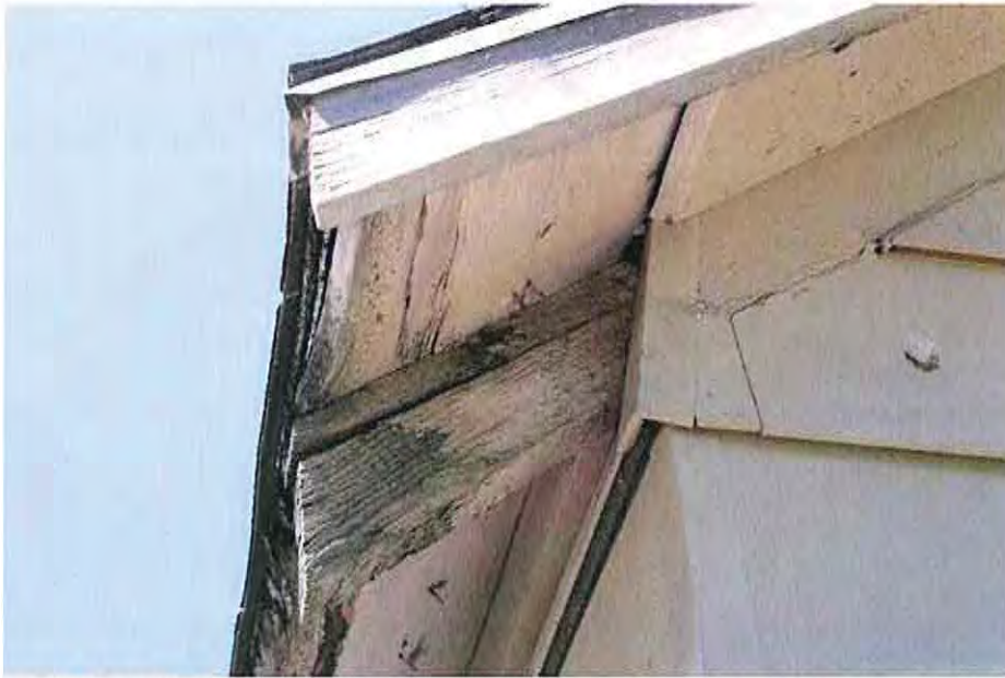
2.Soffit detail northwest corner
