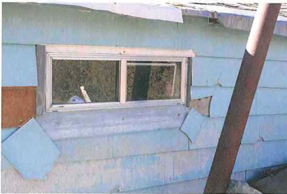
East bathroom aluminum slider 3'-1"W X 12"H and 48" off the ground-patched together casing
