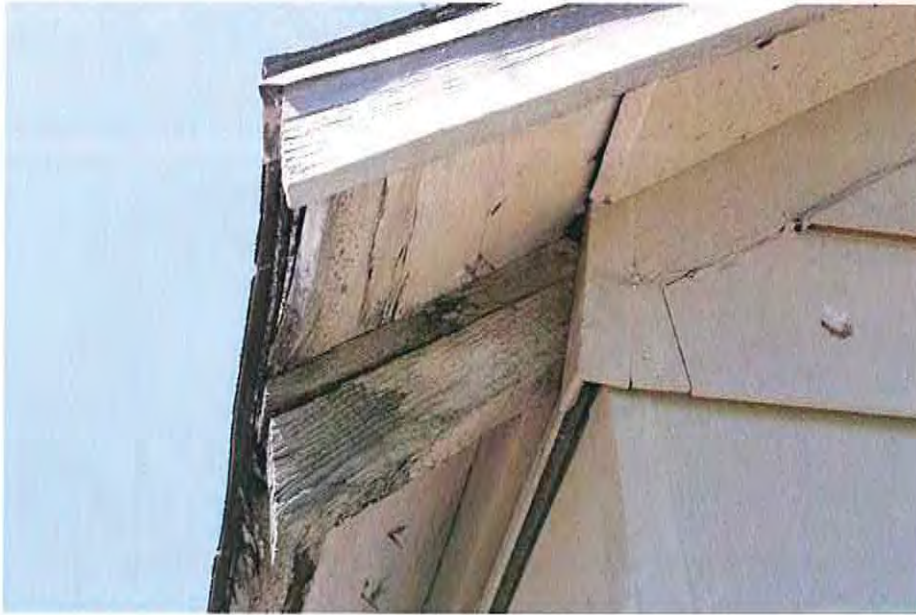
5.Soffit and fascia northwest corner
