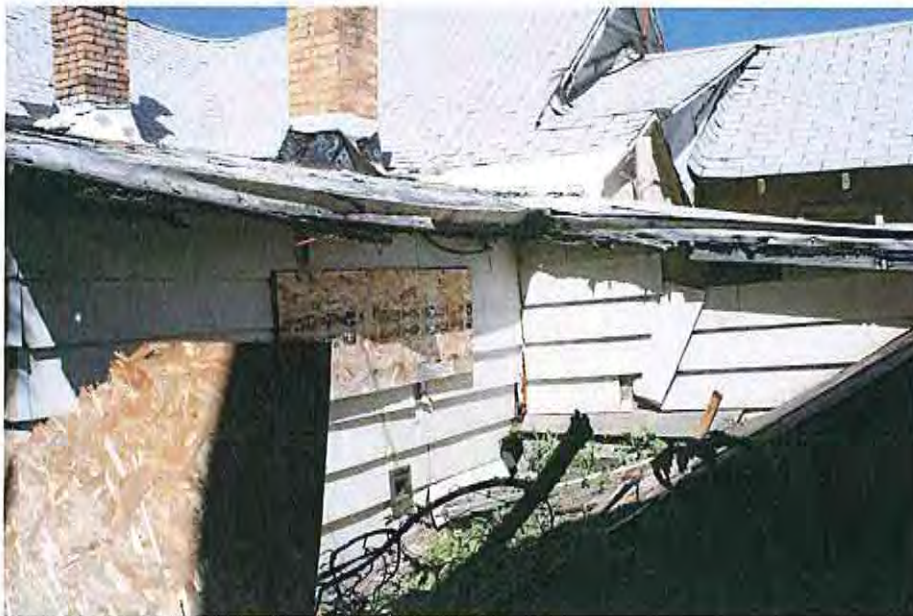
2.East elevation mechanical room shed
