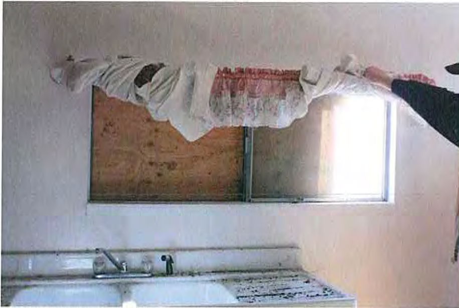
Interior kitchen window casing modified
