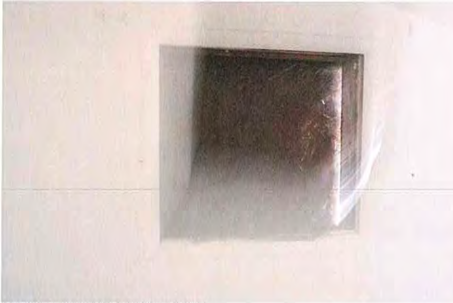
Northeast window-modified frame
