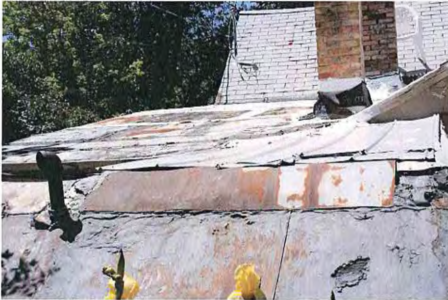
8. East elevation roof condition and chimneys
