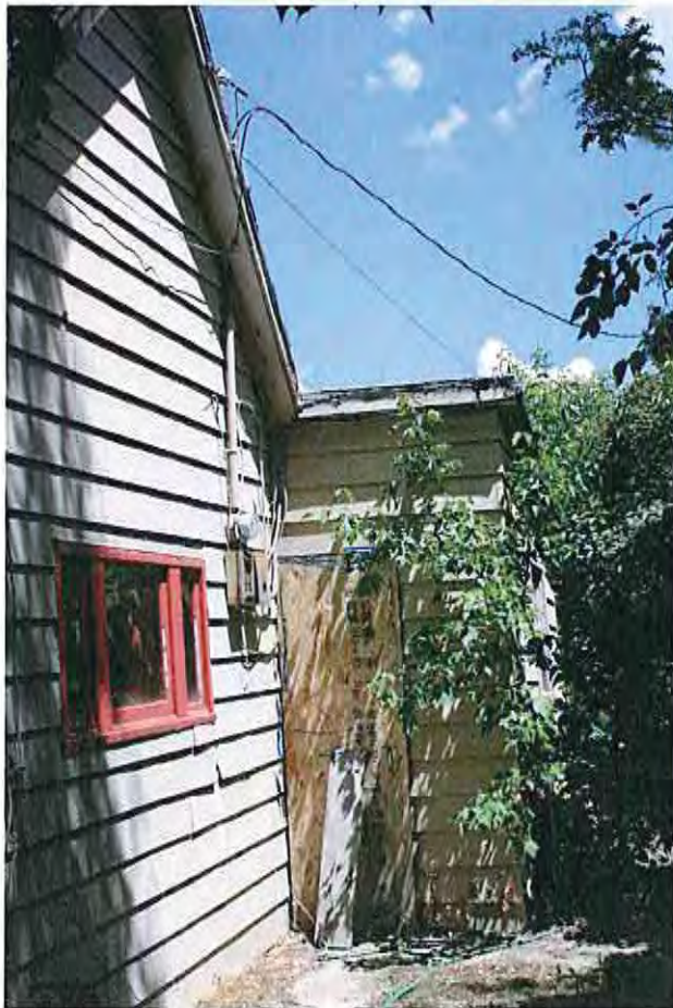
5. West kitchen door
