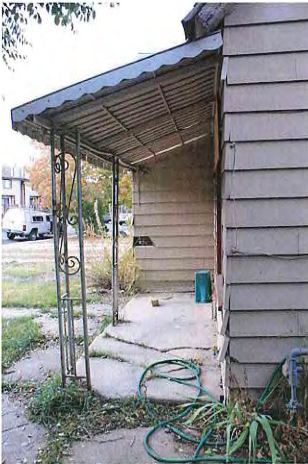
3. Porch- south elevation
