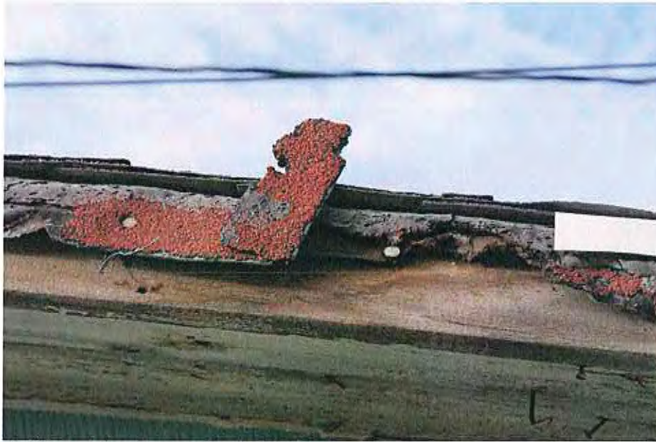
Soffit and fascia south elevation
