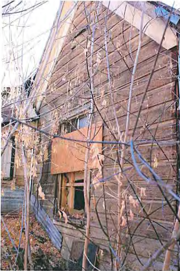
East elevation gable end
