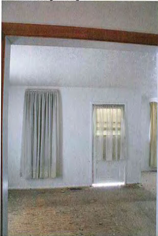
Ceiling lowered throughout house
