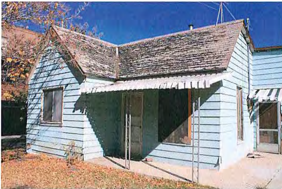
West primary façade- 2010 photograph
