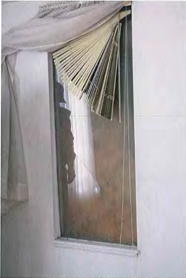
West porch window-2'-7"W X 5'-8"H fixed 24" off porch 2" historic wood casing exterior, interior modified
