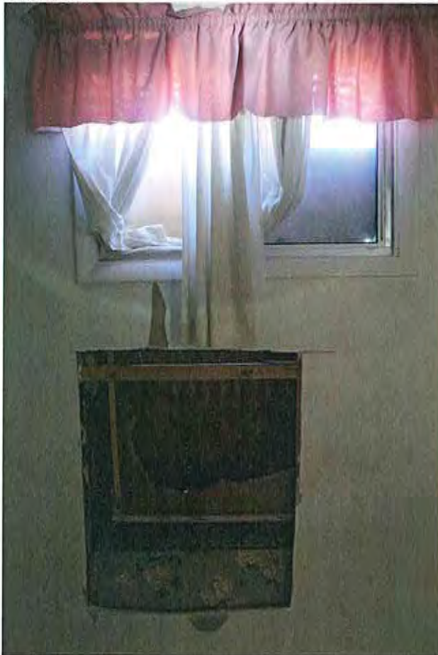
Interior east bedroom window
