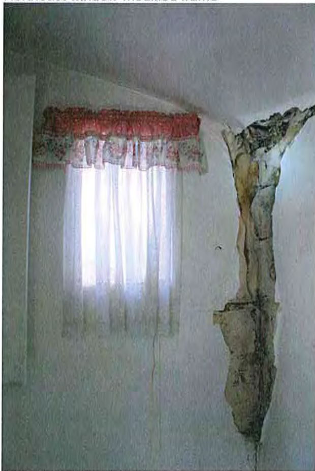
Interior northwest window
