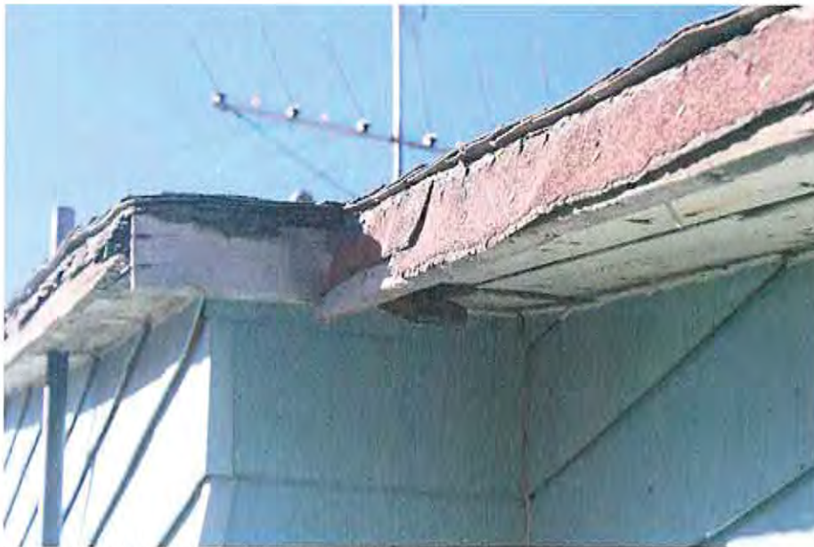
Transition from 6" overhang to 10" overhang
