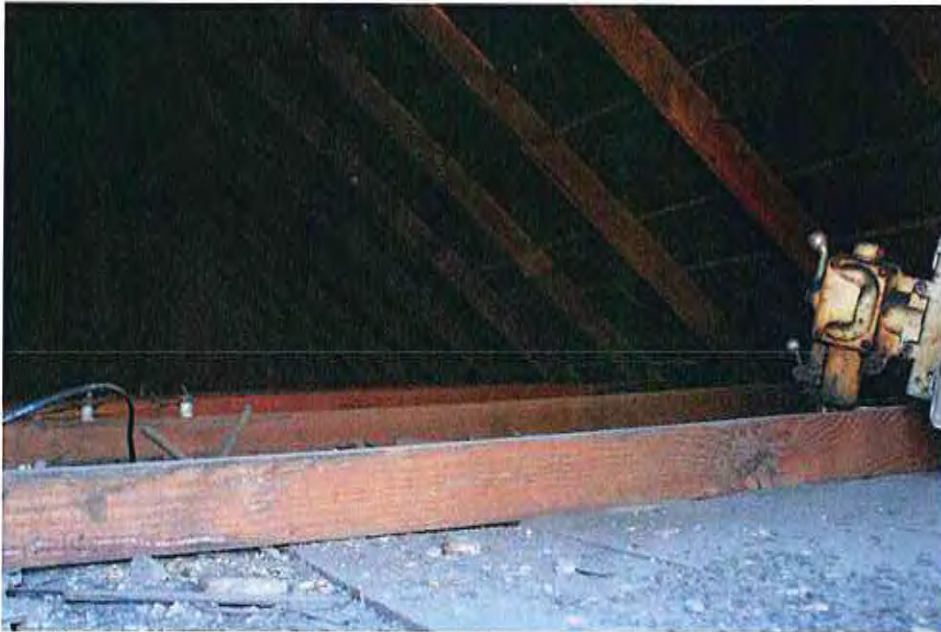
Roof and ceiling framing
