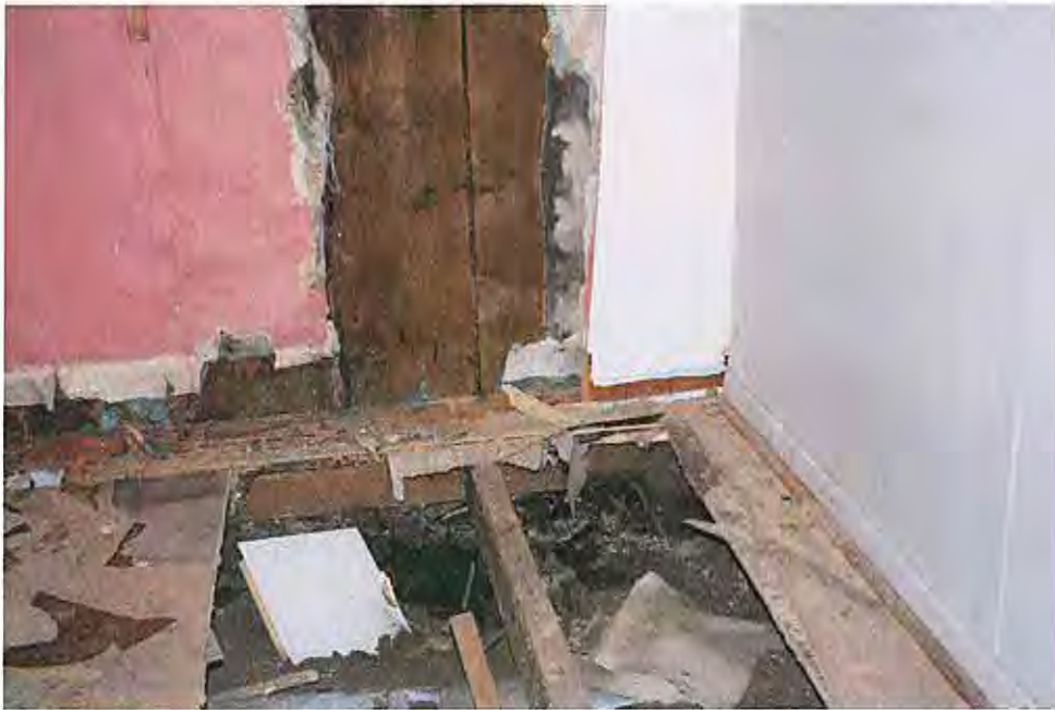
1. 1X12 wall construction. 2 1/8"X6" floor joist.
