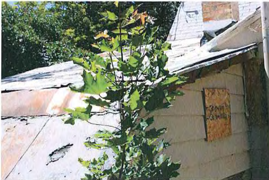
Window at stair to root cellar.
