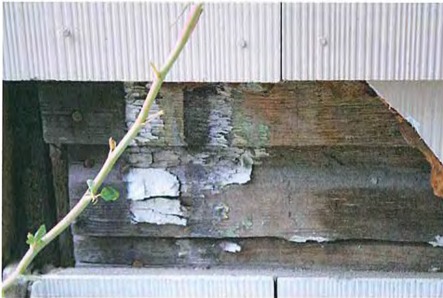
2. Siding detail northwest corner
