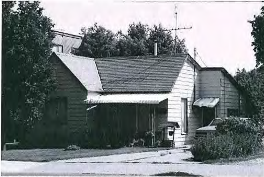
Older photo showing vegetation and concrete areas
