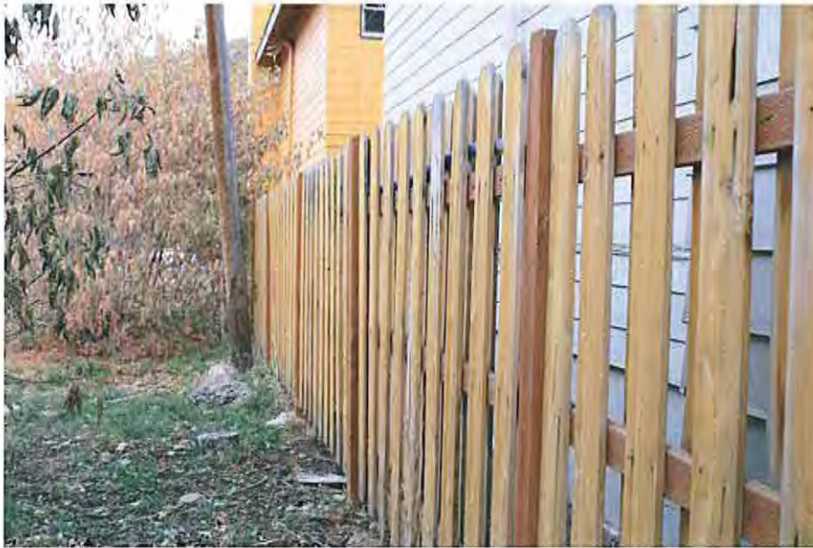
1.South property line wood fence
