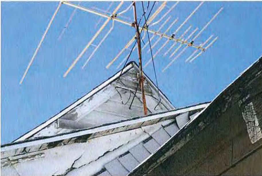
5.East elevation original gable
