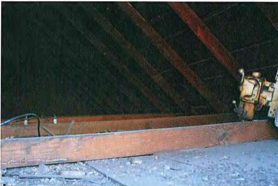
Knob and tube cloth wire-typical
