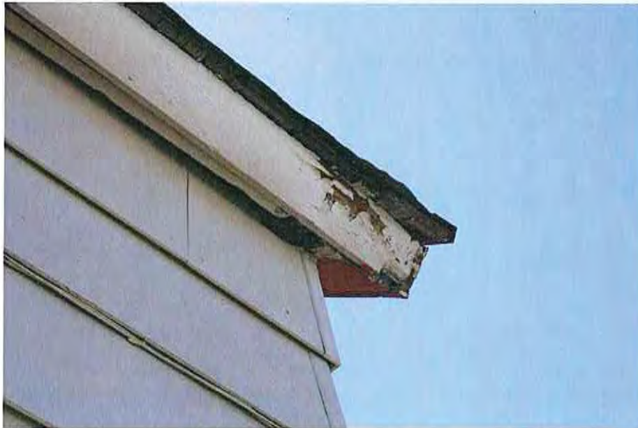
6.Fascia detail northeast corner
