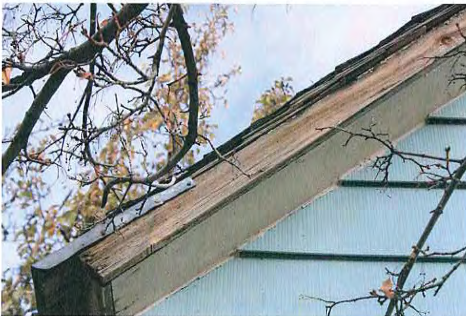
Soffit and fascia at northwest corner.
