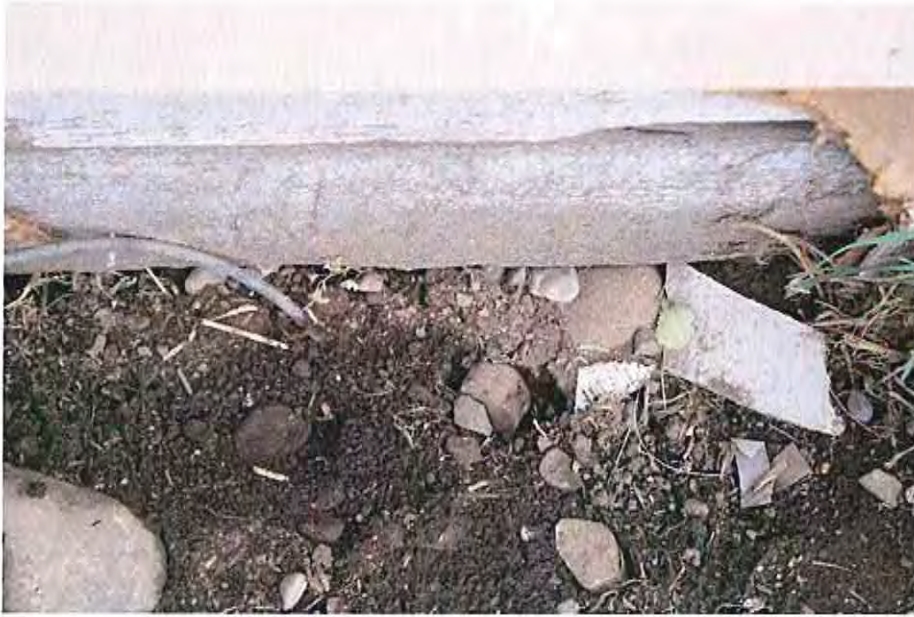
1.Foundation rubble-north elevation
