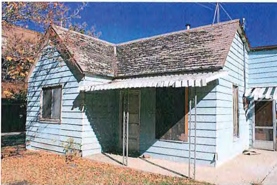
West front porch-2010
