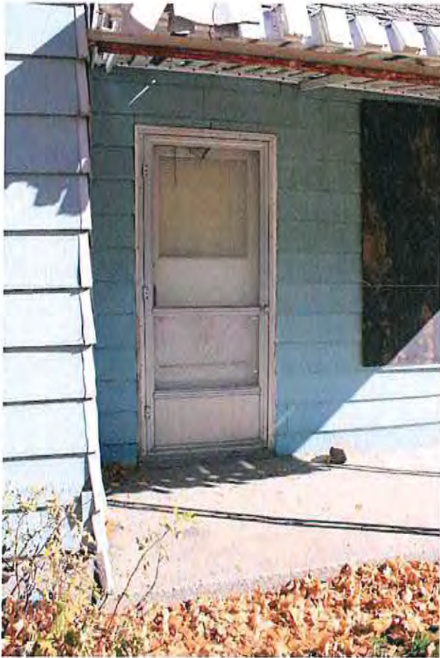
Concrete slab porch floor
