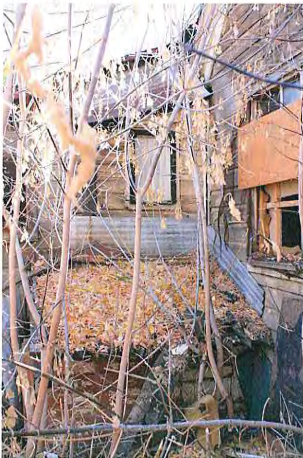
North elevation-shed access to mechanical
