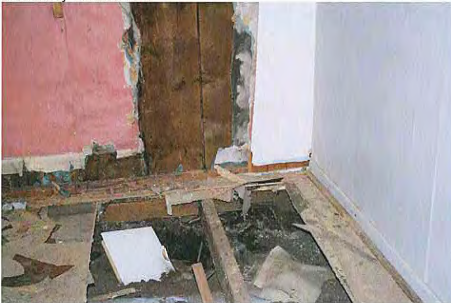
3. Duct work in foreground under floor joist
