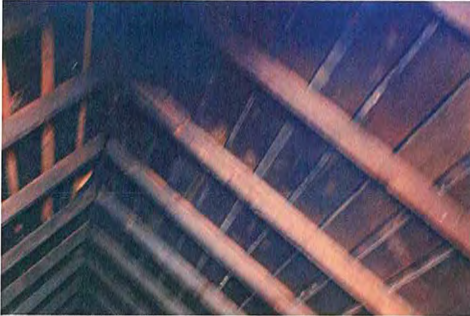
East-west gable framing
