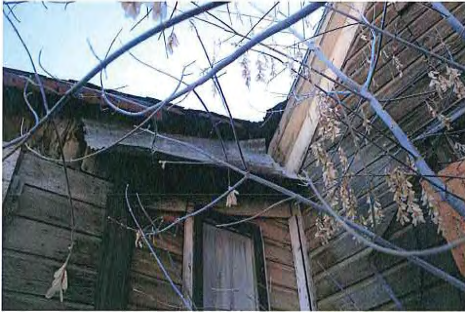
Corner- original 4'-0" shed structure
