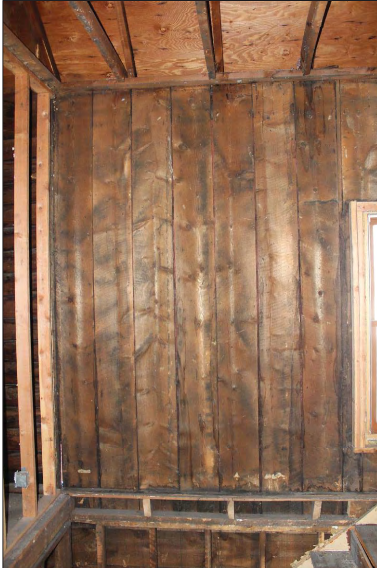
Figure 5. Detail of vertical plank wall construction on the second story, facing northwest. This was likely a wall of the original one-story house that was either raised or dismantled and re-erected to form a second story above the original footprint of the house when major modifications were made in the 1890s. The Type B cut nails present in the plank walls were commonly used through the 1880s. The use of cut nails declined in the 1890s when wire nails became available and these are the nails found on the first story and 1890s rear addition of the house.
