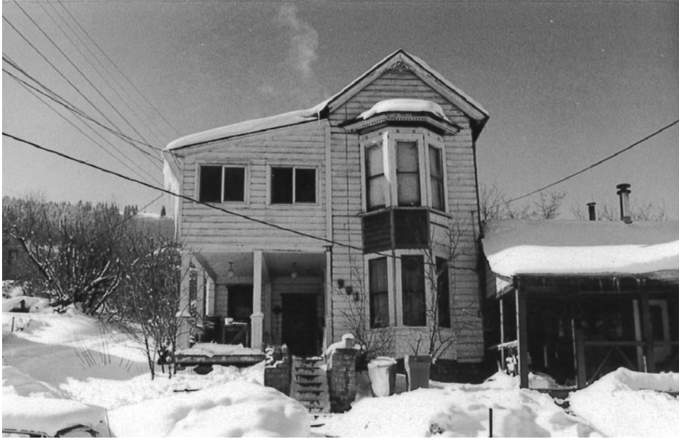
Figure 3 - 901 Woodside Avenue from the 1982 Reconnaissance Level Survey
