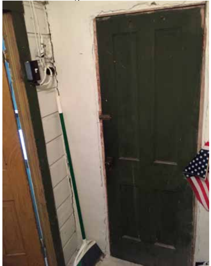
Photo #86: Storage Room
