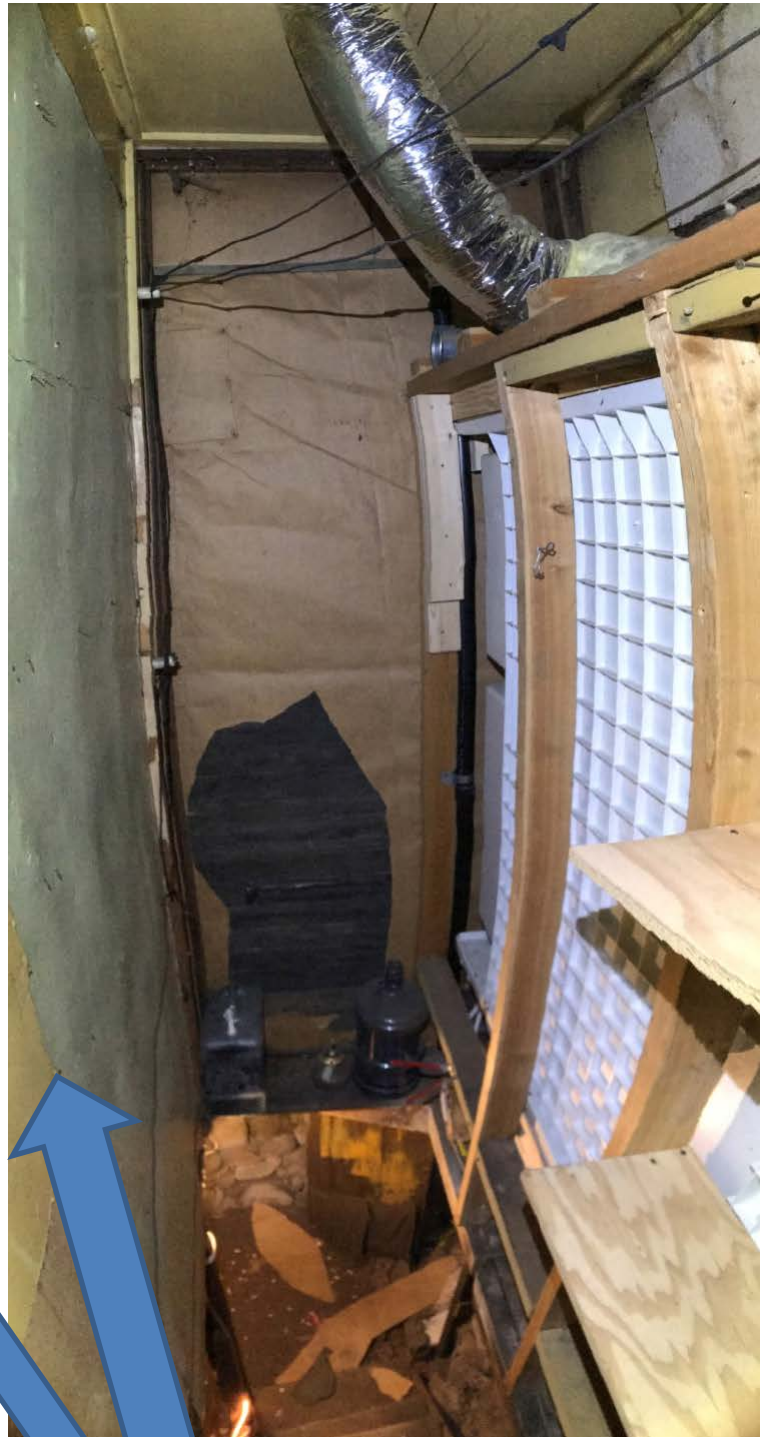
Photograph looking north into enclosed area above cellar staircase.
