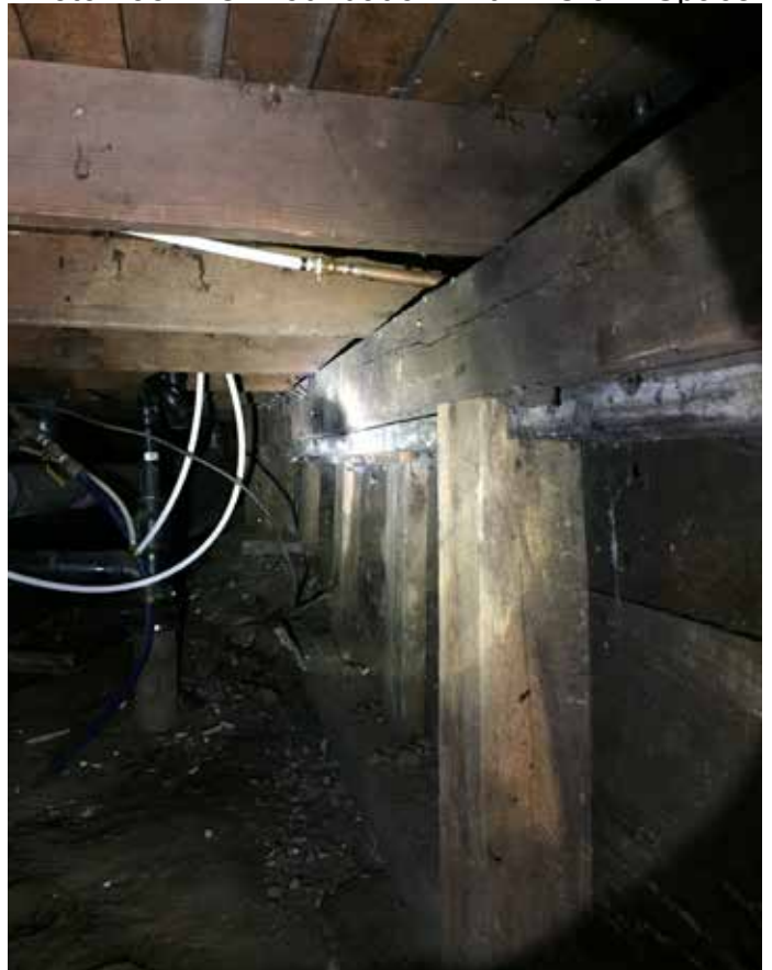
Photo #38: T.O. Foundation Within Crawl Space
