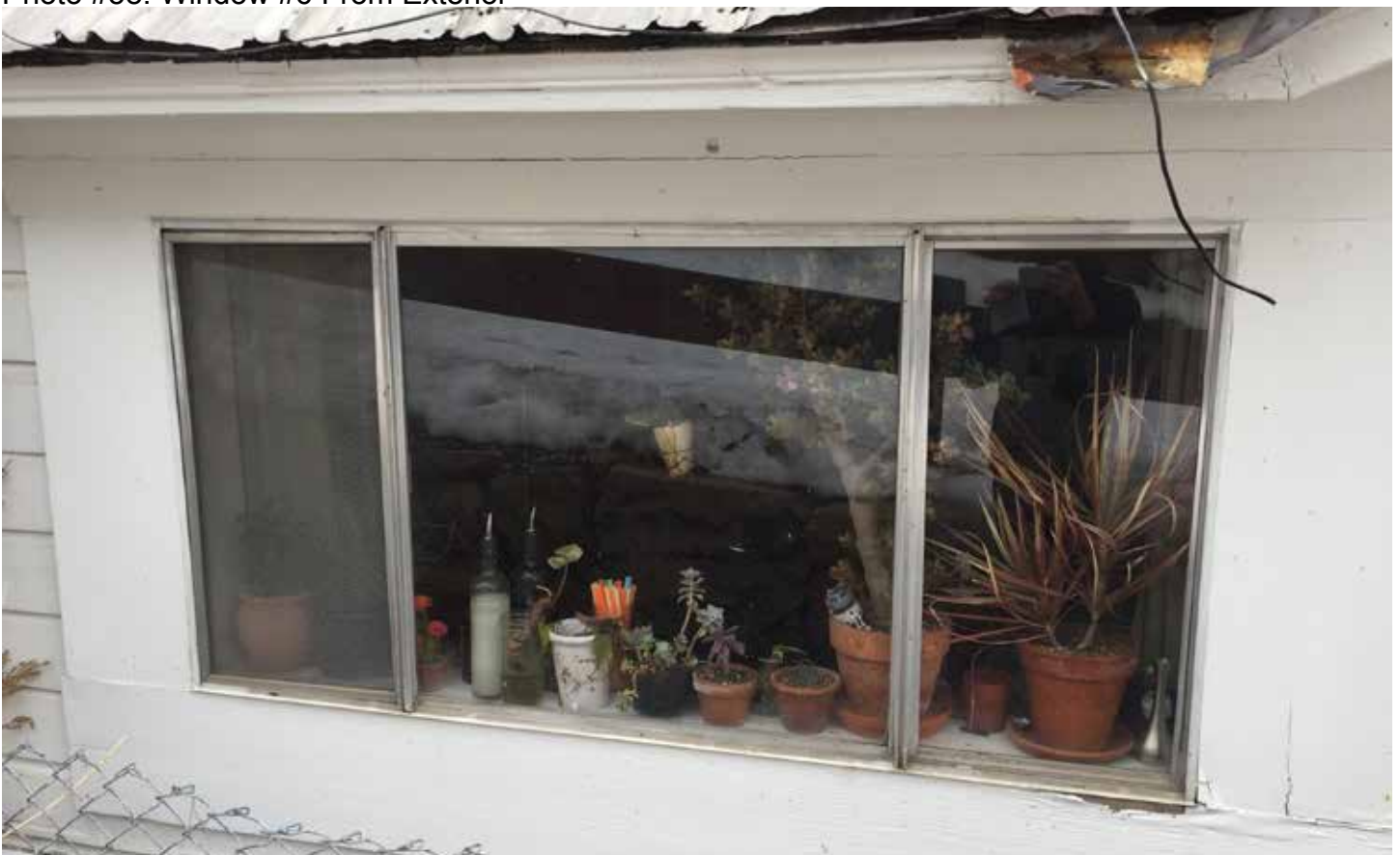
Photo #58: Window #6 From Exterior
