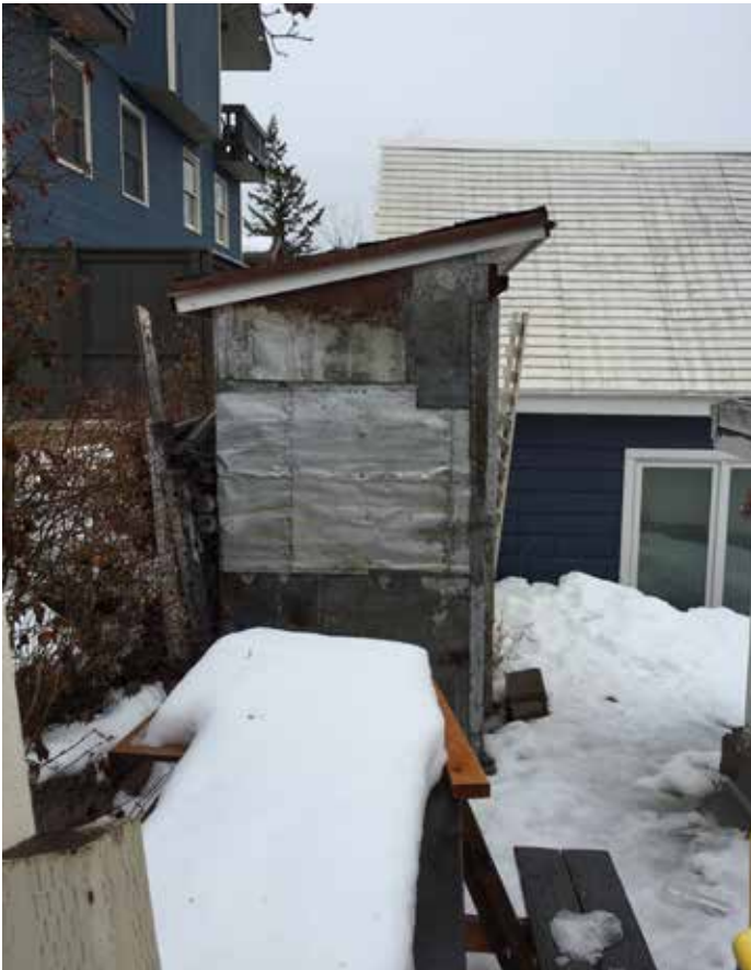
Photo #5: Shed Structure at Northwest Corner
