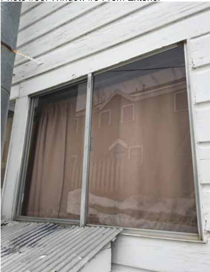
Photo #55: Window #3 From Exterior
