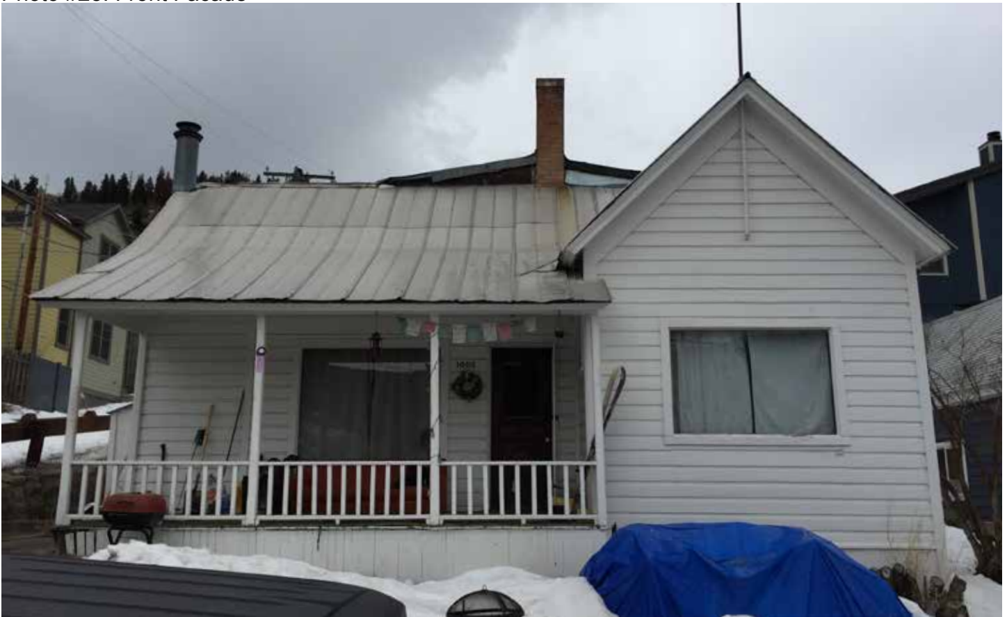
Photo #25: Front Facade
