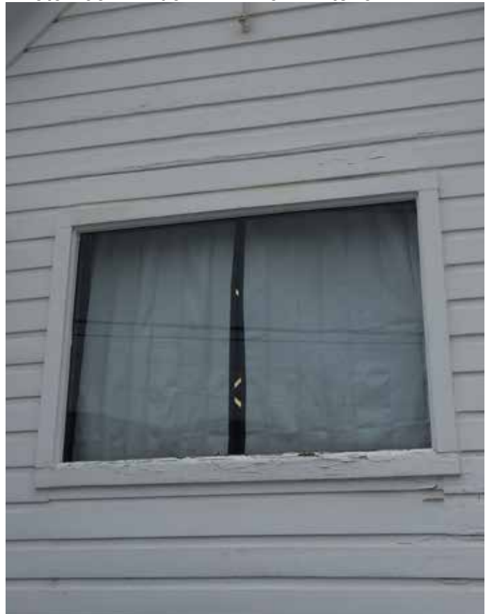
Photo #63: Window #11 From Exterior
