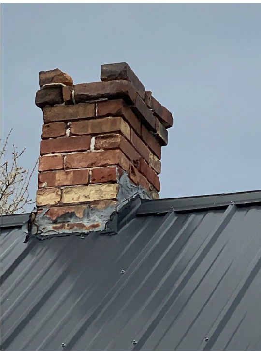
EXISTING BRICK CHIMNEY
