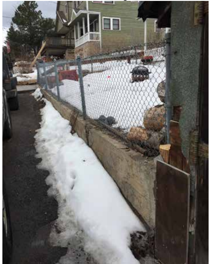
Photo #3: Concrete Retaining Wall & Fence
