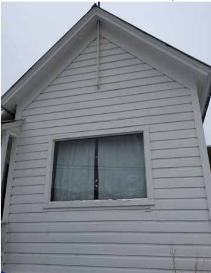
Photo #26: Gable Roofed Wall Close Up
