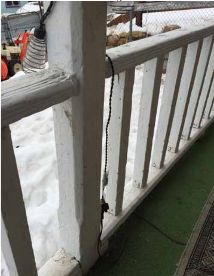
Photo #40: Detail At Railing
