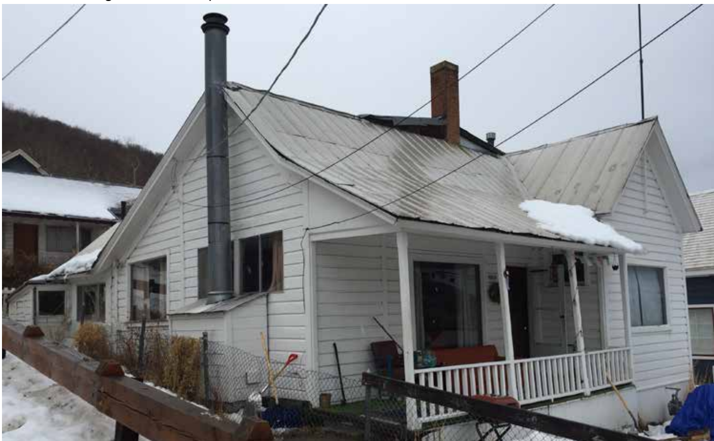
Photo #14: Original Roof Shape From Southeast Corner
