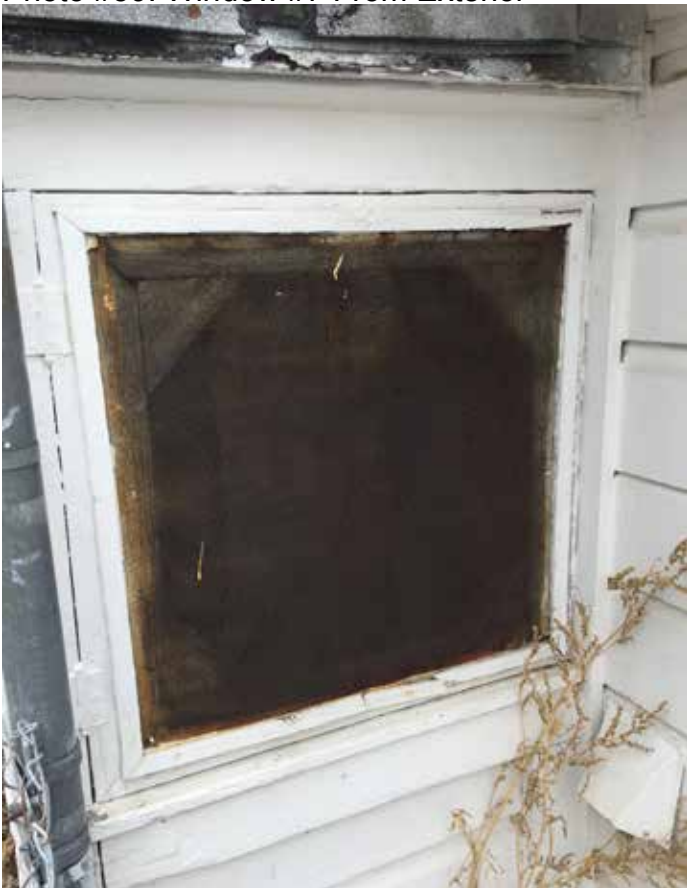
Photo #59: Window #7 From Exterior
