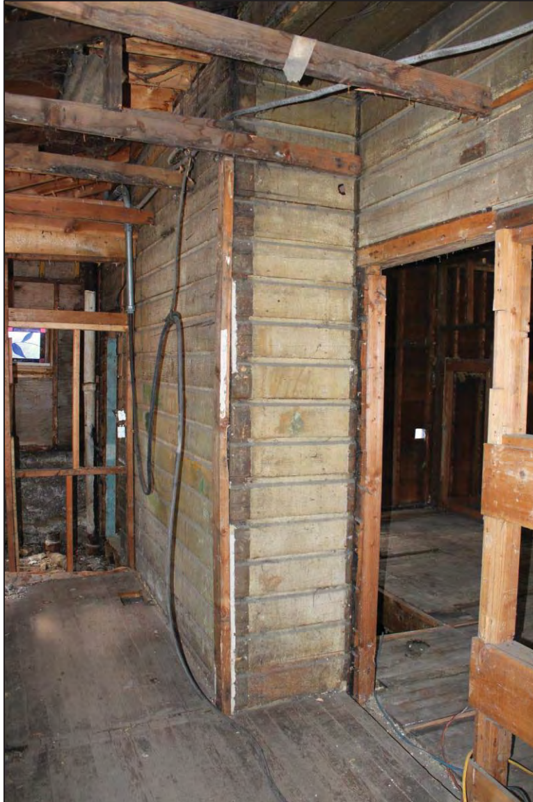
Figure 8. Original drop siding on a former exterior wall at the rear of the house, facing northwest. This wall dates to the 1890s addition and became an interior wall when the rear porch was enclosed by 1941.
