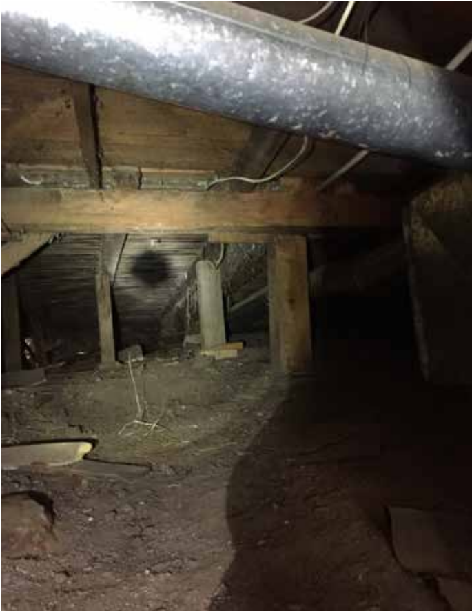
Photo #10: Posts & Beam Supporting Floor
