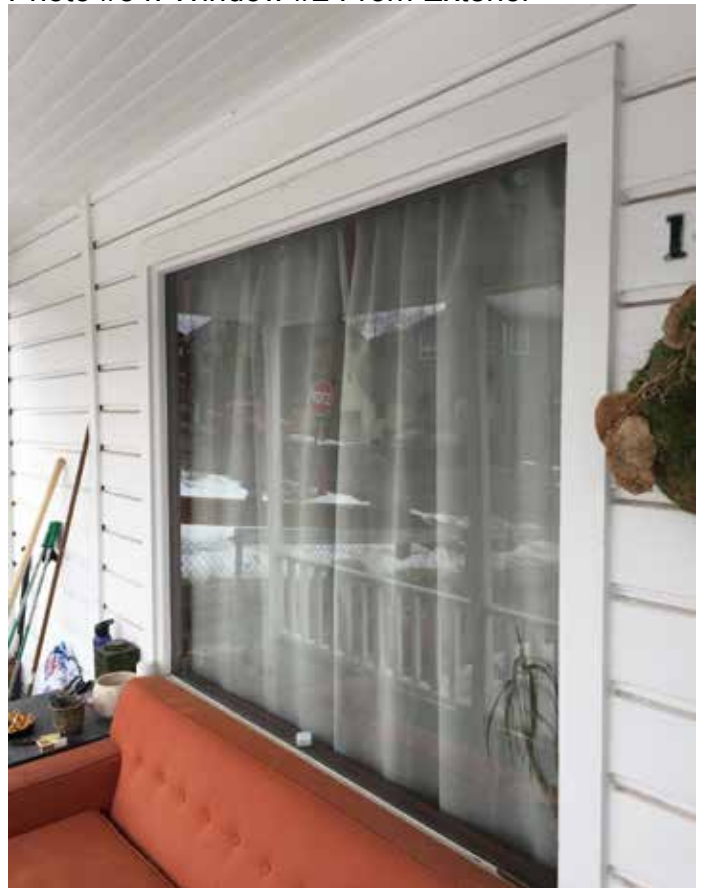
Photo #54: Window #2 From Exterior
