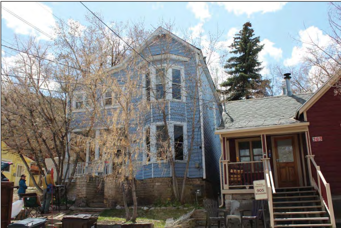
Figure 3. General view of house at 901 Woodside Avenue, facing southwest.
