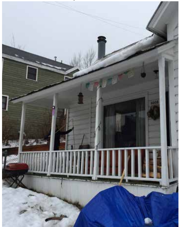
Photo #27: Close Up At Porch
