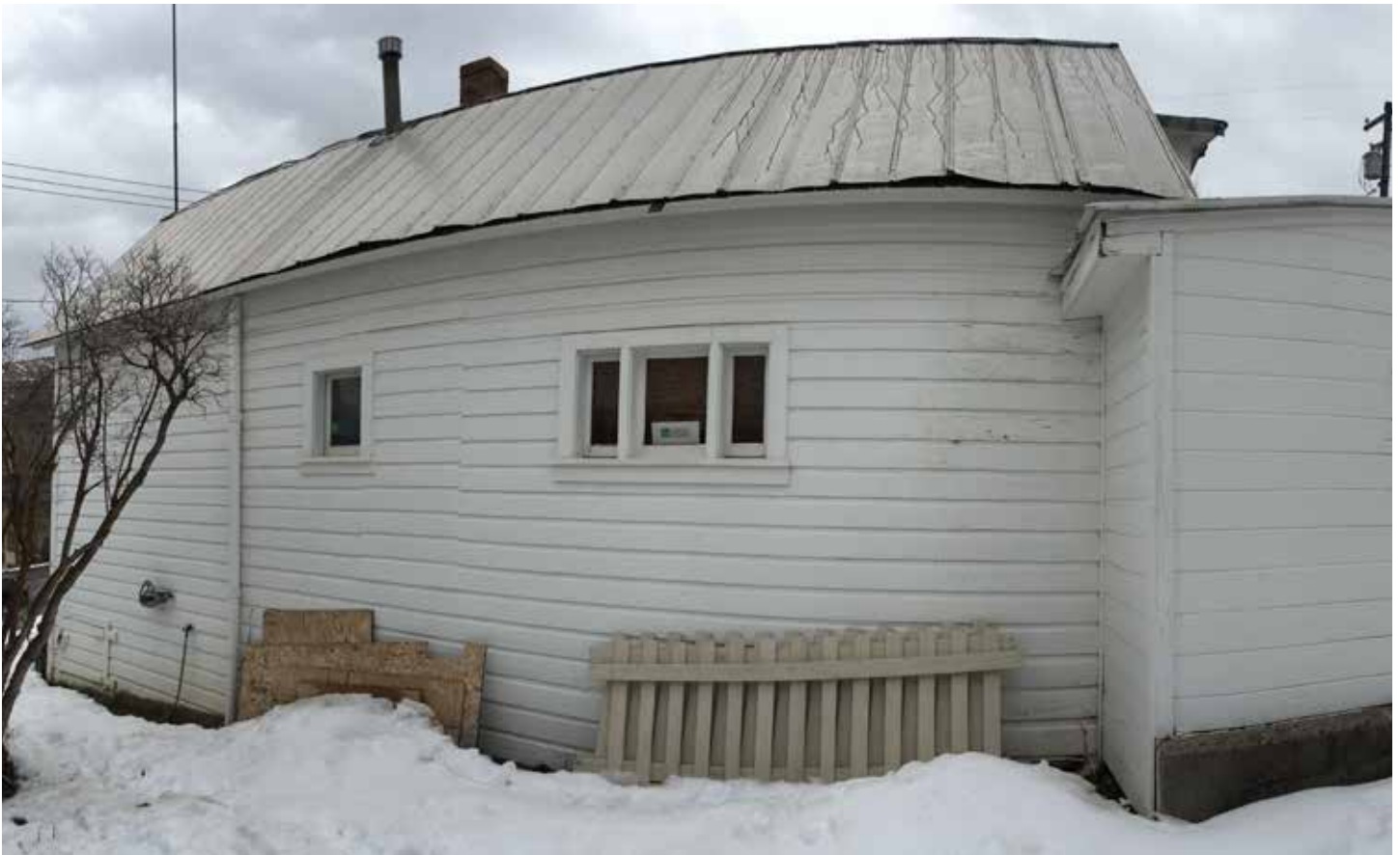
Photo #33: North Facade
