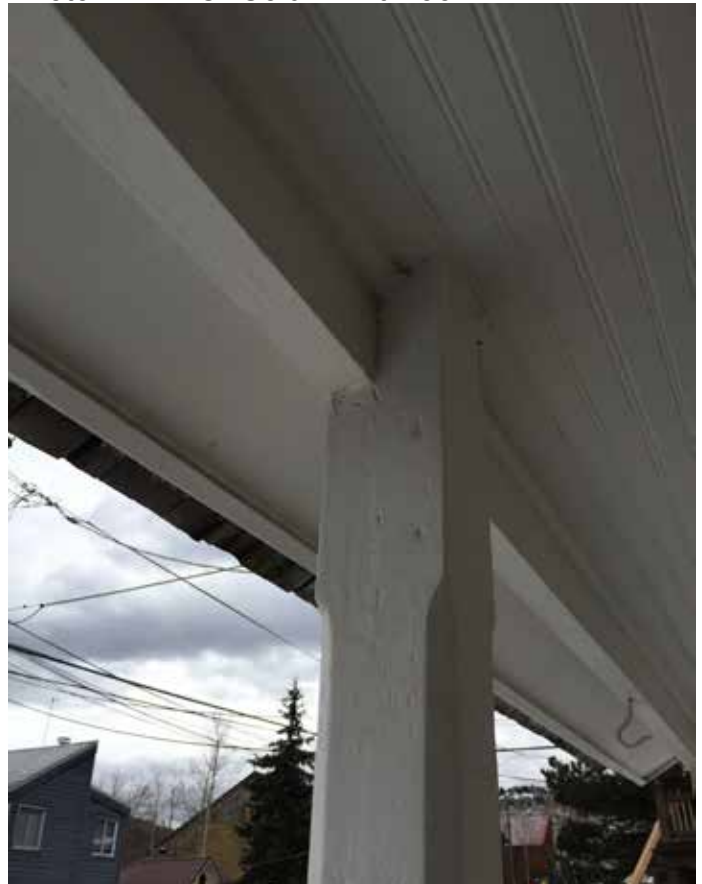
Photo #41: T.O. Column At Roof
