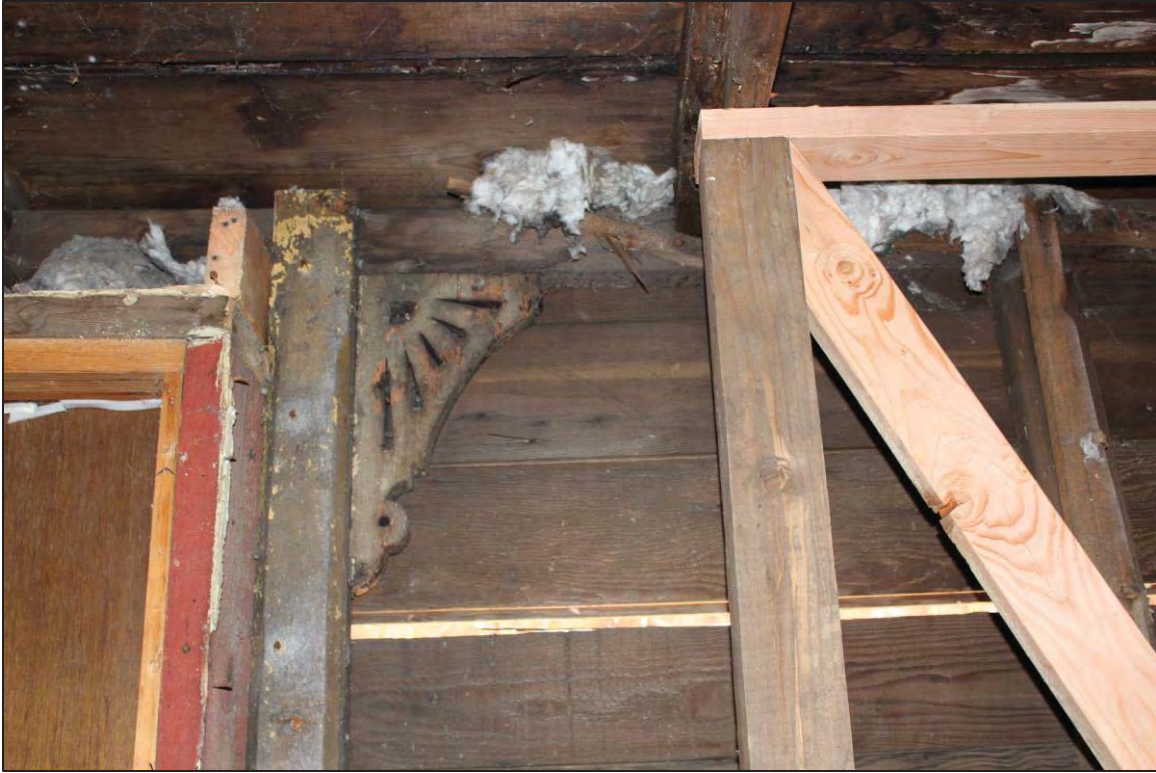
Figure 7. Original rear porch post and bracket, facing southwest. This porch dates to the 1890s rear addition and was enclosed by 1941.
