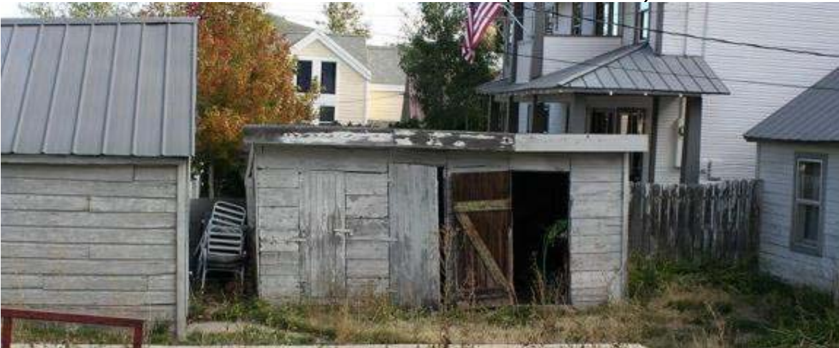
Historic Shed: North Elevation
