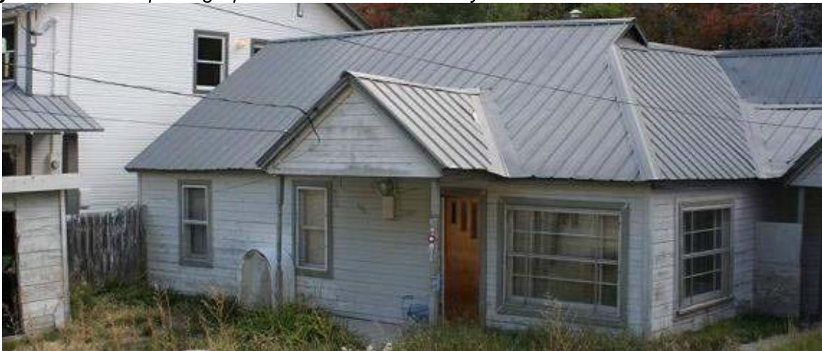
Historic House: West Elevation (northern end)
