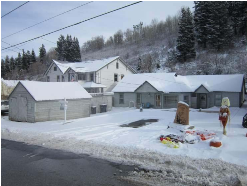
173 Daly Avenue. Southwest oblique. November 2013.
