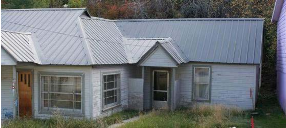
Historic House: West Elevation (southern end)
