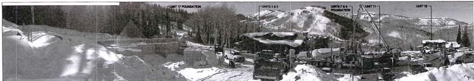
LOOKING SOUTH AT UNIT 17 AND UNITS 7/8
