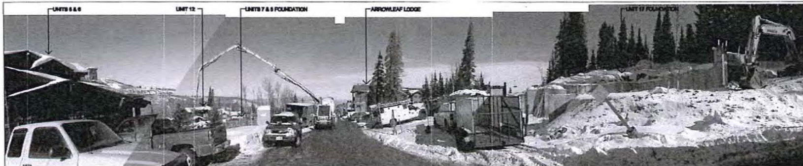
LOOKING NORTH AT UNITS 7/8 AND UNIT 17
