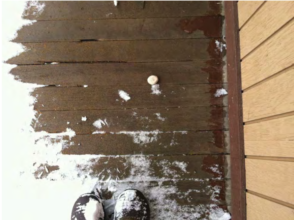
Wood floorboards on porch
