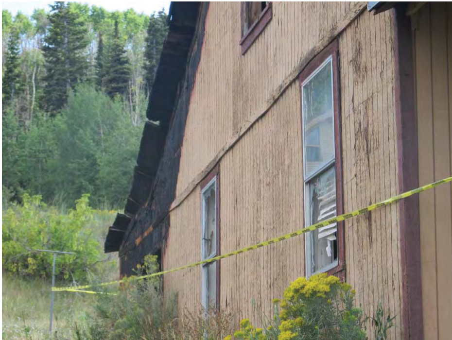
Close-up of East Elevation
