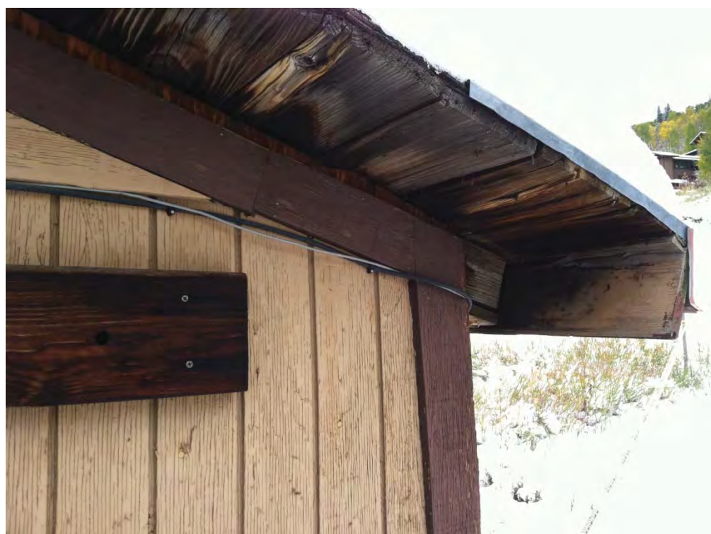
Exposed roof eave, showing old growth timber
