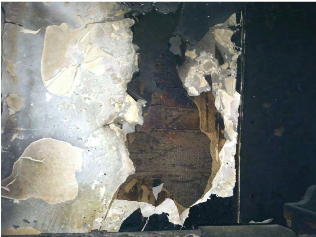
Wall paper applied atop wood wall structure
