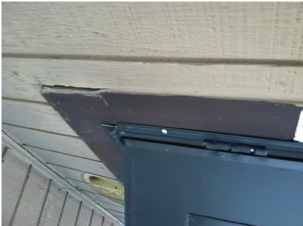
Original wood trim. Note the reveal. Layers of Bricktex and vertical wood siding have hidden much of the reveal on this original trim.
