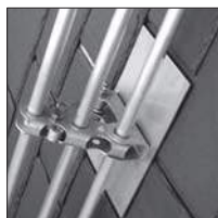
C SNOW RETENTION BARS NO SCALE
