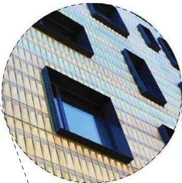
Steel Shrouds on Exterior Windows
