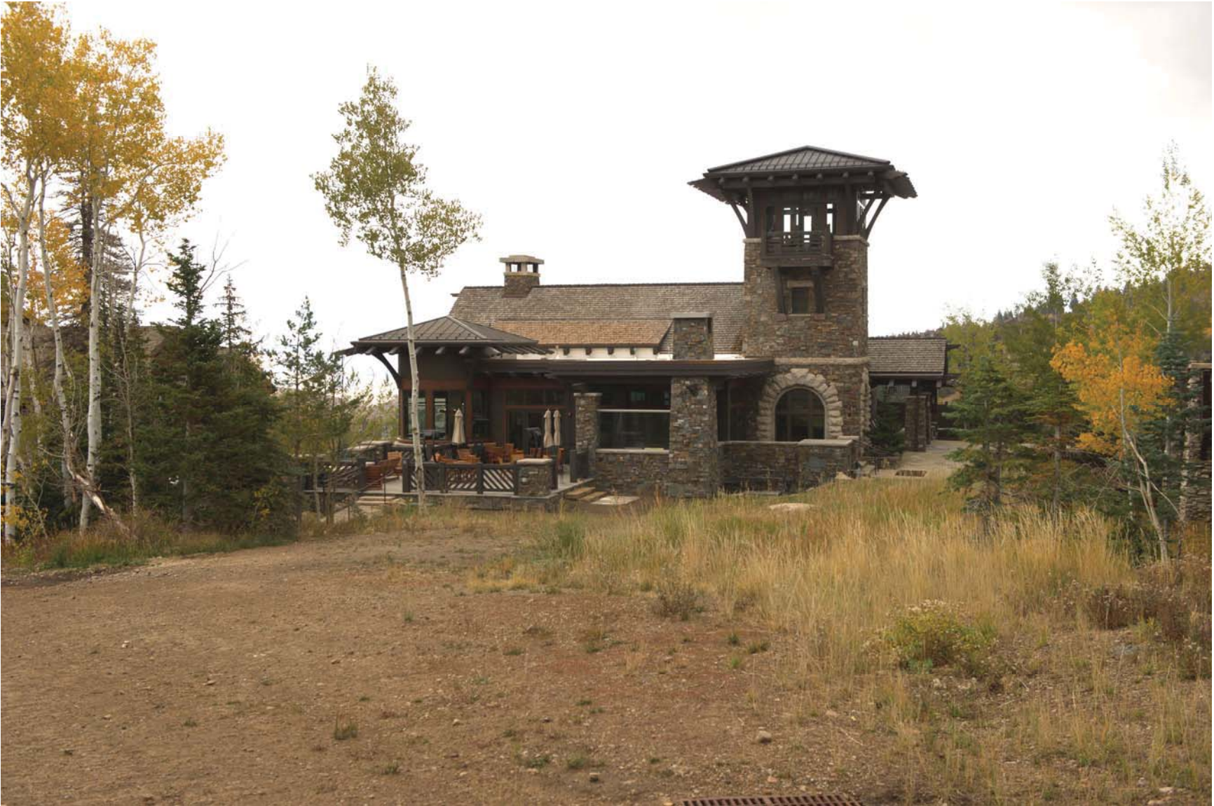
Tower Club – looking Northeasterly
