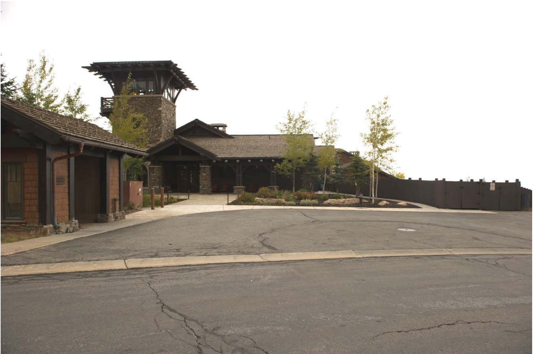
Tower Club – looking Northerly
