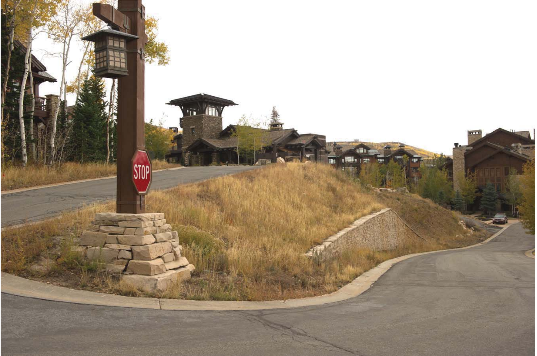
Tower Club – looking Northwesterly
