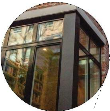
Metal Clad Wood Windows
