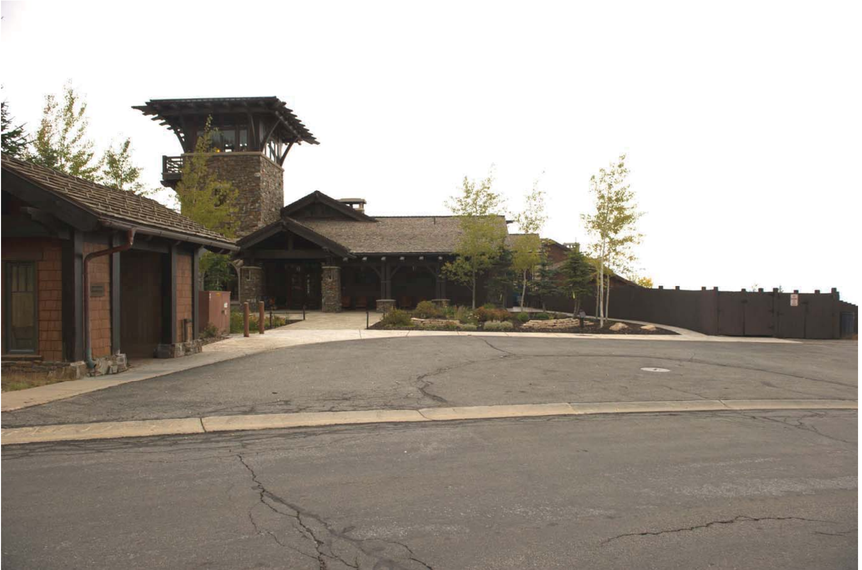
Tower Club – looking Northerly
