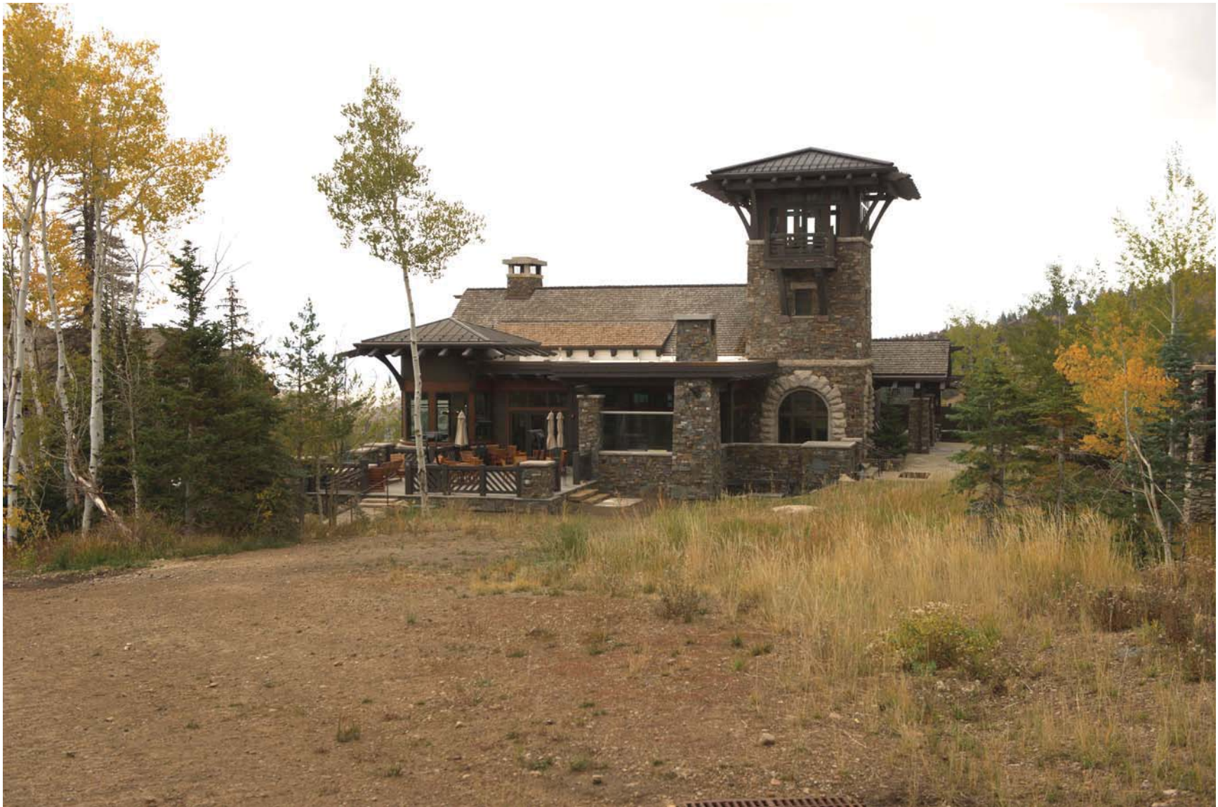
Tower Club – looking Northeasterly
