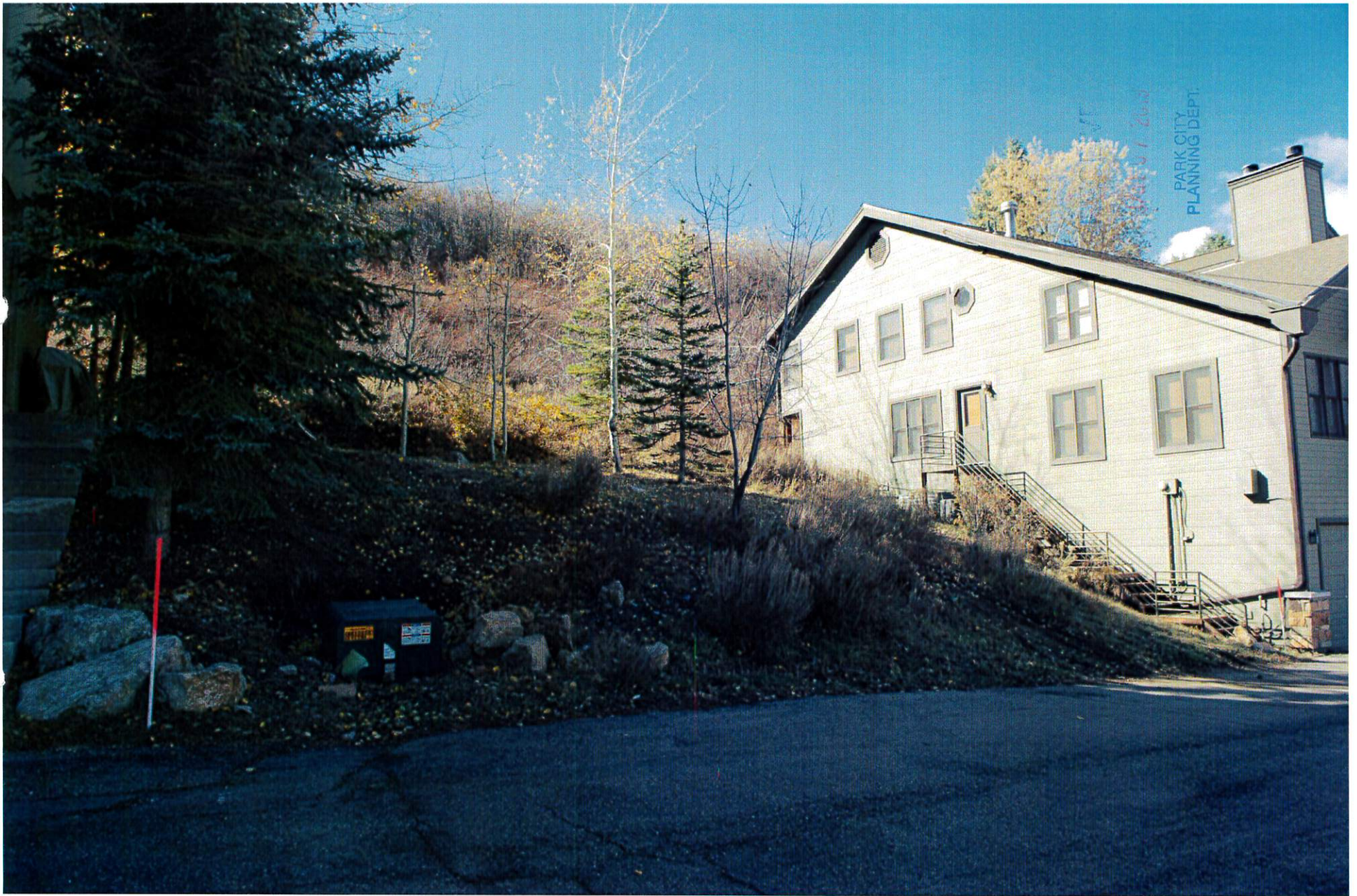
1137 Lowell Avenue - looking westerly from private driveway
