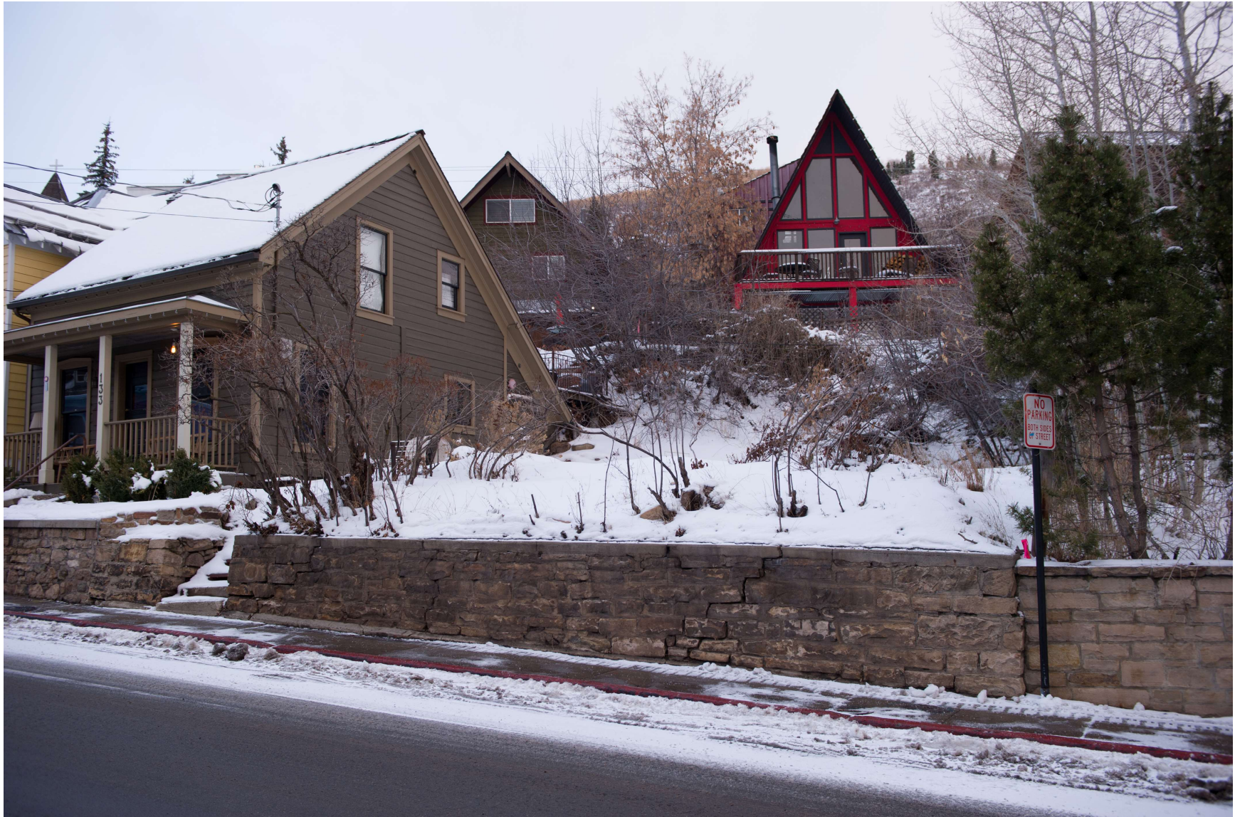
139 Main Street – Looking Westerly
