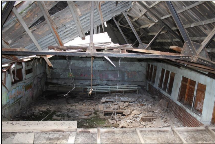
Figure 13. Interior of Judge Mining and Smelting Company Office changing room, facing southwest. Note accumulation of debris on floor and collapsed roof, but with intact metal truss system.
