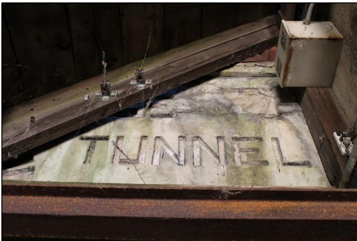
Figure 17. Embossed concrete panel over Anchor (Daly-Judge) Drain Tunnel, facing southwest. Note roof framing partially covering embossed panel, as well as minor cracks and evidence of water infiltration.
