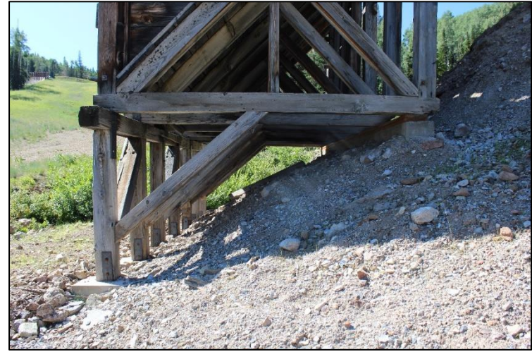
Figure 70. Concrete footings and repaired wood posts supporting Little Bell Mine Ore Bin, facing south.
