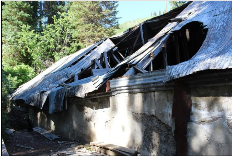
Figure 9. Southeast side of Judge Mining and Smelting Company Office, facing west. Note collapsed roof and spalling concrete of wall.
