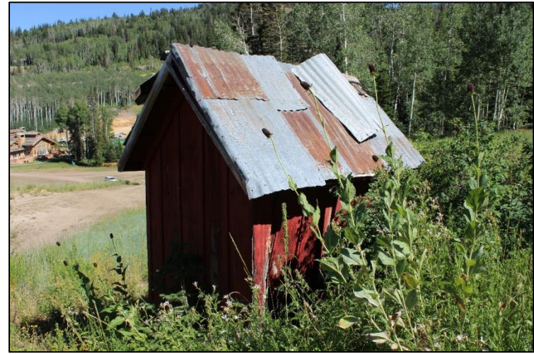
Figure 42. Detached roofing on Daly-West Mine Fire Hydrant Shack No. 2, facing east.
