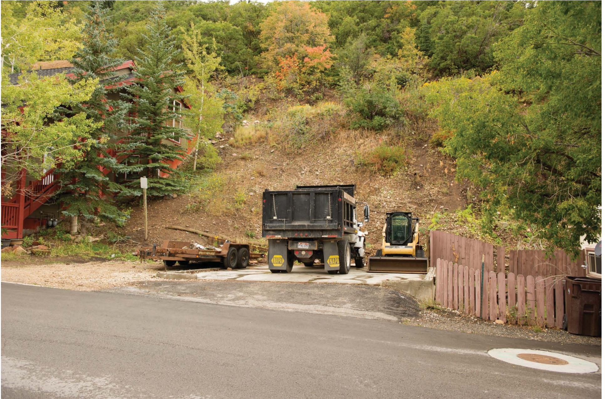
182 & 184 Daly Avenue – looking Southwesterly
