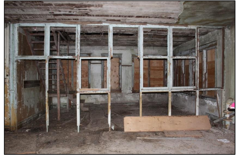
Figure 12. Interior of Judge Mining and Smelting Company Office, first floor, facing northwest. Note the wood partition wall, which may have originally contained windows.
