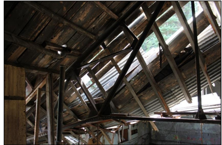
Figure 14. Interior of Judge Mining and Smelting Company Office changing room. Detail of collapsed roof with intact metal truss system, facing south.
