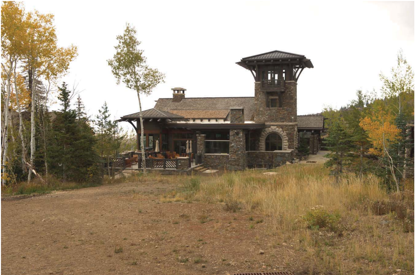
Tower Club – looking Northeasterly
