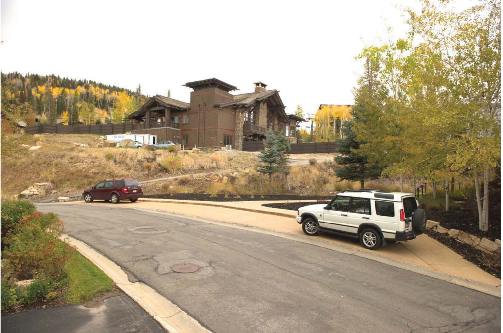
Tower Club – looking Southwesterly
