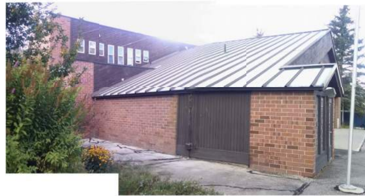
4. View From North Elevation
