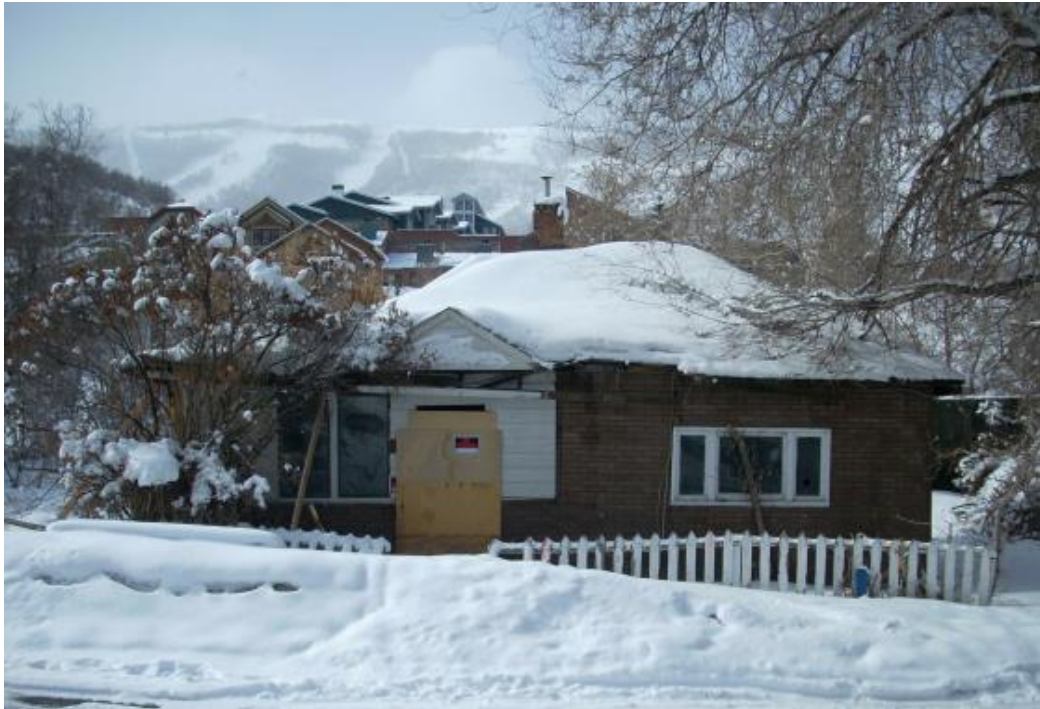
Figure 4: Photograph prior to removal ca. 2009.
