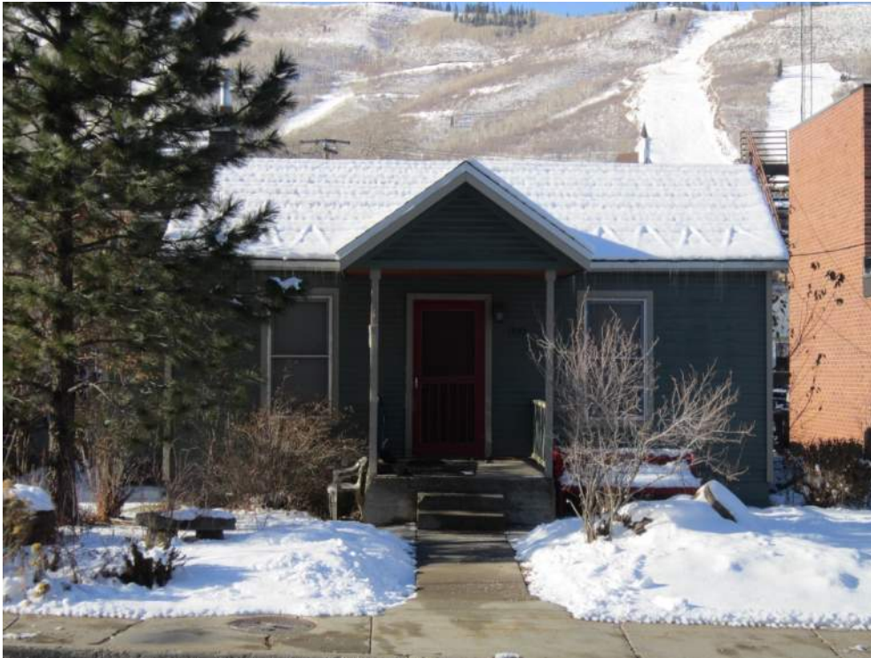
1333 Park Avenue. East elevation. November 2013.
