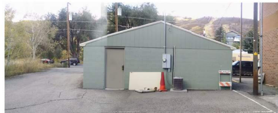
6. View From West Elevation
