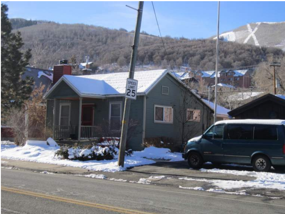
1333 Park Avenue. Northeast oblique. November 2013.
