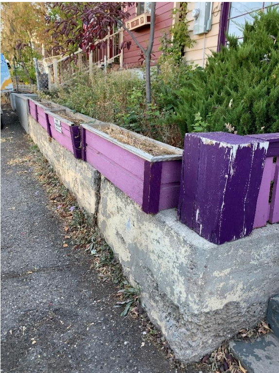
Photo 70: Concrete retaining wall
