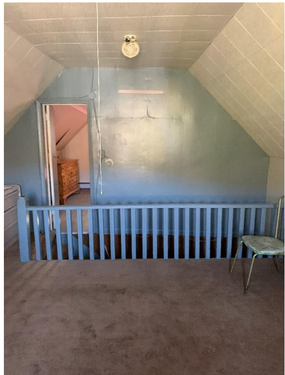
Photo 40: Stairs and railing
