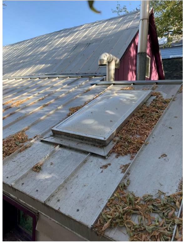
Photo 59: North elevation sky light
