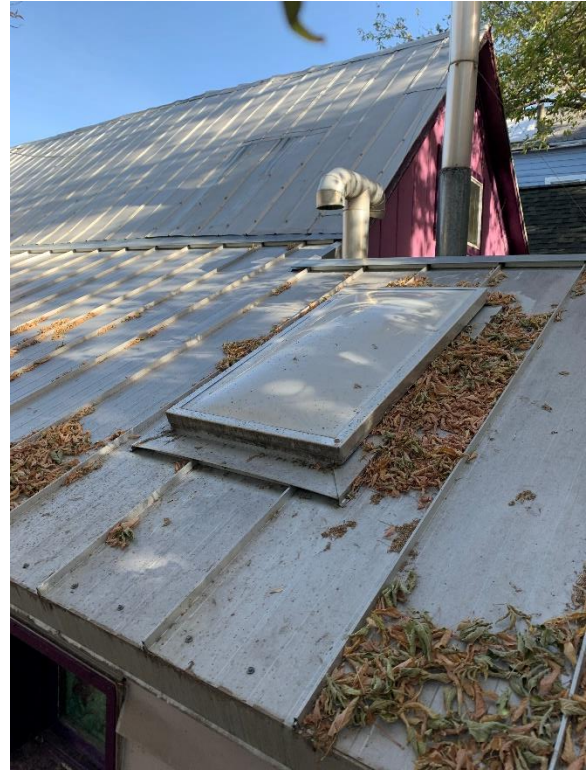
Photo 59: North elevation sky light
