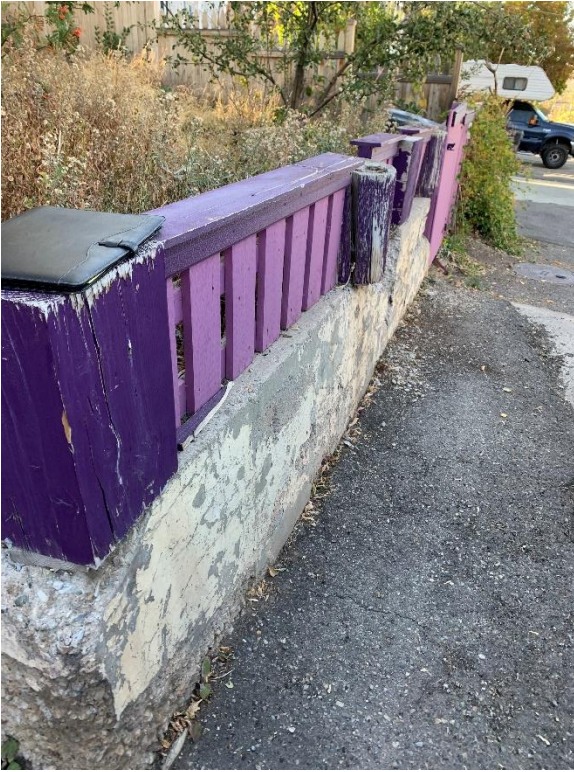
Photo 69: Concrete retaining wall
