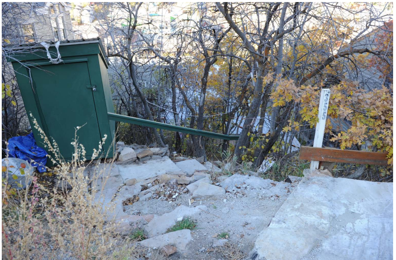
355 Ontario Avenue looking west
