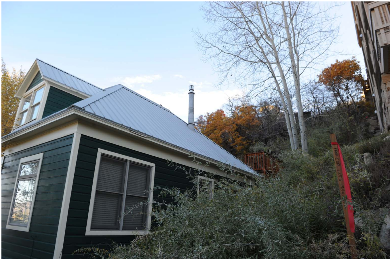
355 Ontario Avenue looking east
