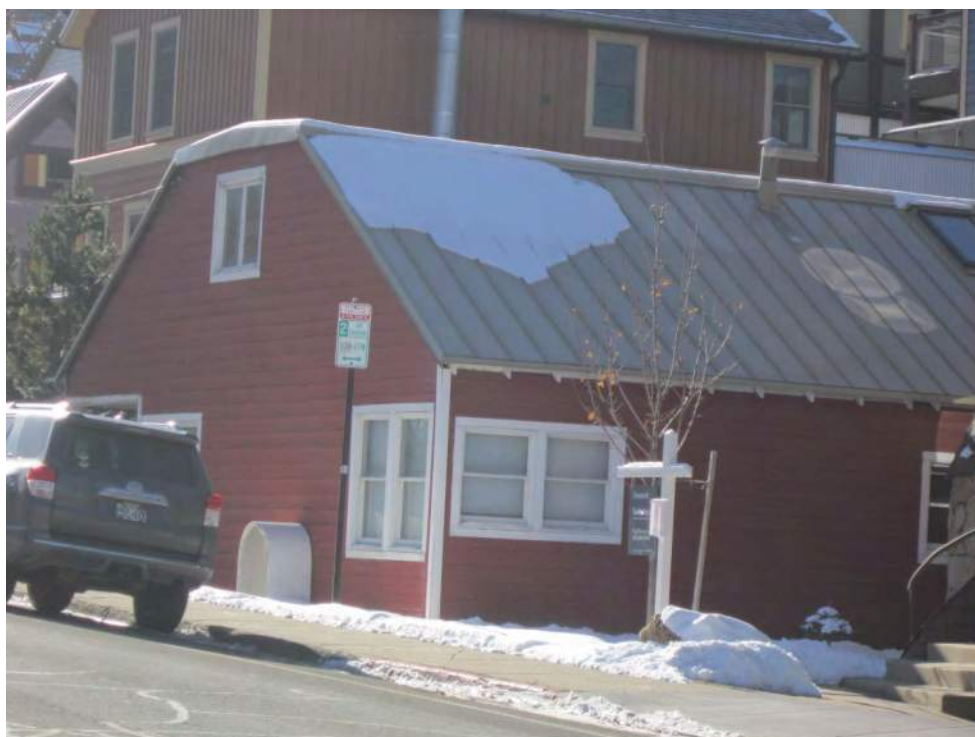
819 Park Avenue. Northeast oblique. November 2013.
