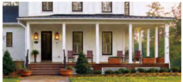
Porch raised above finished grade
