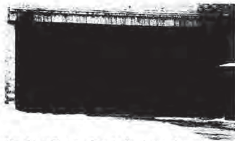
Not this - Garage door is dominant element
