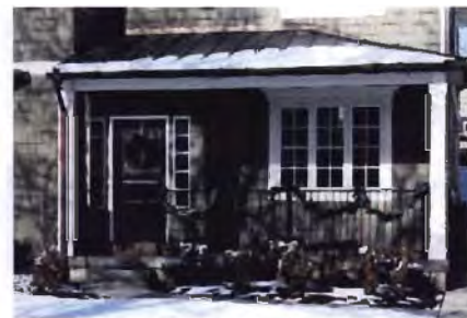
Porches are elevated 18" 8" above finished grade
