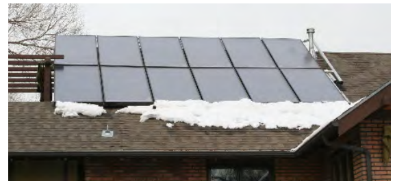
Solar panels visual impacts are minimized
