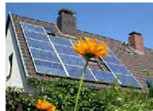
Solar panels visual impacts are minimized
