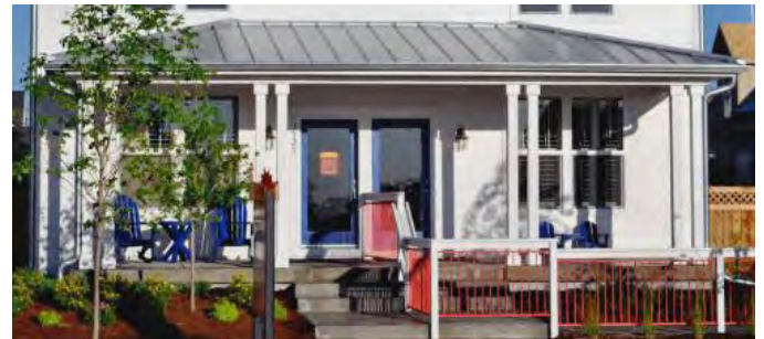
Properly detailed porch elements
