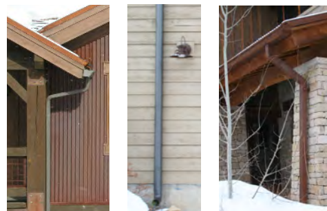
Gutters must complement the homes style
