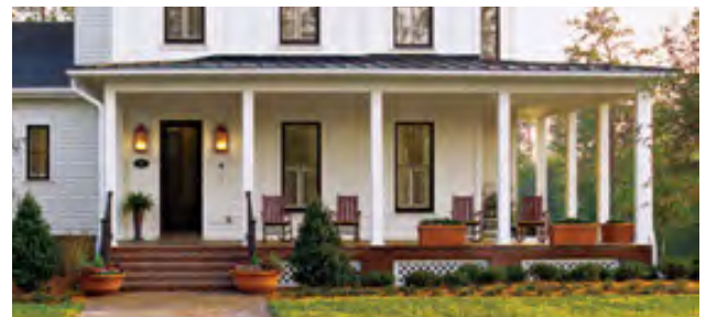
Porch raised above finished grade
