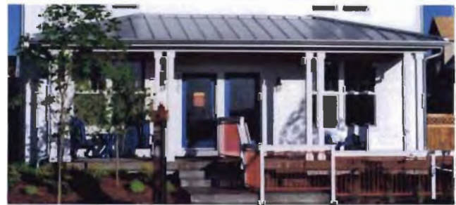
Properly detailed porch elements
