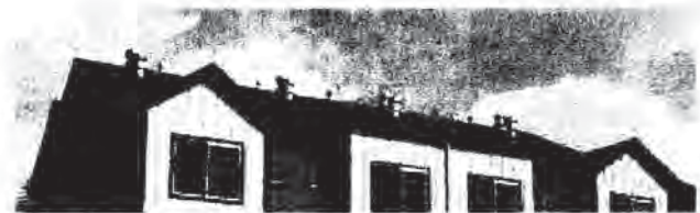
Mechanical vents reflect architectural style
