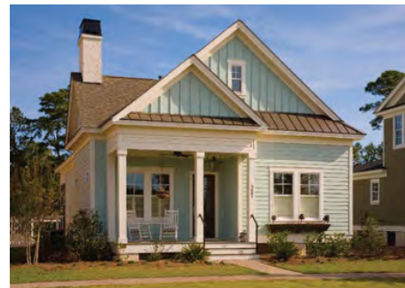
Porch roof forms are consistent with home
