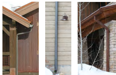
Gutters must complement the homes style
