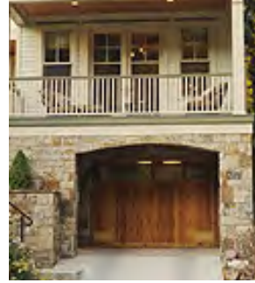
Patio over garage lessens its visual impact
