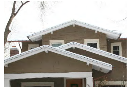
Appropriate roof overhangs
