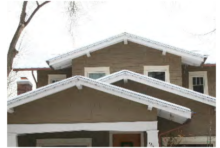
Appropriate roof overhangs
