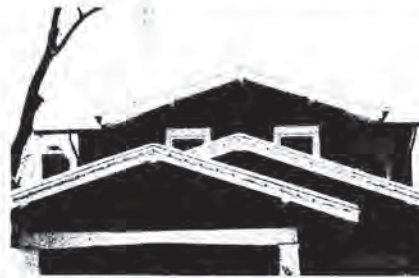
Appropriate roof overhangs
