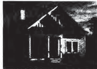
Porch roof forms are consistent with home
