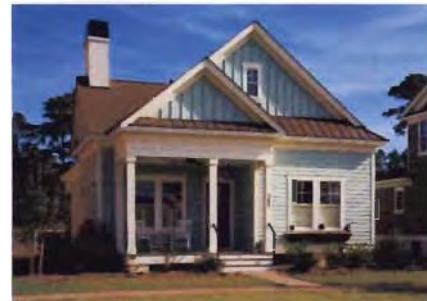
Porch roof forms are consistent with home
