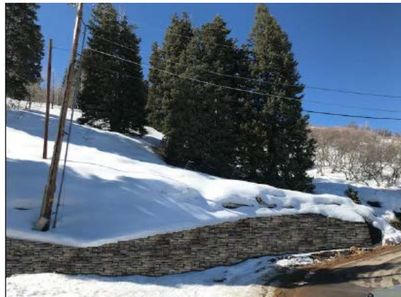
Figure 2: Photo of built wall with Veneer
