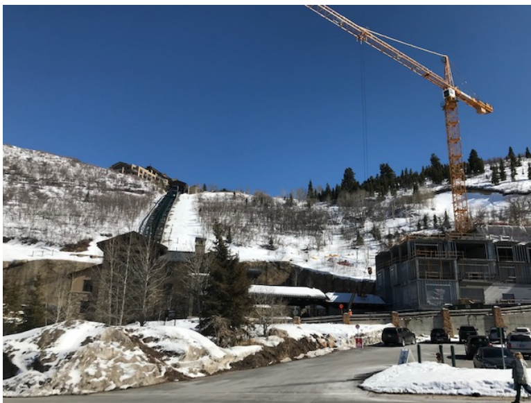
Figure 1: Phase 2 of the St. Regis Under Construction
