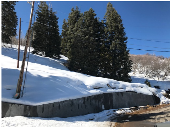
Figure 1: Photo of built wall
