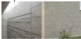
MASONRY BRICK/ARCHITECTURAL CONCRETE
