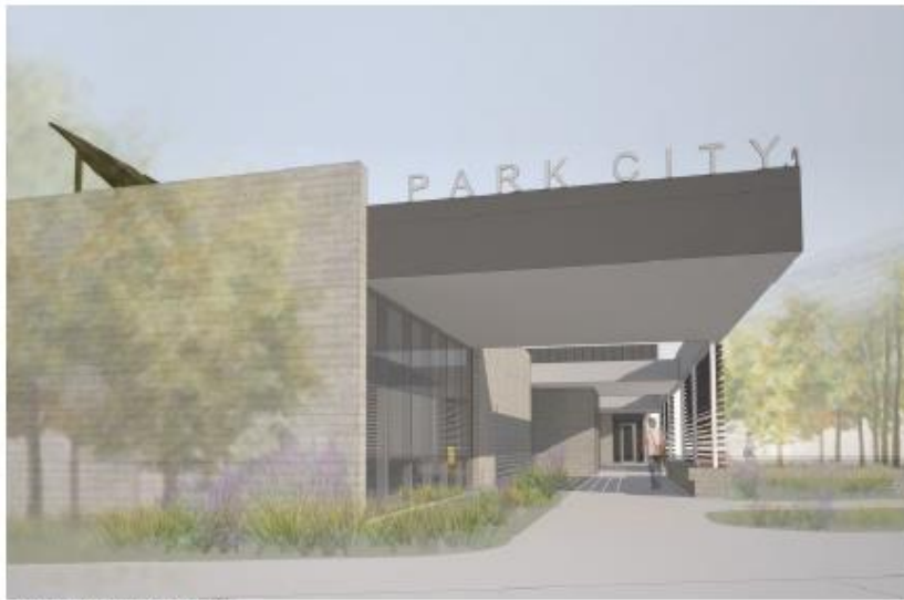
VIEW LOOKING EAST AT COVERED ENTRY
