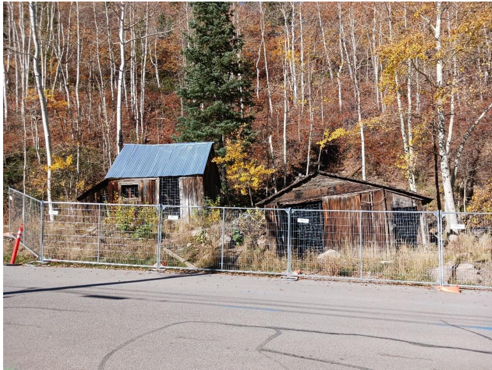
Figure 1: October 18, 2022 photograph of site including single-cell cabin (left) and single-car garage (right).
