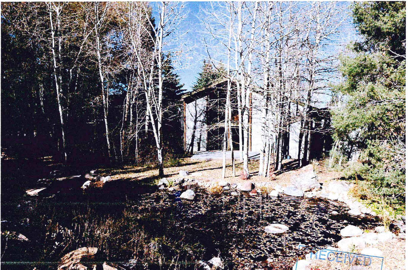
Rear, looking north
