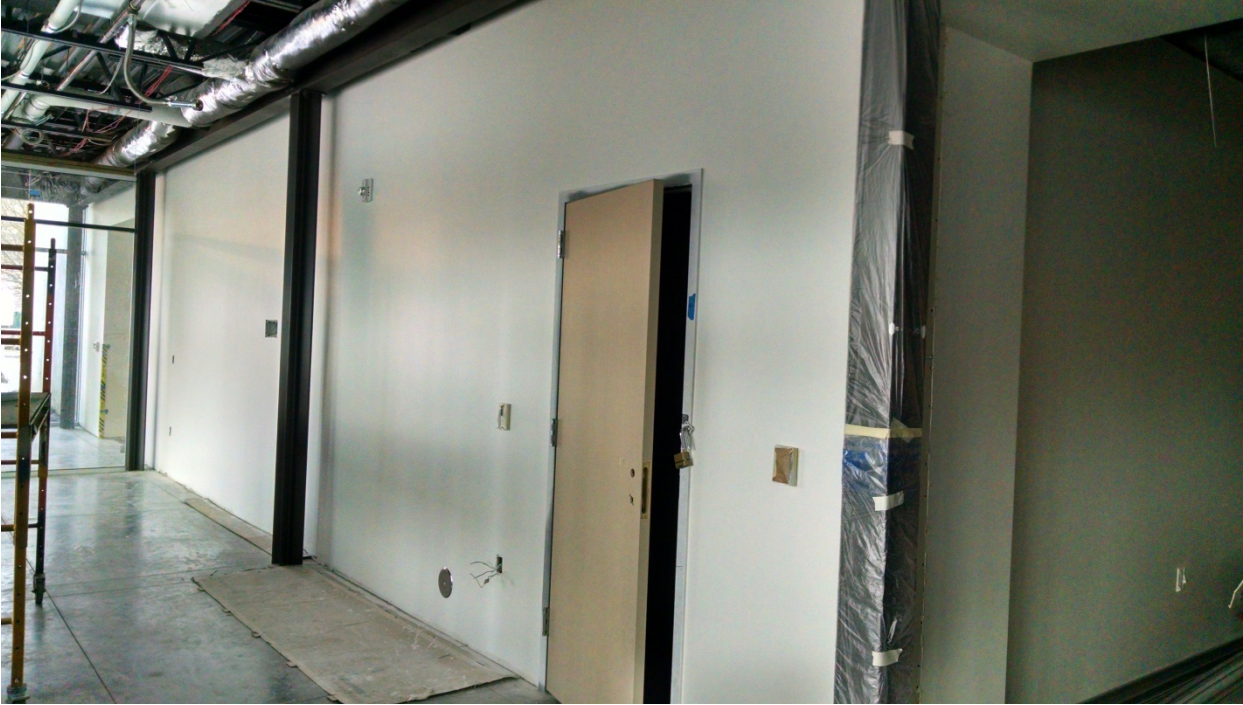
Exhibit A - Image of Library Interior Entry Hall Space, provided to artists in RFP process.
