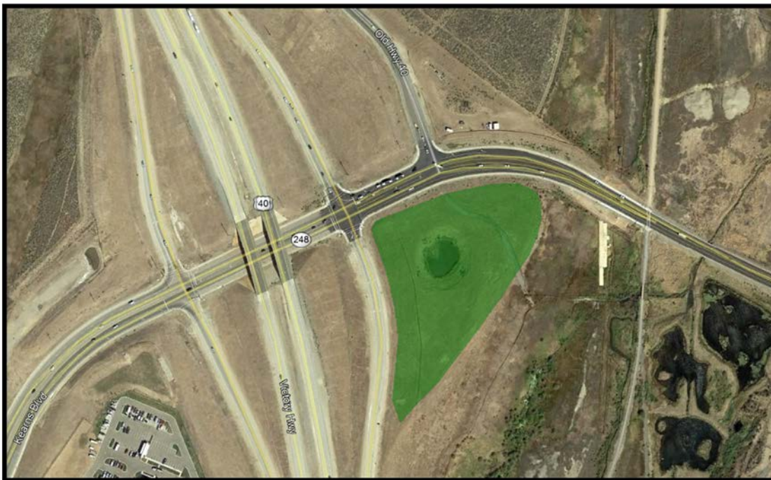
Figure 4 - UDOT Detention Basin Site- (Source: Google Earth)
