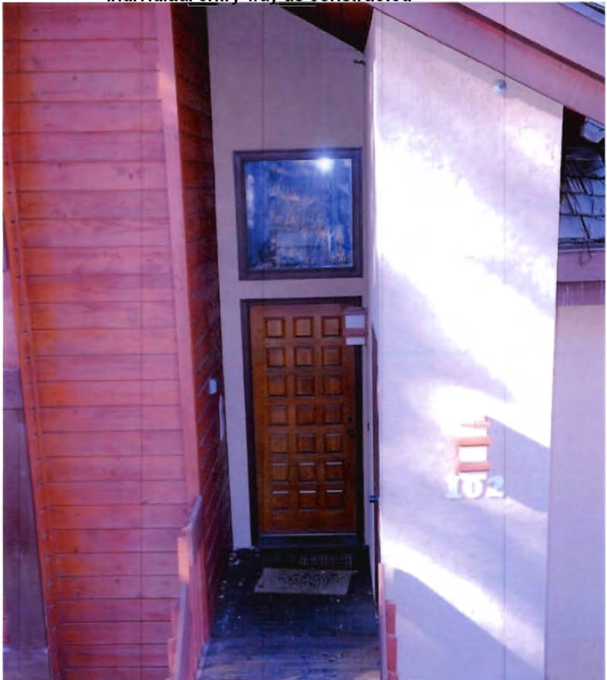
Individual entry-way as constructed
