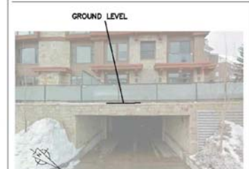
VIEW LOOKING SOUTHWEST
