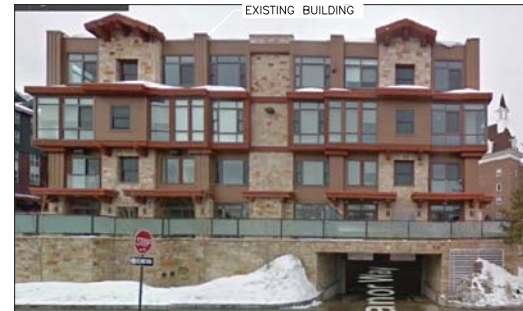
VIEW OF EXISTING BUILDING (LOOKING SOUTHEAST)
