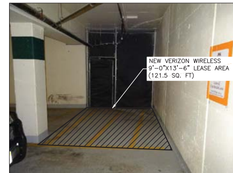
VIEW OF NEW LEASE AREA "1" (IN PARKING STRUCTURE)
