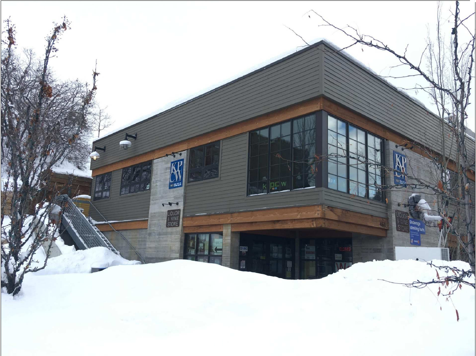
Unit 200, Marsac-Swede Condominiums - looking easterly
