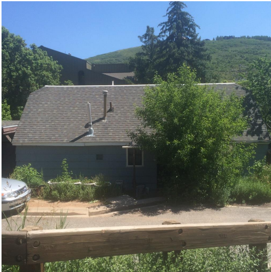
1302 Norfolk Avenue. West Elevation. June 2016.
