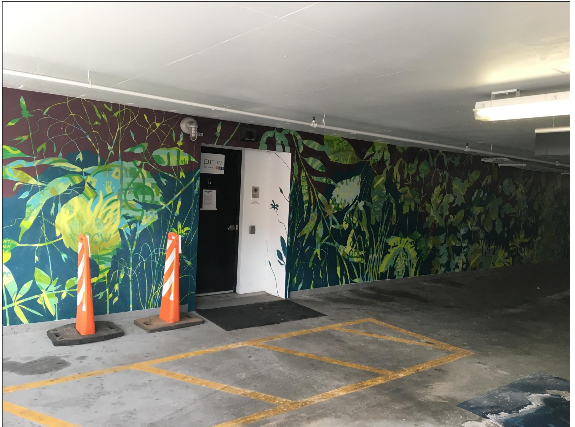
Unit 200, Marsac-Swede Condominiums - looking northerly
