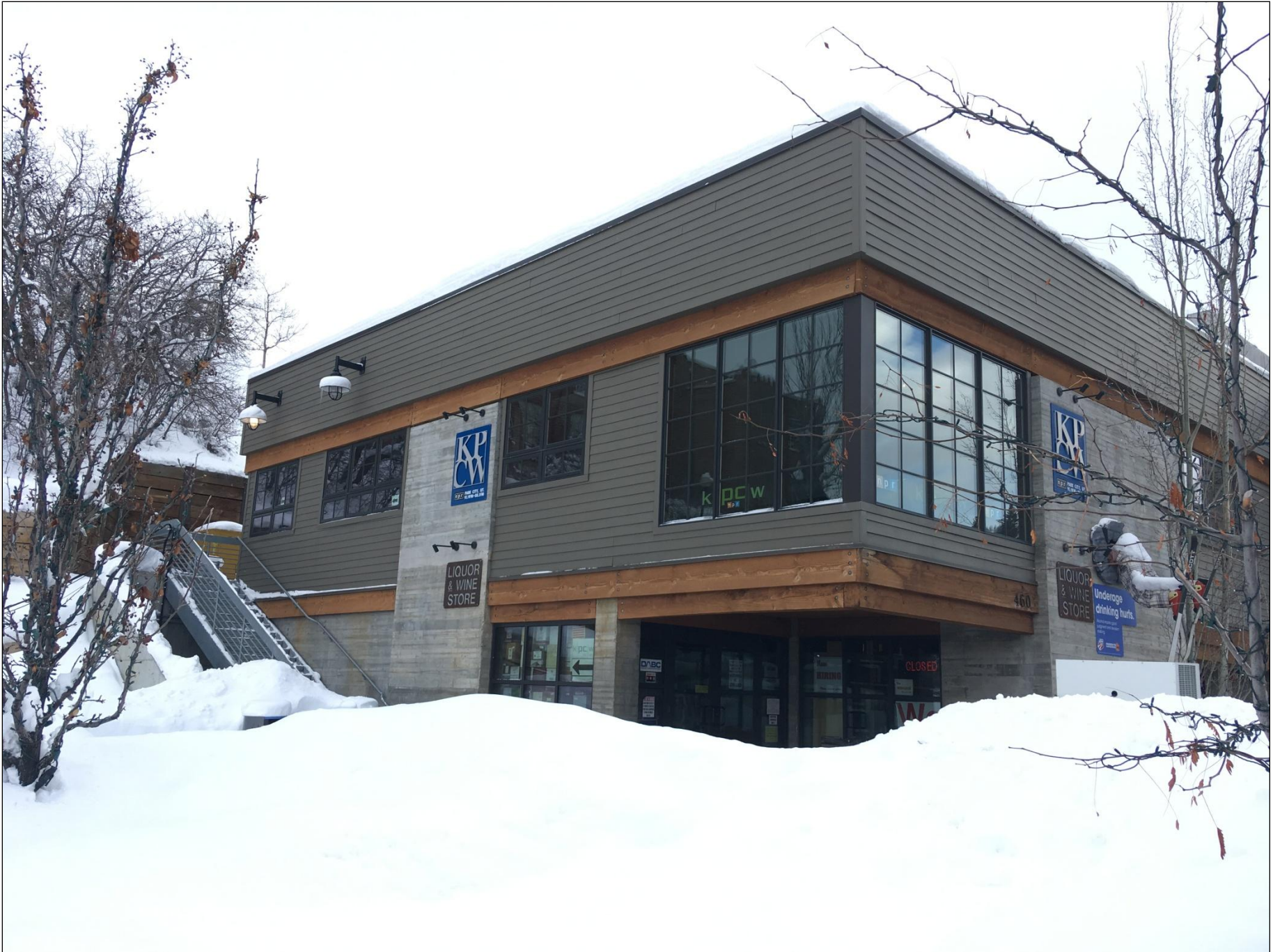
Unit 200, Marsac-Swede Condominiums - looking easterly
