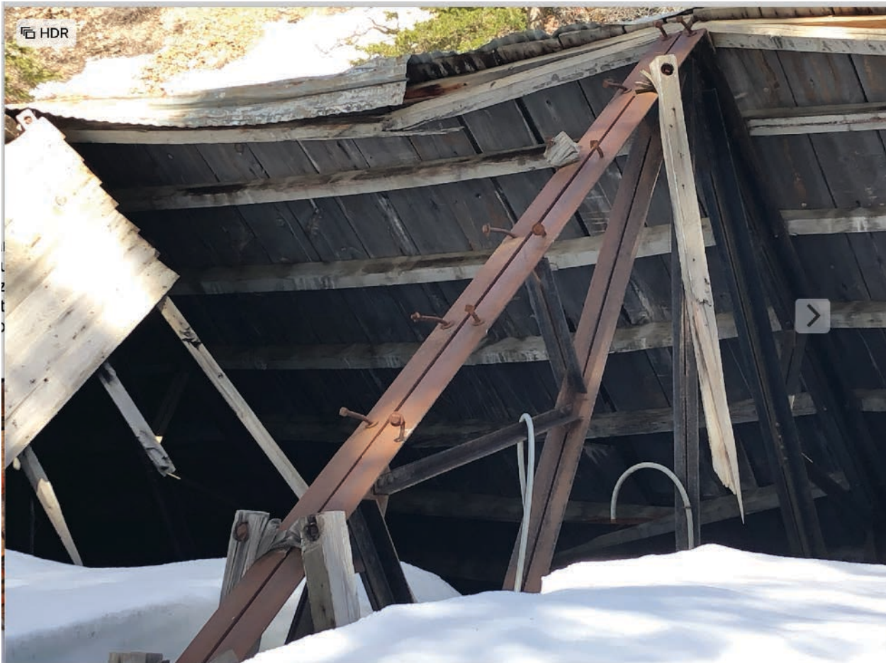
Judge Mining & Smelting - roof prior to repairs
