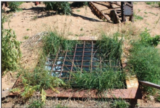
Figure 37. Detail of Daly-West Mine Shaft, facing southeast.
