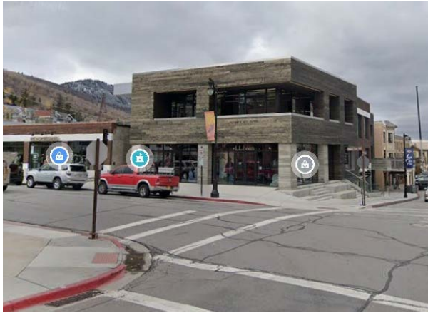
Modern Building corner of Main Street and Heber Ave
