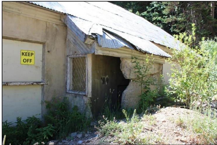
Figure 7. Entrance on northwest side of building, facing south. Note damaged roofing and deteriorated concrete, as well as earth piled against the building.
