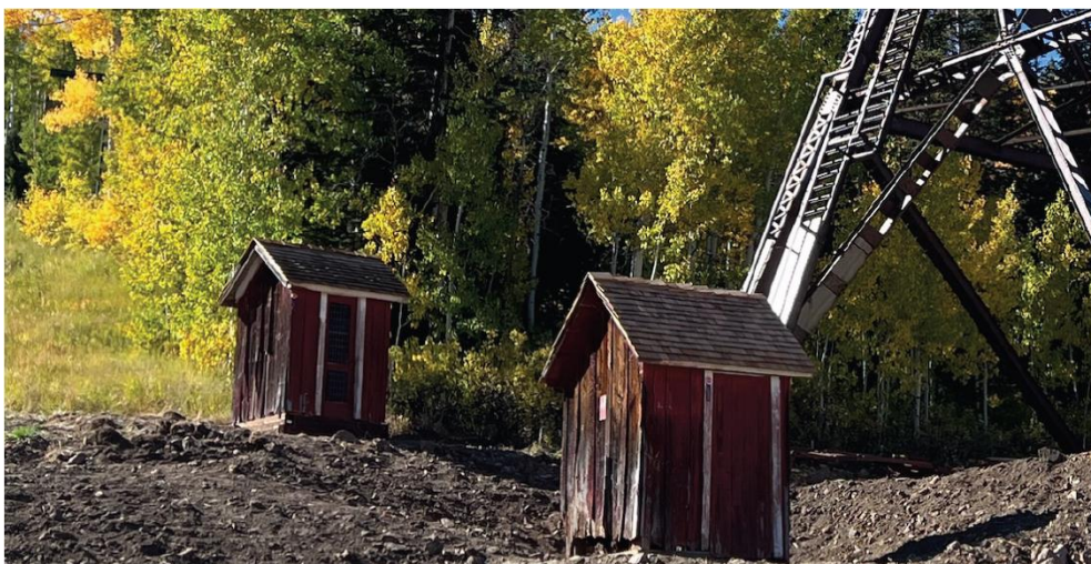
Figure 1: Fire Hydrant Shacks at Daly West Shaft
