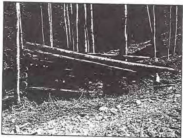
Figure 47 – West side of log structure.
