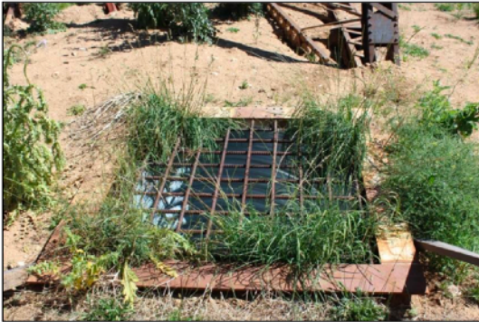
Figure 37. Detail of Daly-West Mine Shaft, facing southeast.
