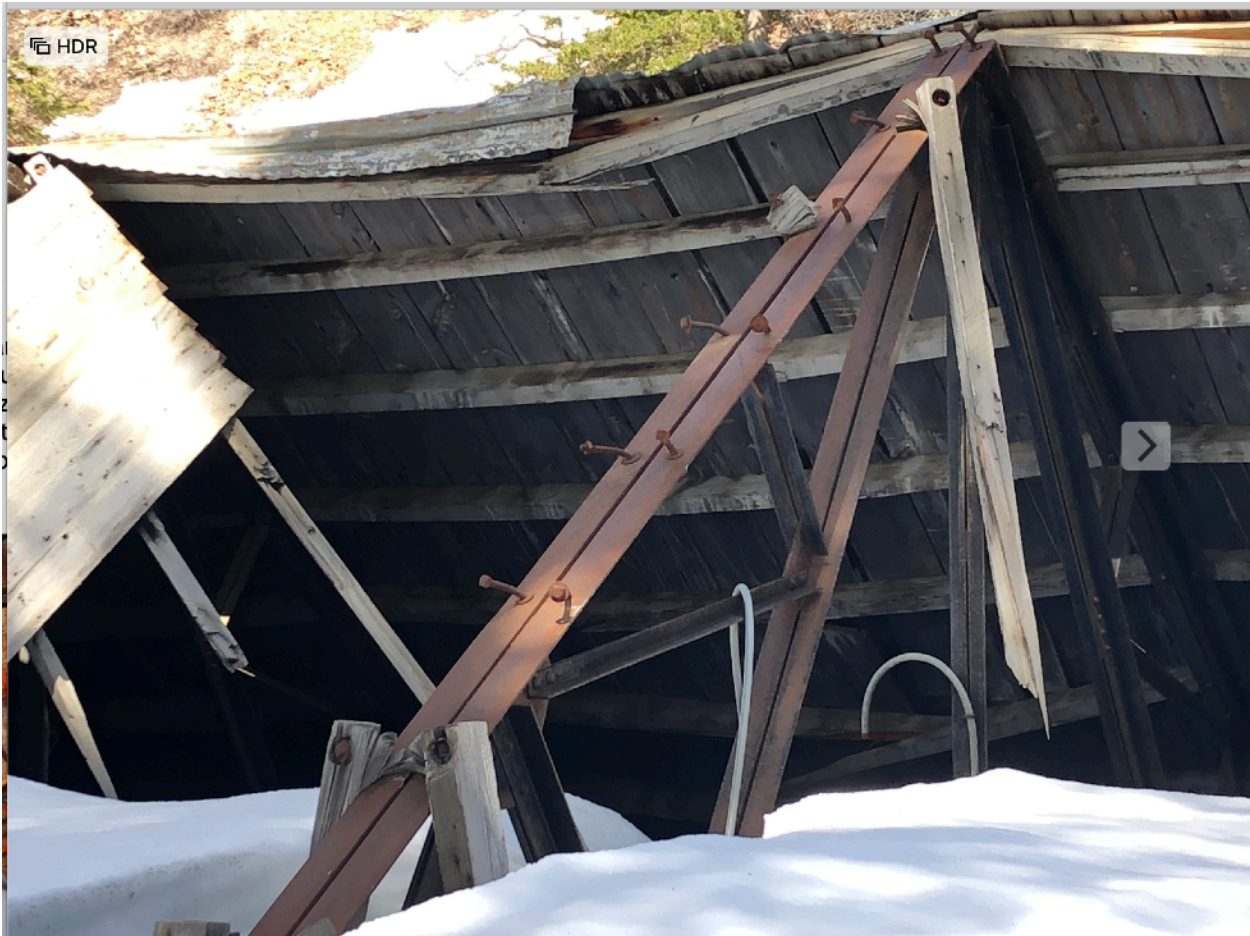
Judge Mining & Smelting - roof prior to repairs
