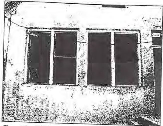
Figure 20 – Window frames in front wall.
