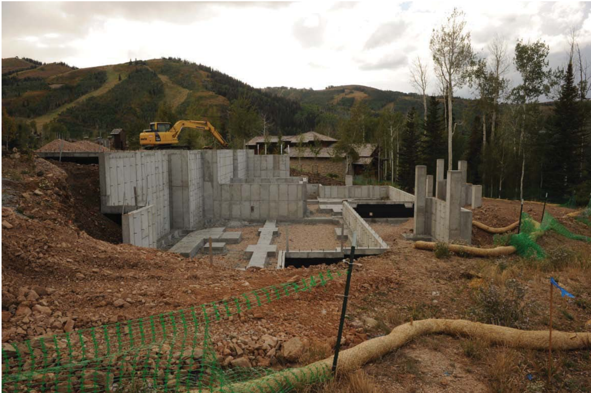
The Belles at Empire Pass, Units 13 & 14, looking west
