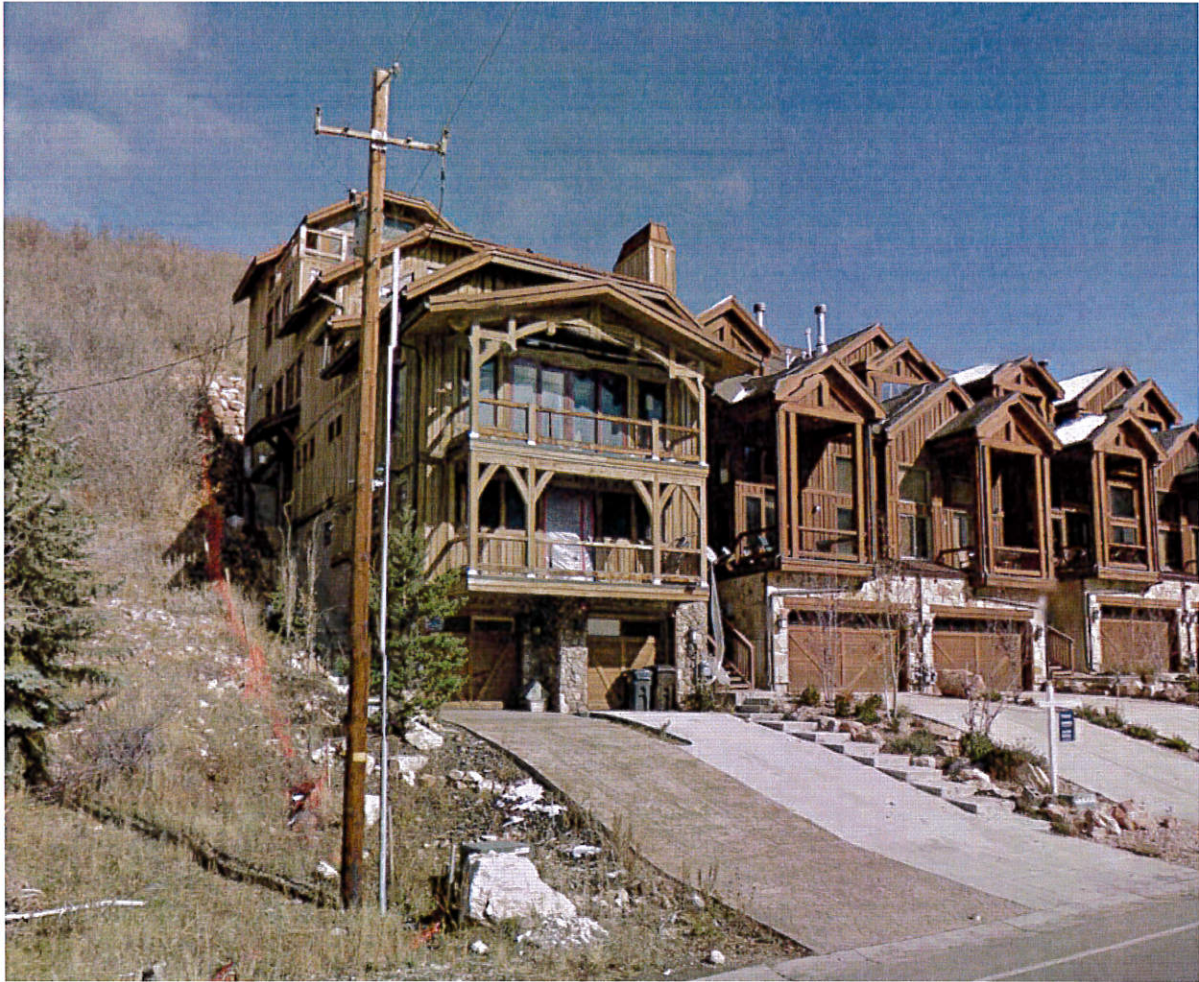
Figure 1: View Looking North East Photo
