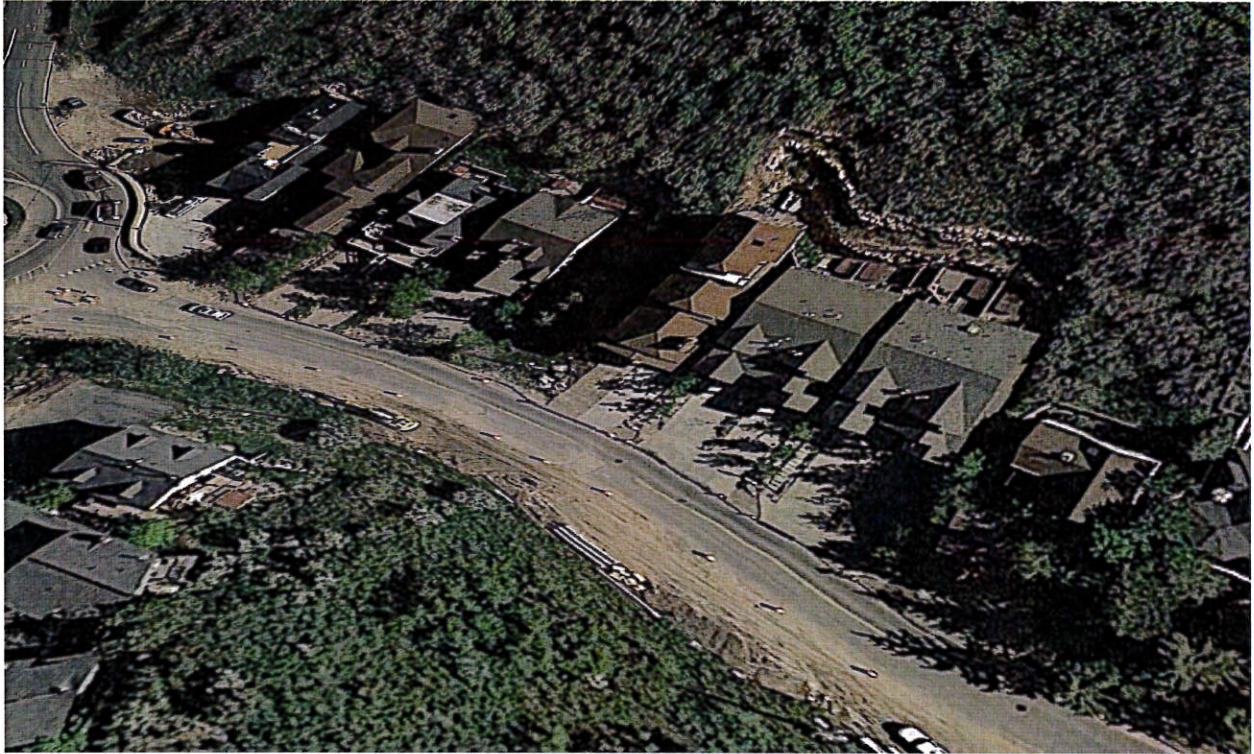
Figure 4: View Looking North West Aerial
