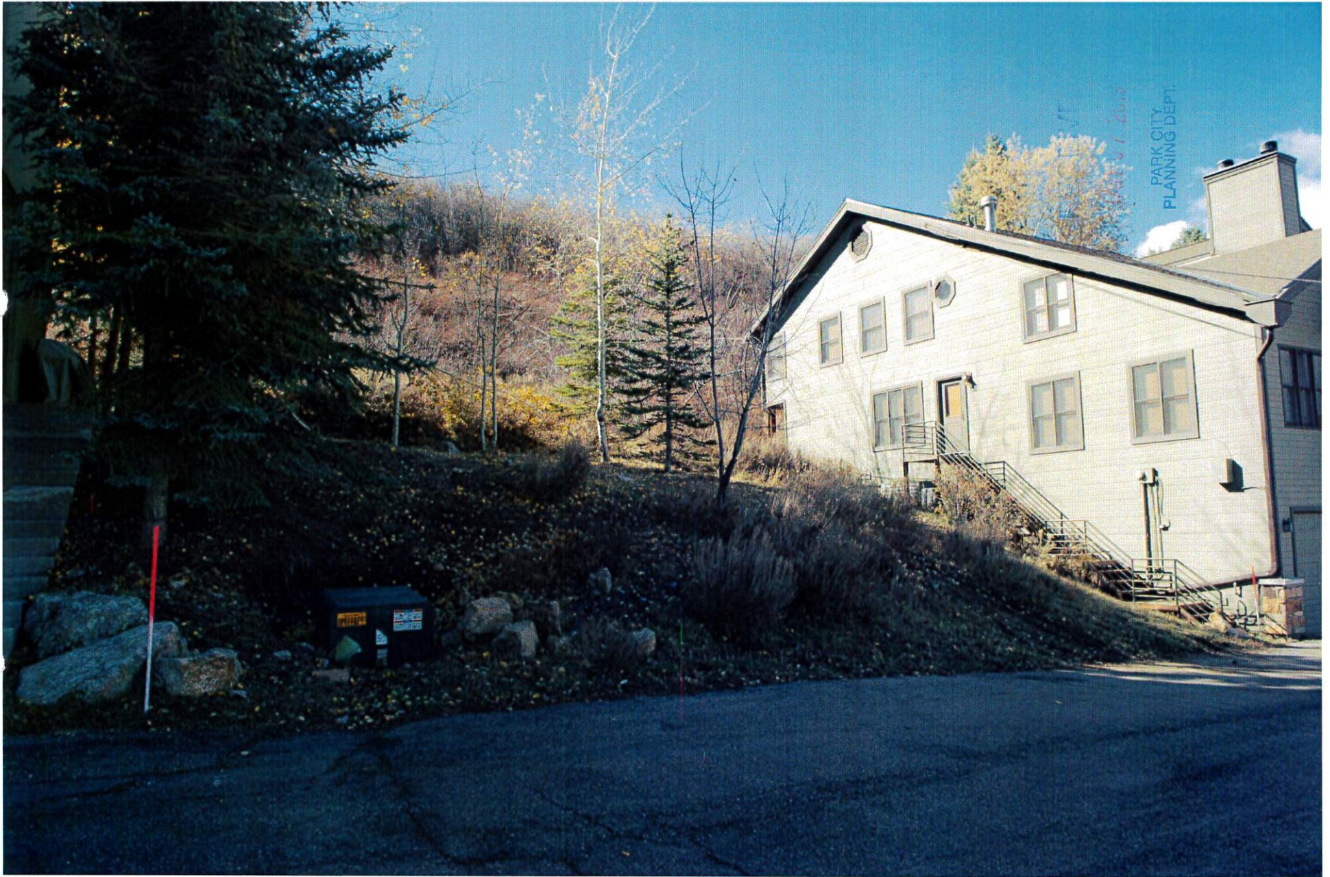
1137 Lowell Avenue - looking westerly from private driveway
