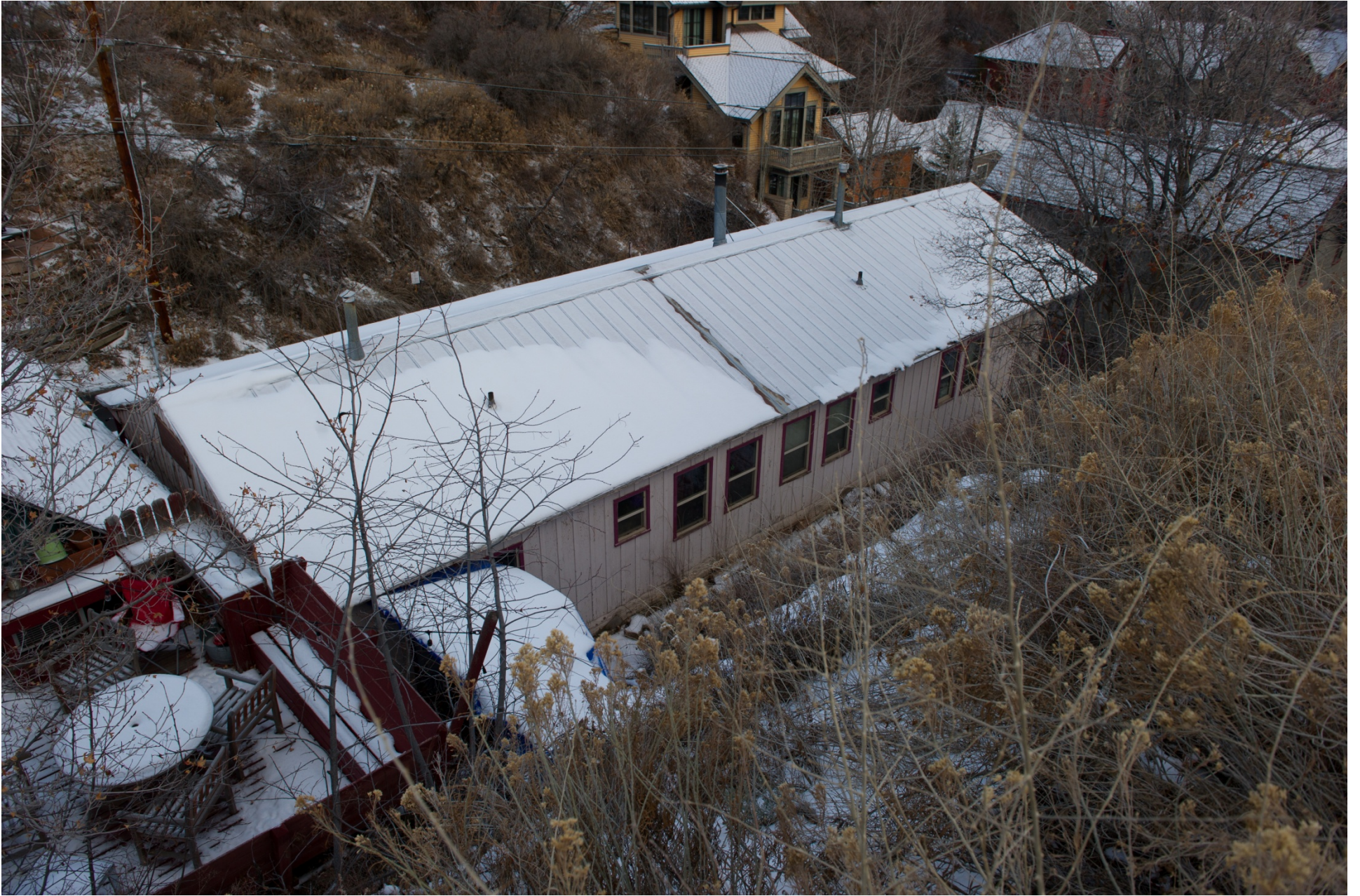
89 King Road - looking northwesterly
