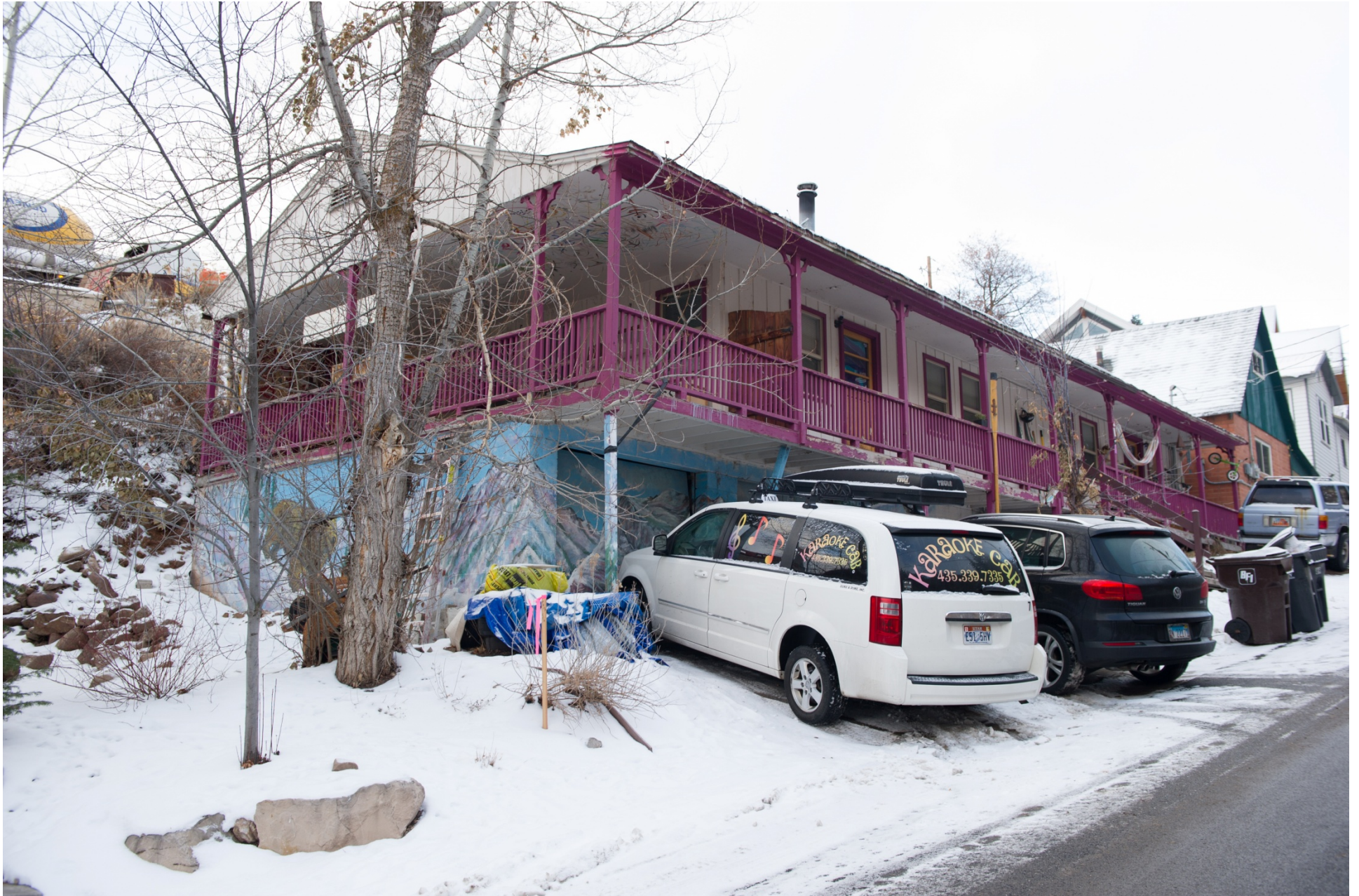
89 King Road - looking southerly
