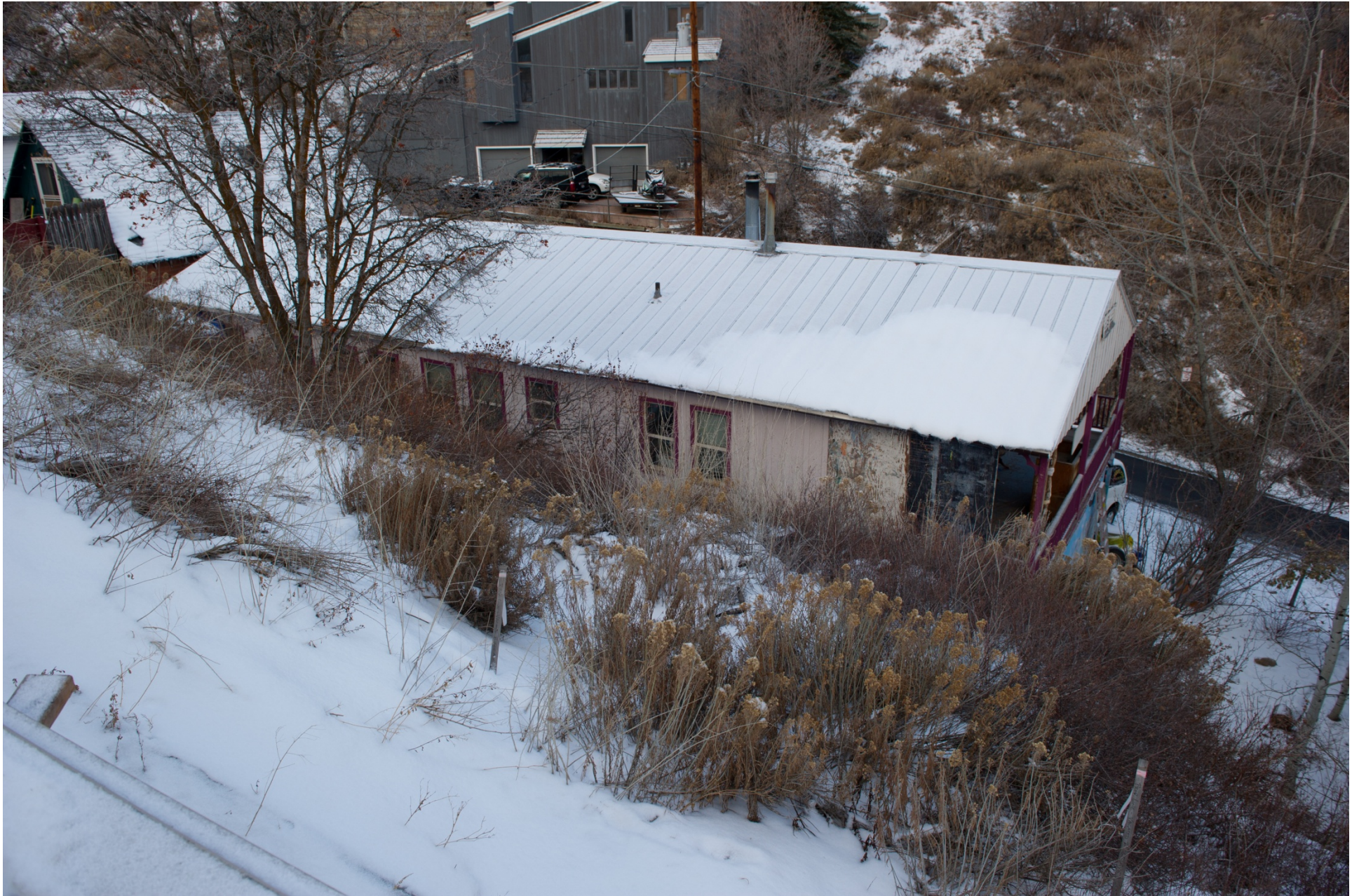
89 King Road - looking westerly
