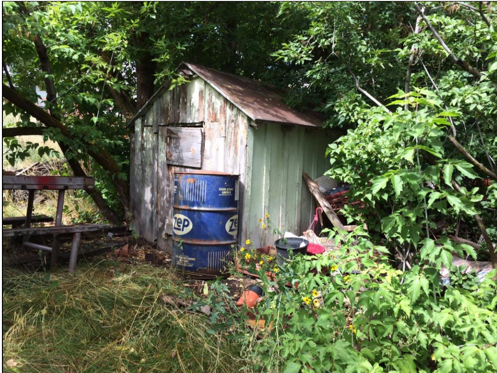
Figure 8. General view of storage shed, facing northwest.
