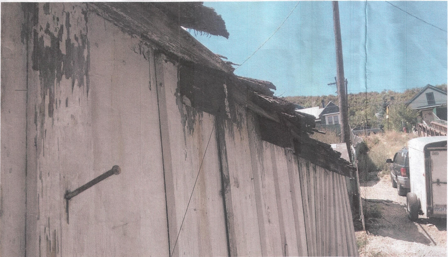
2x4 Rafters @ 24" O.C. - Wood Shingles
