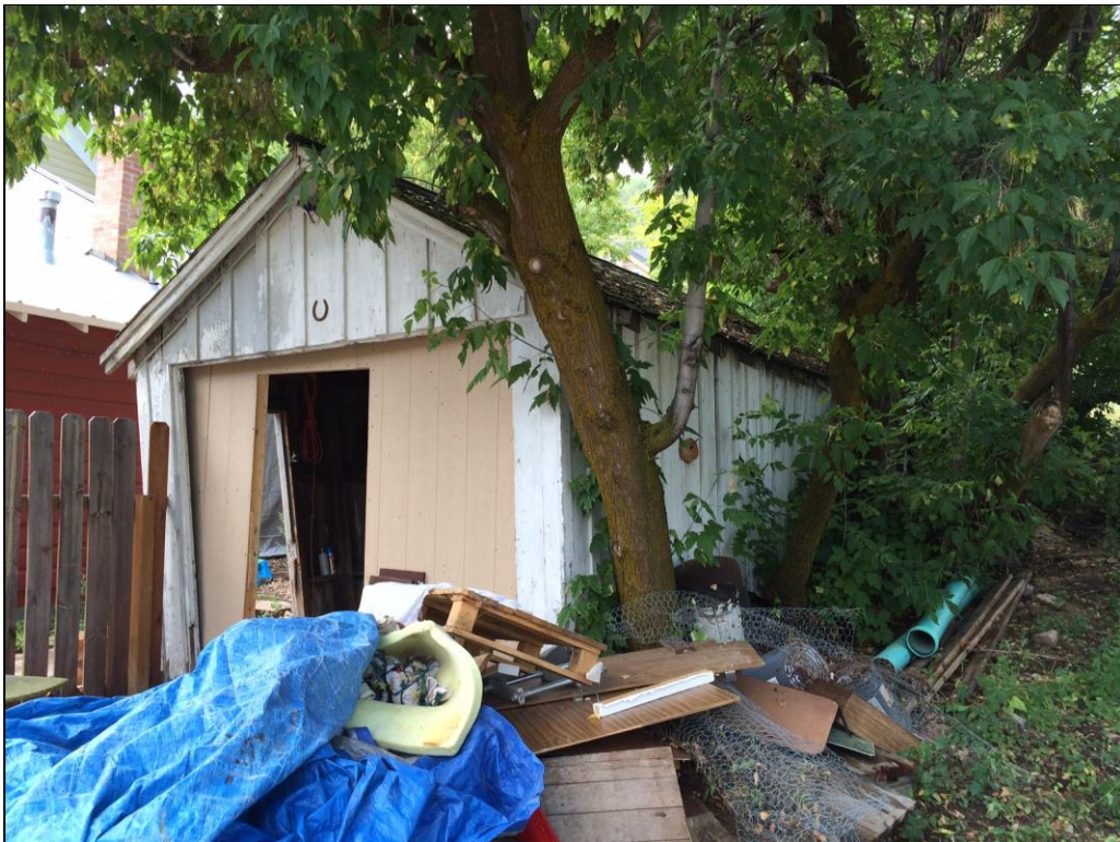
Figure 4. General view of garage, facing southwest.
