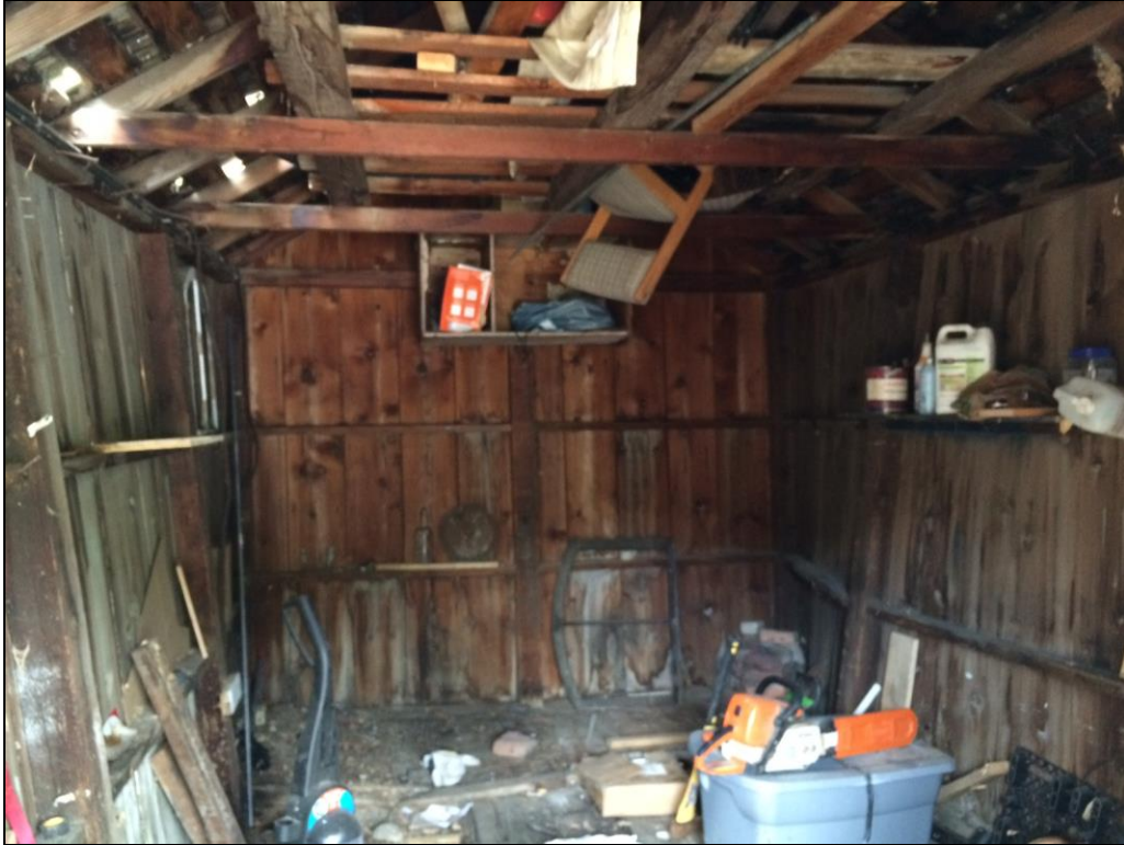
Figure 5. General view of garage interior, facing west.
