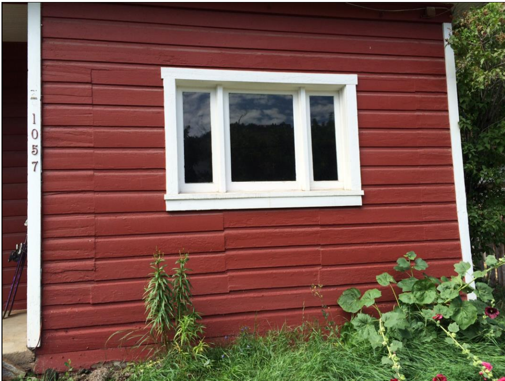
Figure 2. Detail of east façade of house, with original window locations visible in siding.
