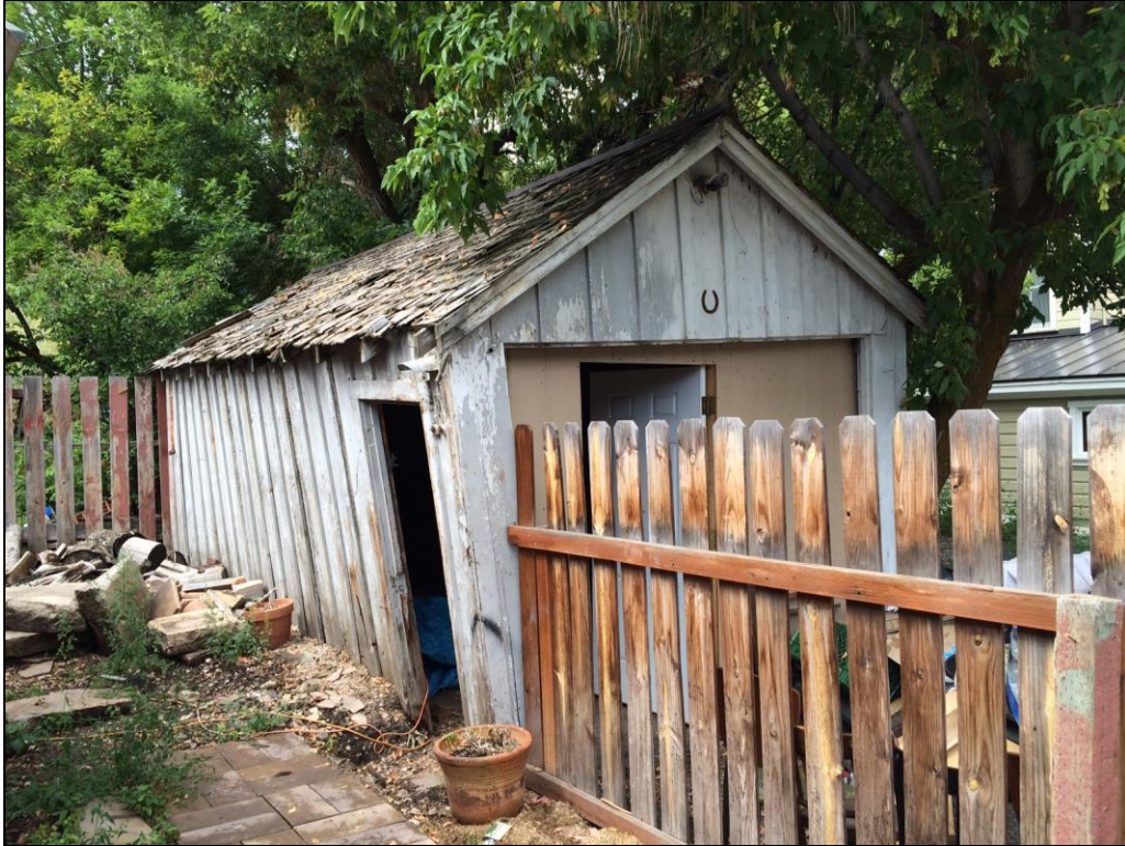
Figure 3. General view of garage, facing northwest.
