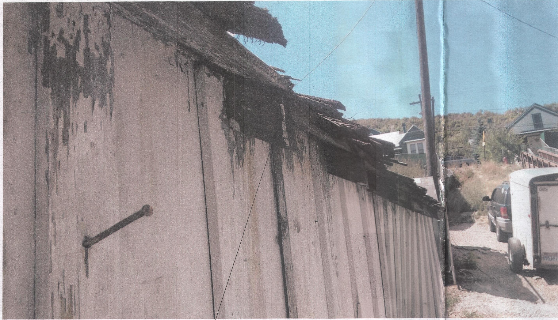
2x4 Rafters @ 24" O.C. - Wood Shingles
