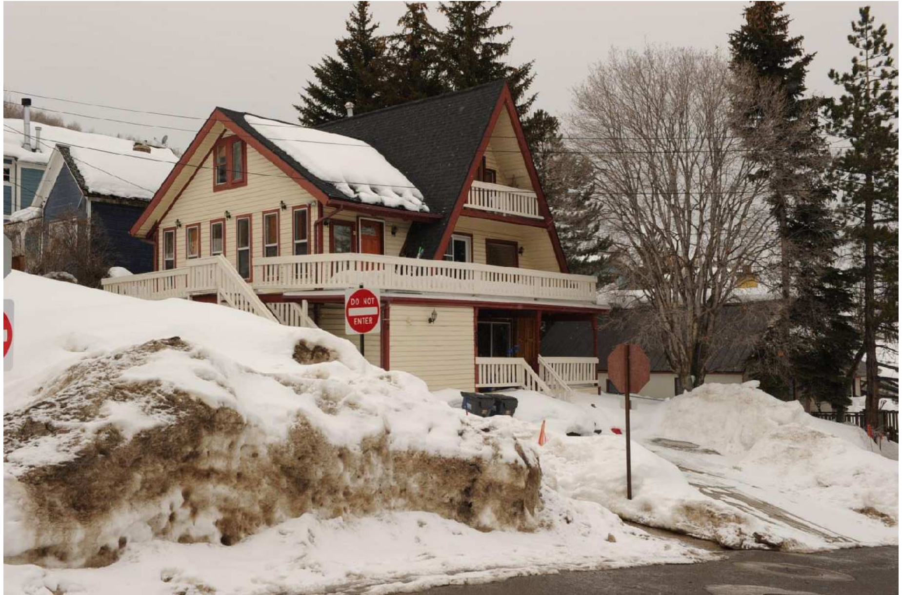
1003 Woodside Avenue – looking northwesterly
