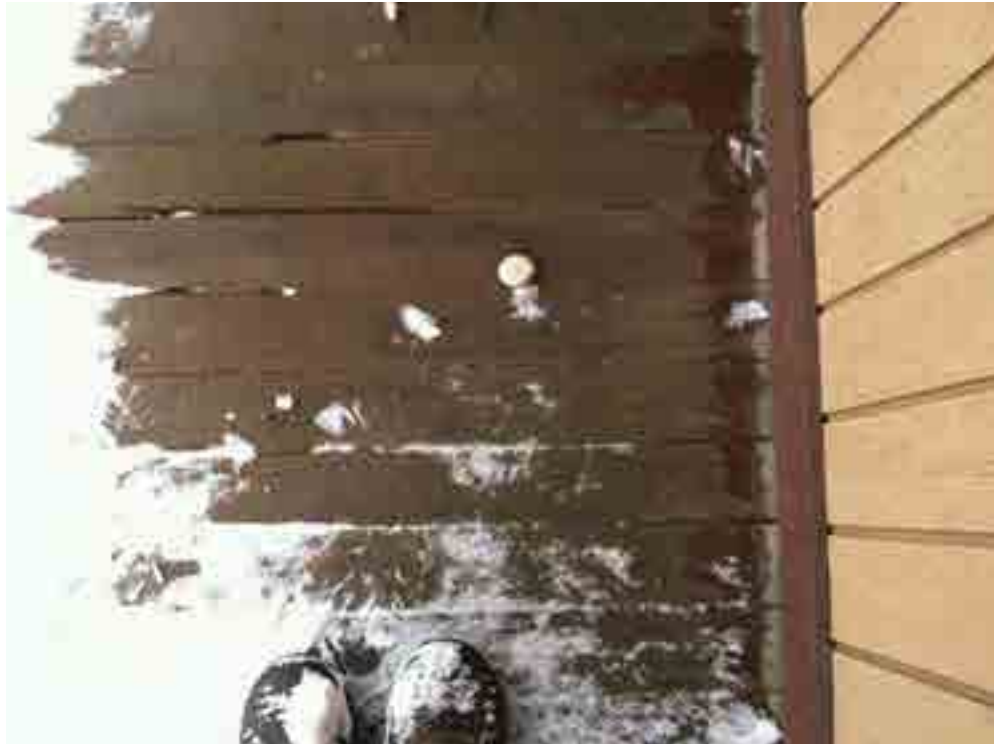
Wood floorboards on porch
