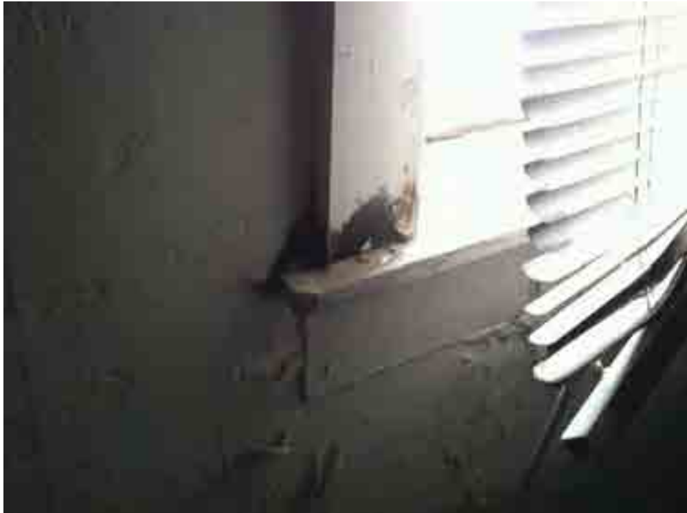
Historic interior wood window trim in front bedroom.
