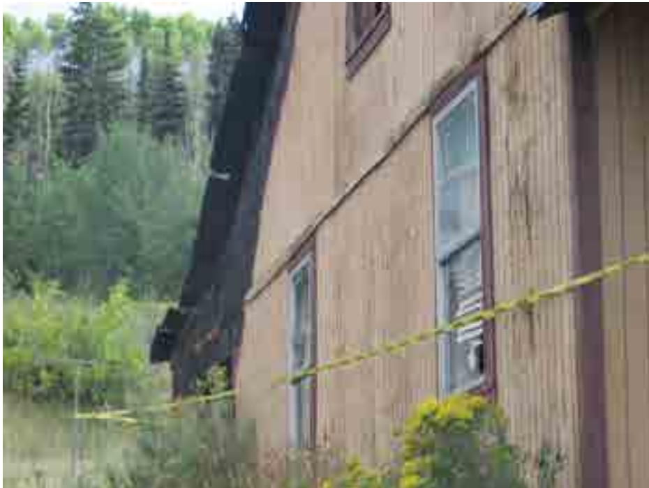
Close-up of East Elevation
