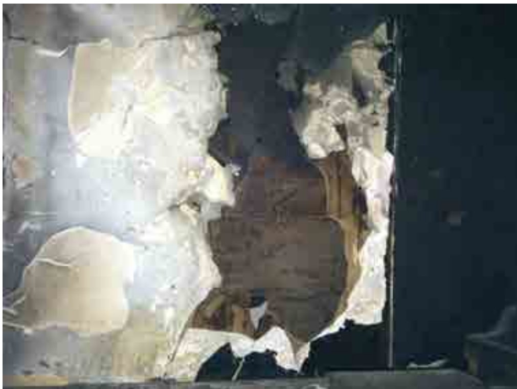
Wall paper applied atop wood wall structure
