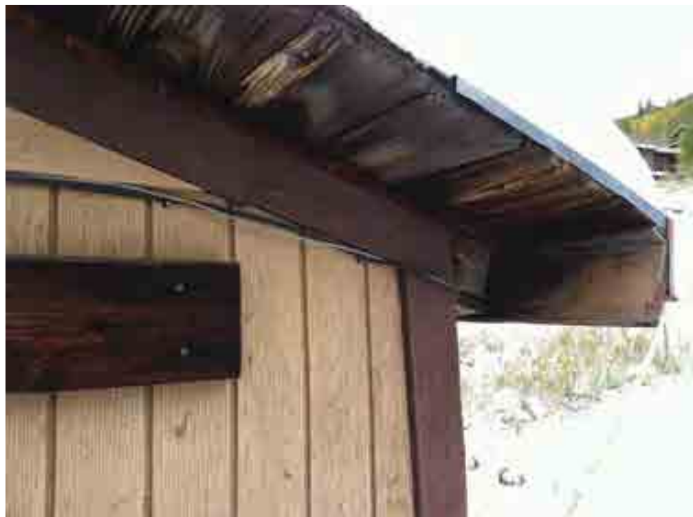
Exposed roof eave, showing old growth timber
