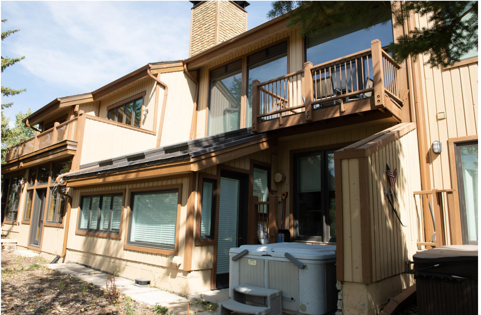
Little Belle, Unit 2 West Elevation
