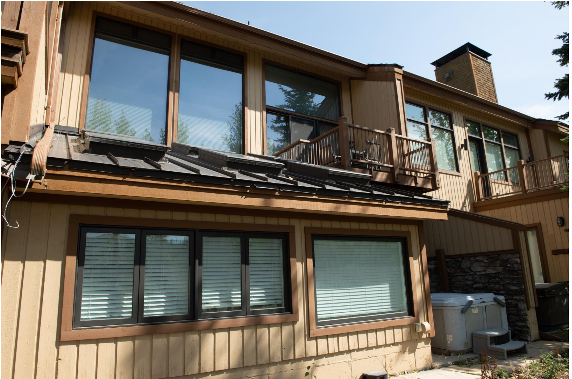
Little Belle, Unit 2 West Elevation
