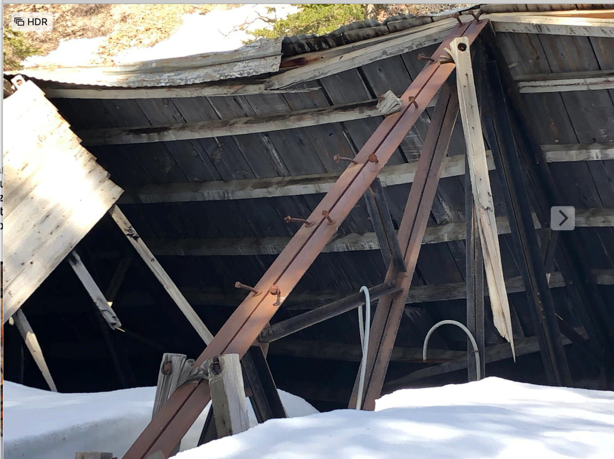
Judge Mining & Smelting - roof prior to repairs
