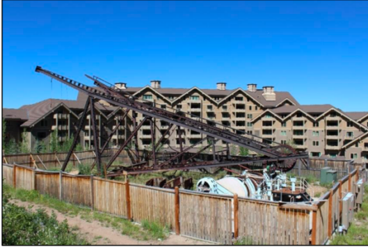
Figure 35. Overview of Daly-West Mine Headframe, Shaft, and Hoist, facing north. Note collapsed headframe.
