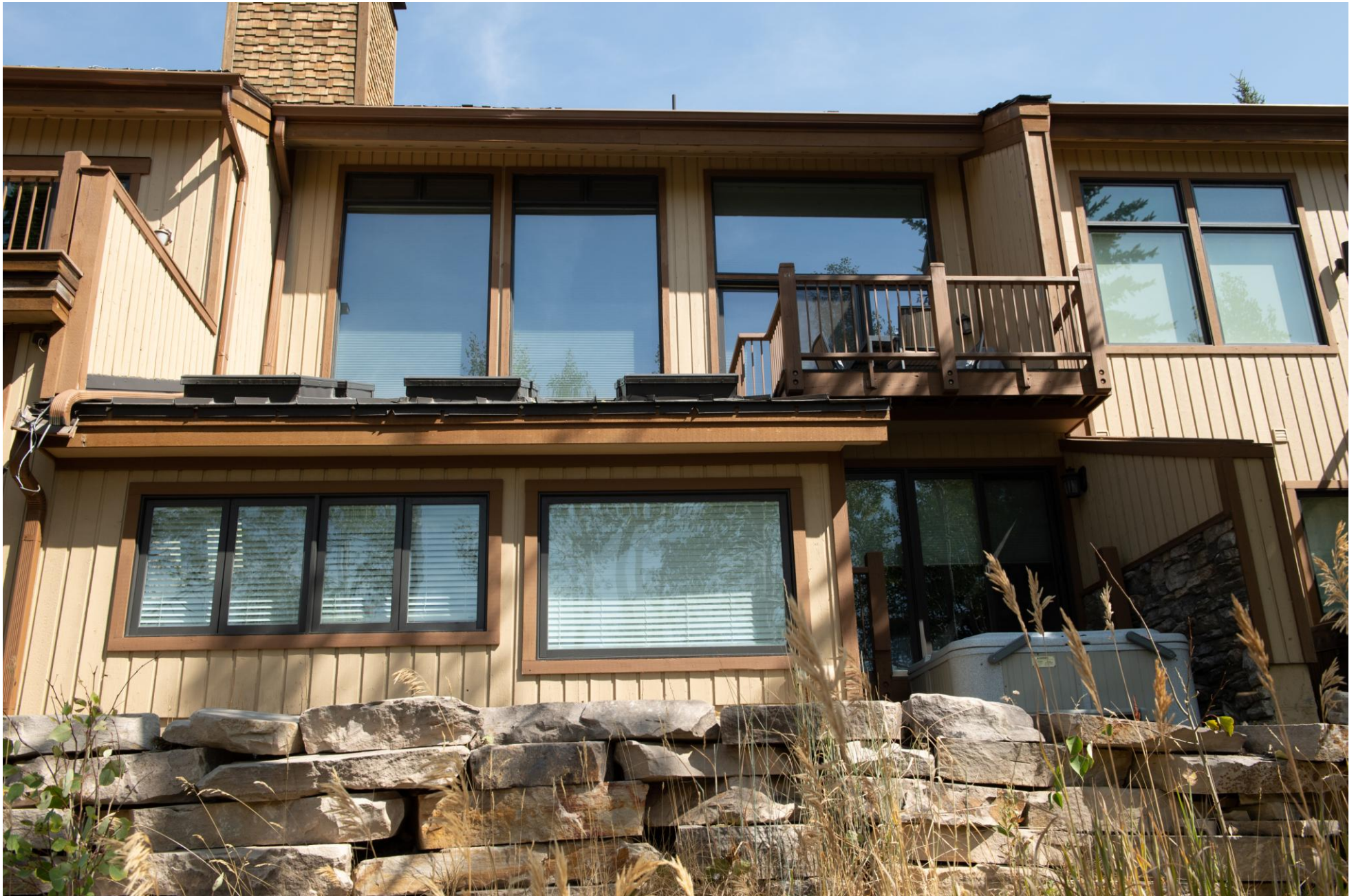
Little Belle, Unit 2 West Elevation
