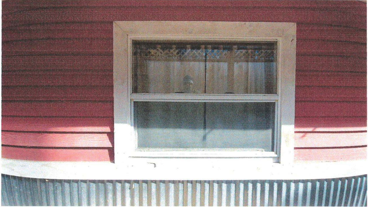
Photo 23: Rear (Window E-207) Non-Historic Addition
