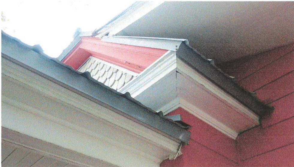
Photo 8: Soffit and Fascia
