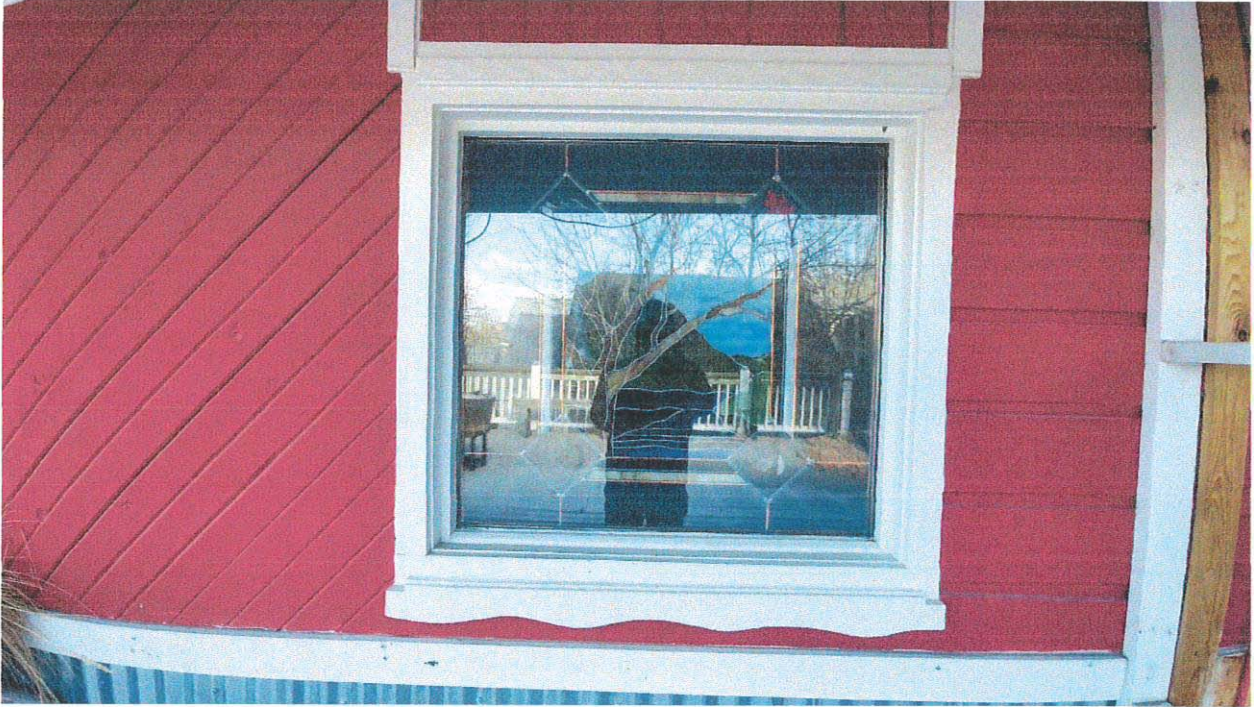
Photo 21: Deck Right Side (Window E-211) Non-Historic Addition
