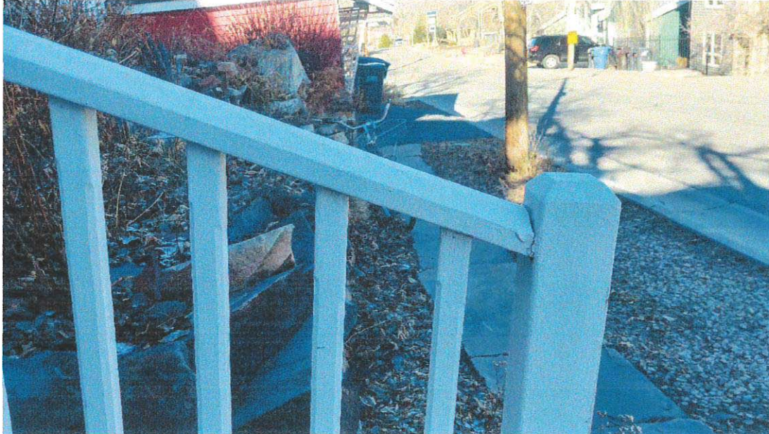
Photo 11: Front Railing Steps
