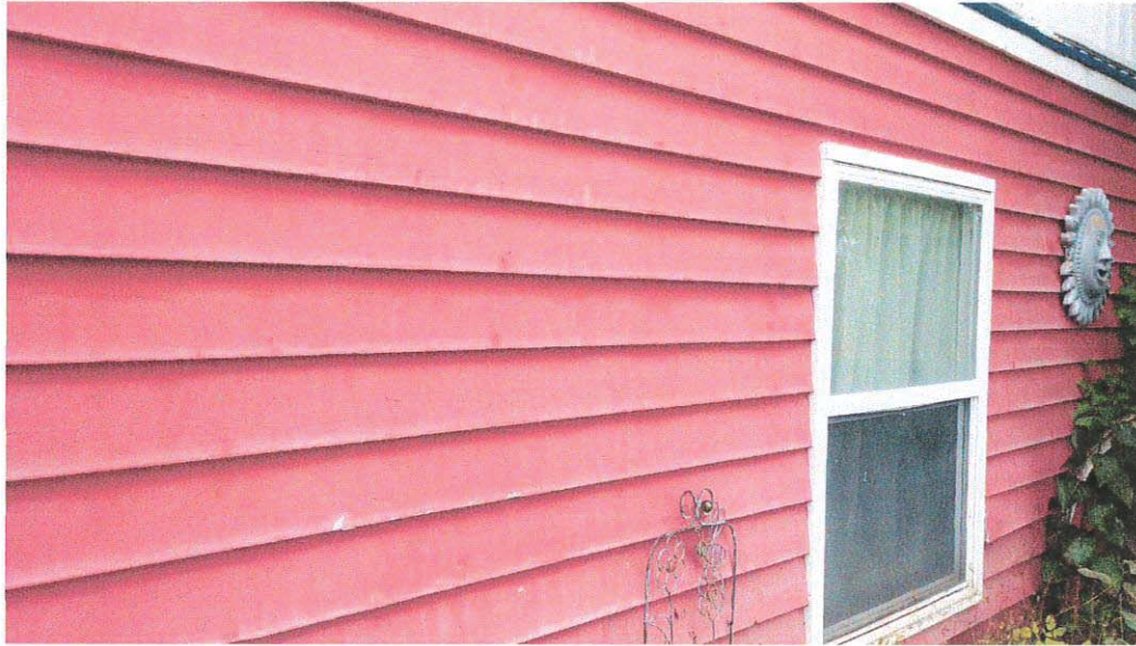
Photo 5: Siding and Window Trim
