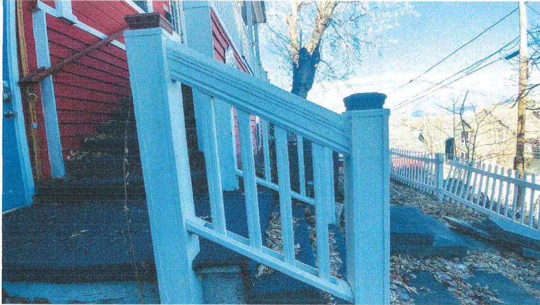
Photo 13: Railing to Front Porch
