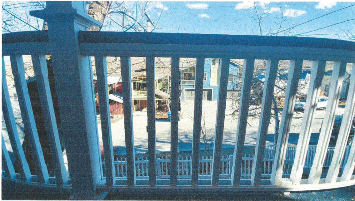
Photo 14: Front Porch Railing
