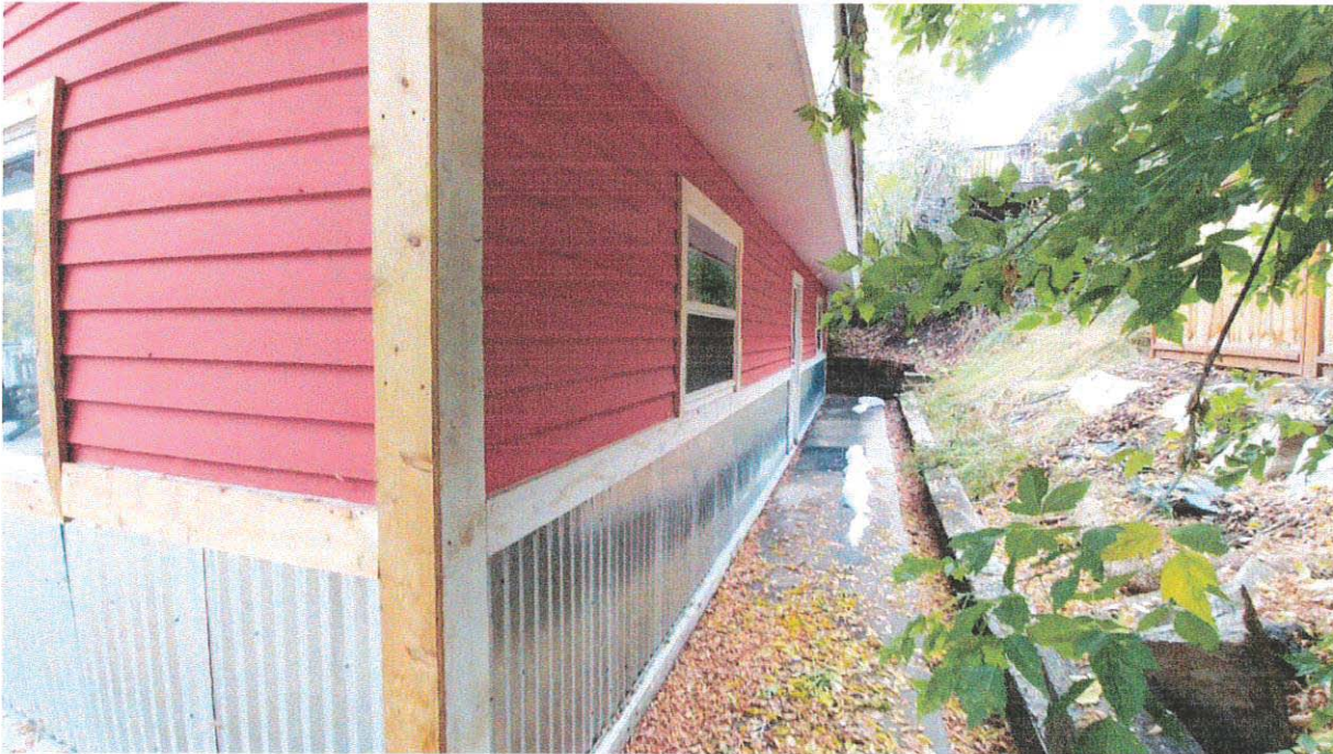
Photo 6: Rear View of Existing Home Non-Historic Addition
