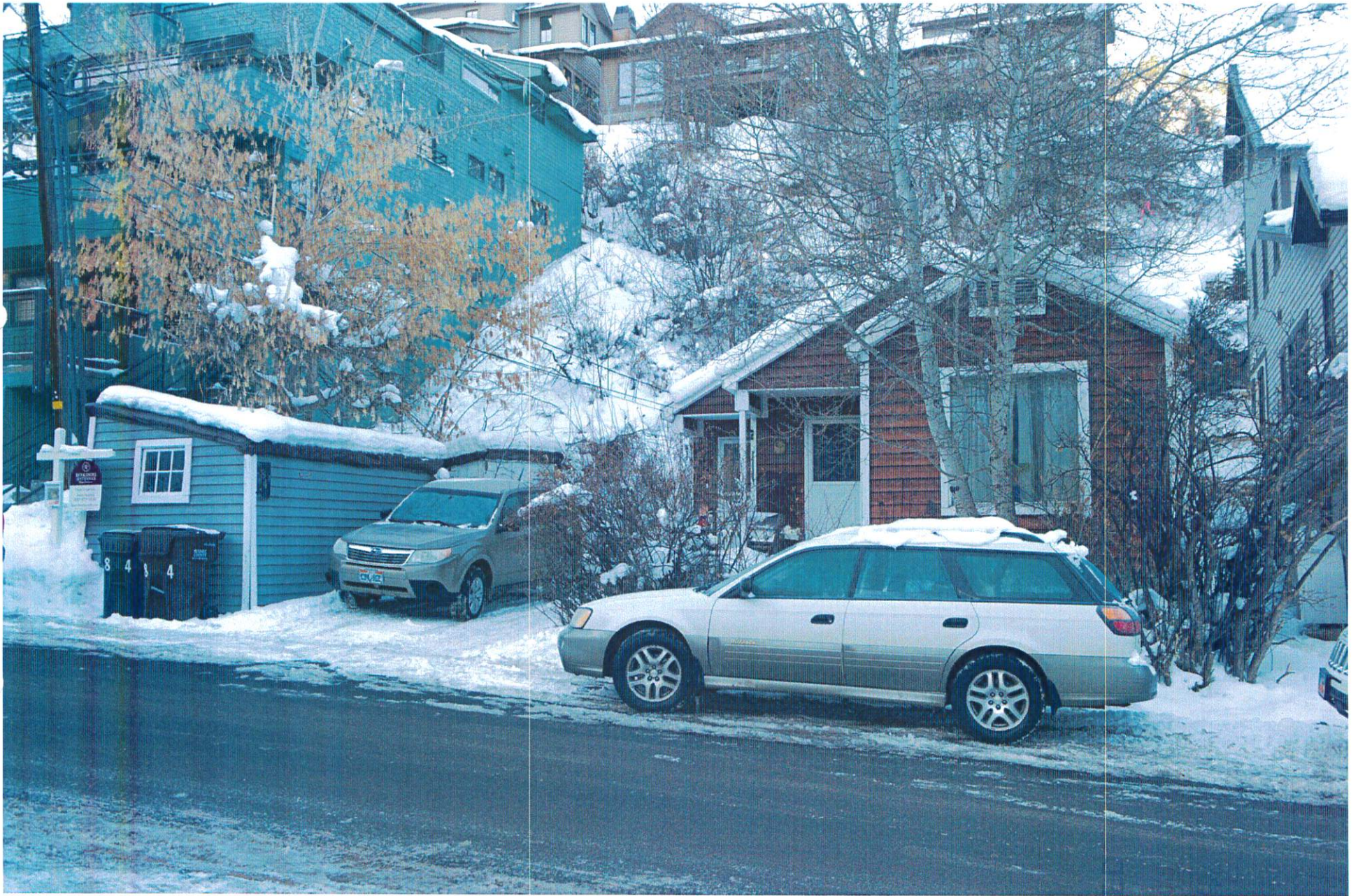
84 Daly Avenue - Looking westerly
