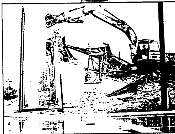
The remains of the Tarboro Depot on the morning of November 14, 1997.
