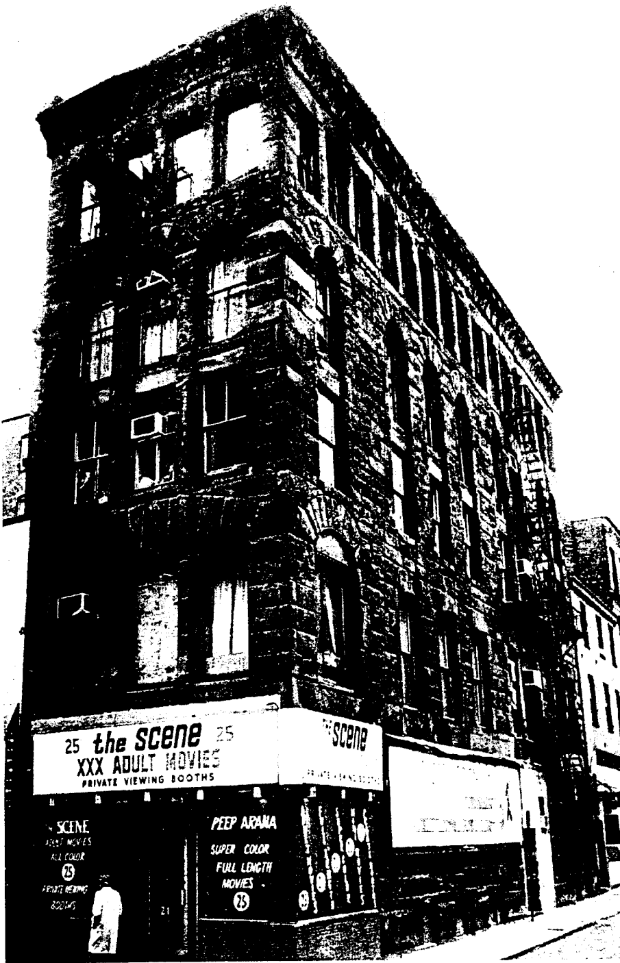
Historic Boston, Inc. has actively pursued the rehabilitation of the 1875 Hayden Building as a way to stimulate revitalization of the surrounding district. This photo shows the building after it was severely damaged by a fire in 1985.
