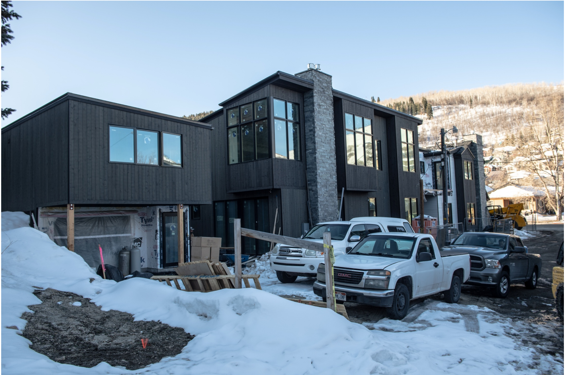
1064 Park Avenue - looking southerly
