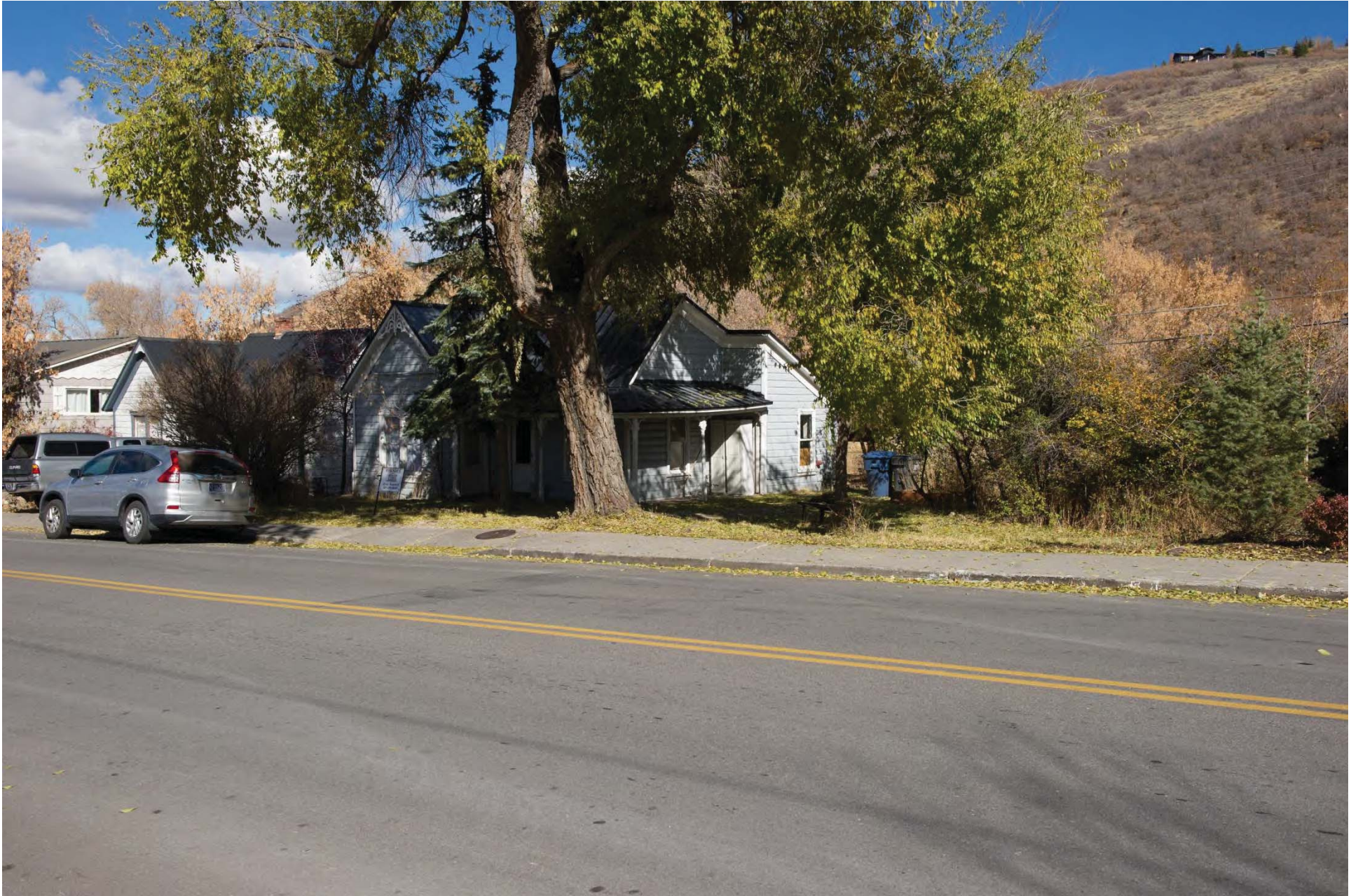
1124 & 1128 Park Avenue - looking northerly
