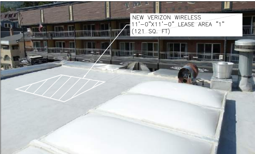
VIEW OF NEW LEASE AREA "1" (LOOKING SOUTHWEST)
