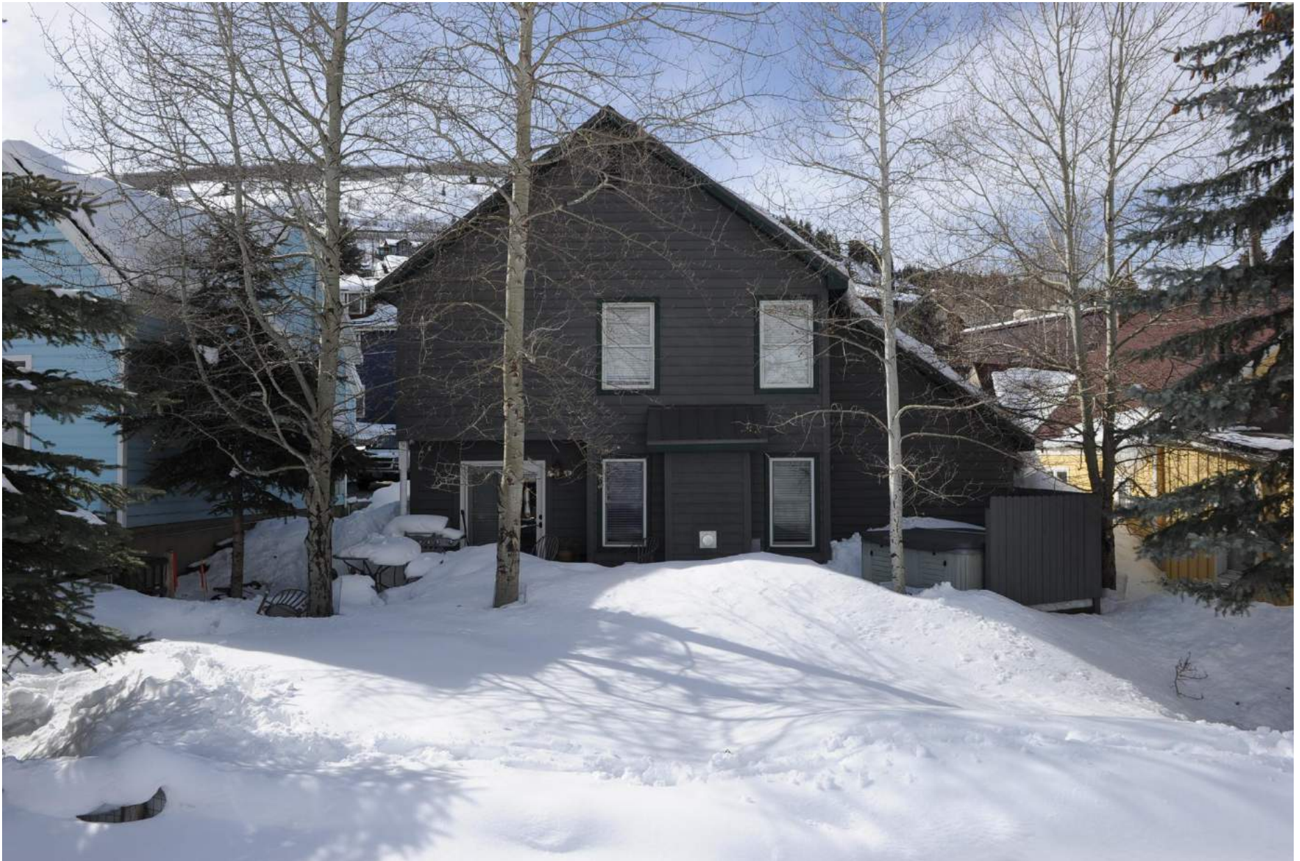
166 Main Street – looking westerly
