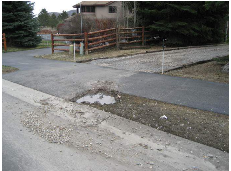
Examples of the need for gravel regulation. When laid by itself, gravel mulch often bleeds off the gravel areas and into the streets and public infrastructure systems, especially when driven over.
