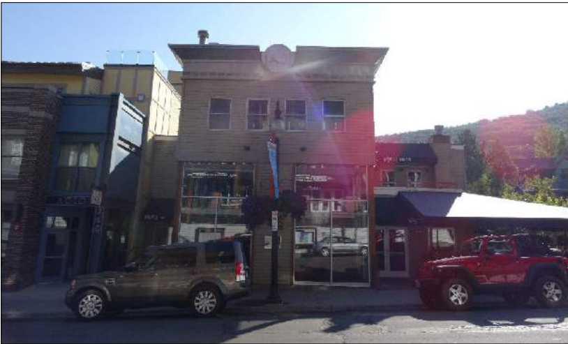
VIEW OF EXISTING BUILDING (LOOKING NORTHEAST)
