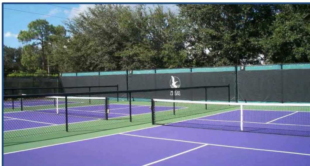
Figure 6. AcoustiFence Surrounding Pickleball Courts
