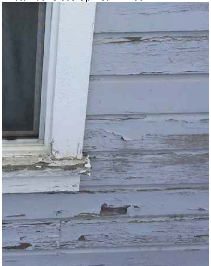
Photo #35: Close Up Near Window
