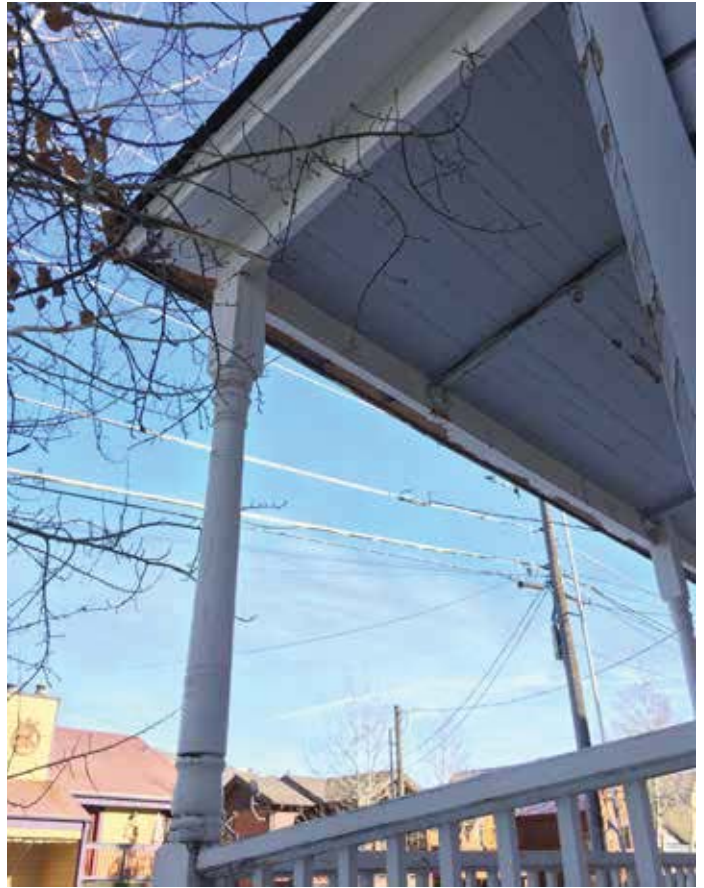
Photo #43: Underside Of Porch Roof
