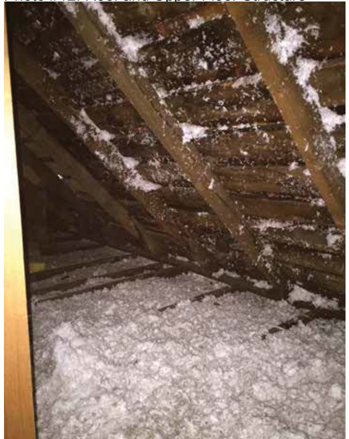
Photo #12: Roof and Upper Floor Structure
