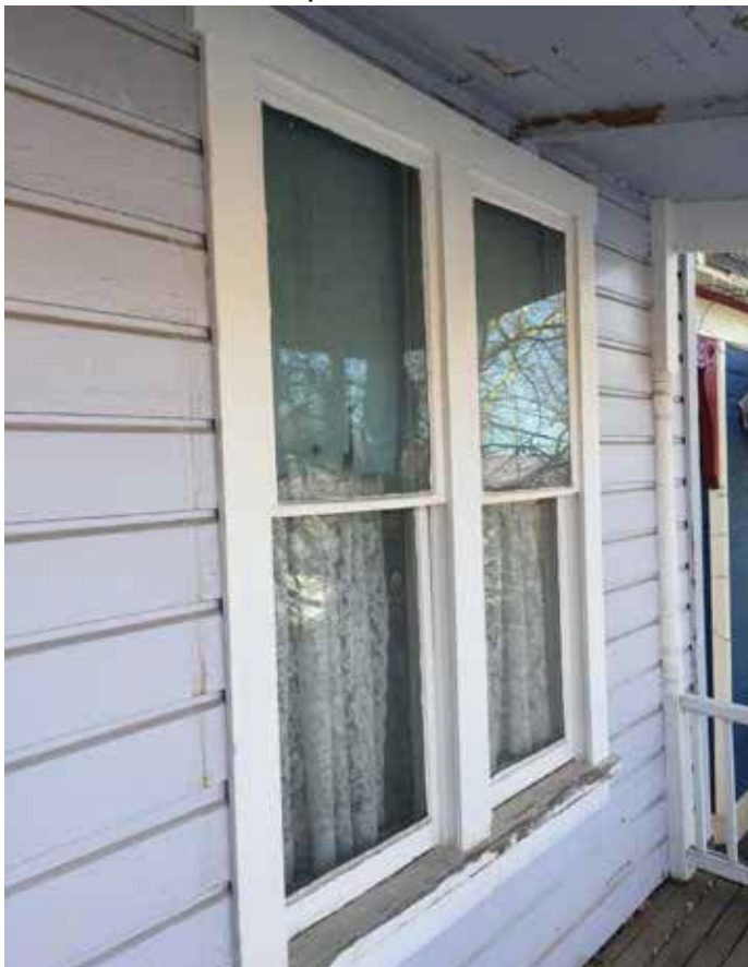
Photo #27: Close Up At Window
