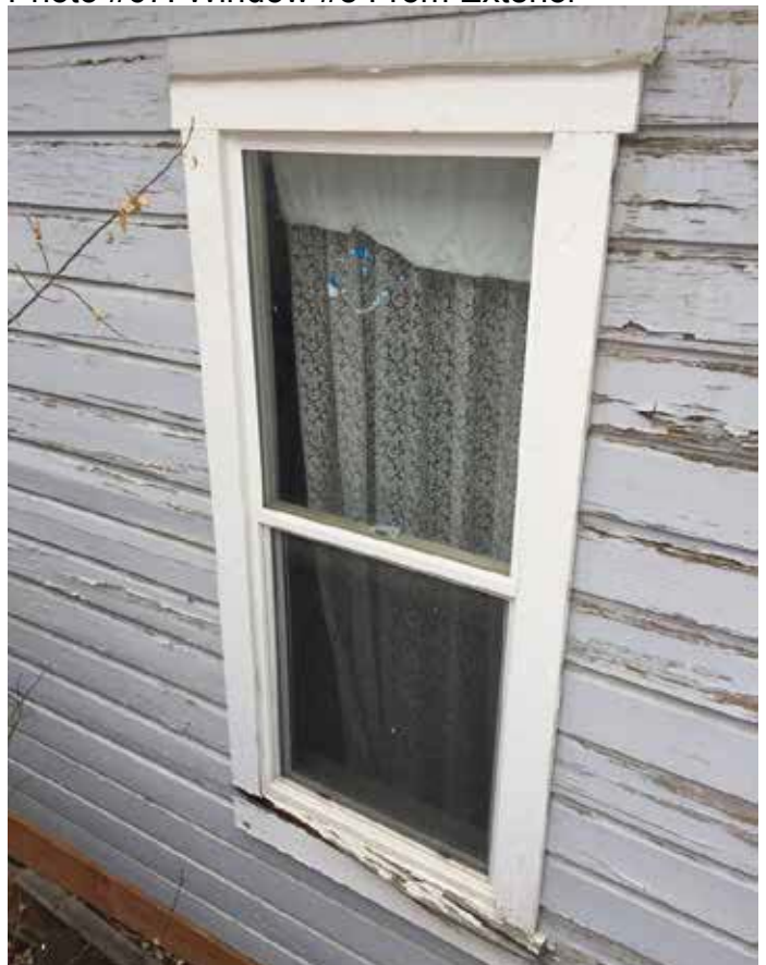
Photo #67: Window #8 From Exterior
