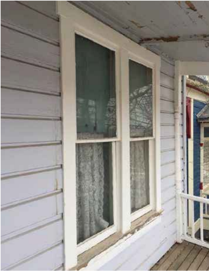
Photo #60: Window #1 From Exterior
