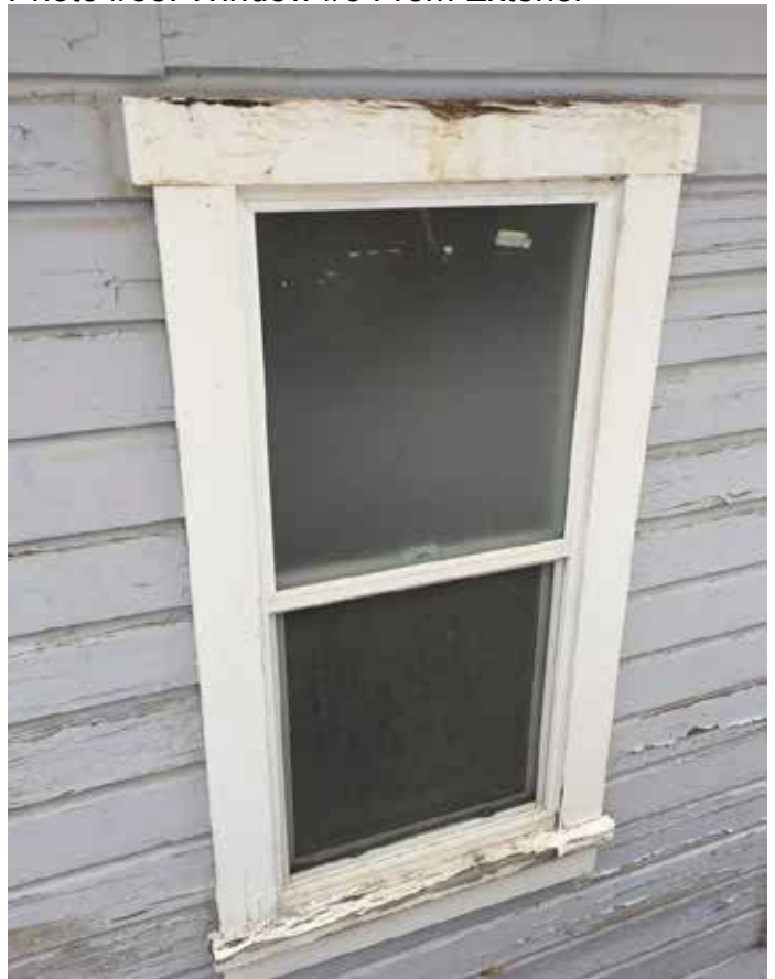
Photo #65: Window #6 From Exterior
