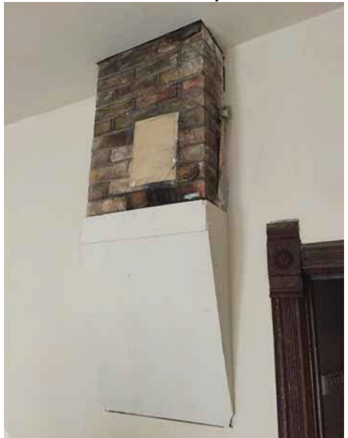
Photo #21: Bottom Of Chimney At Interior
