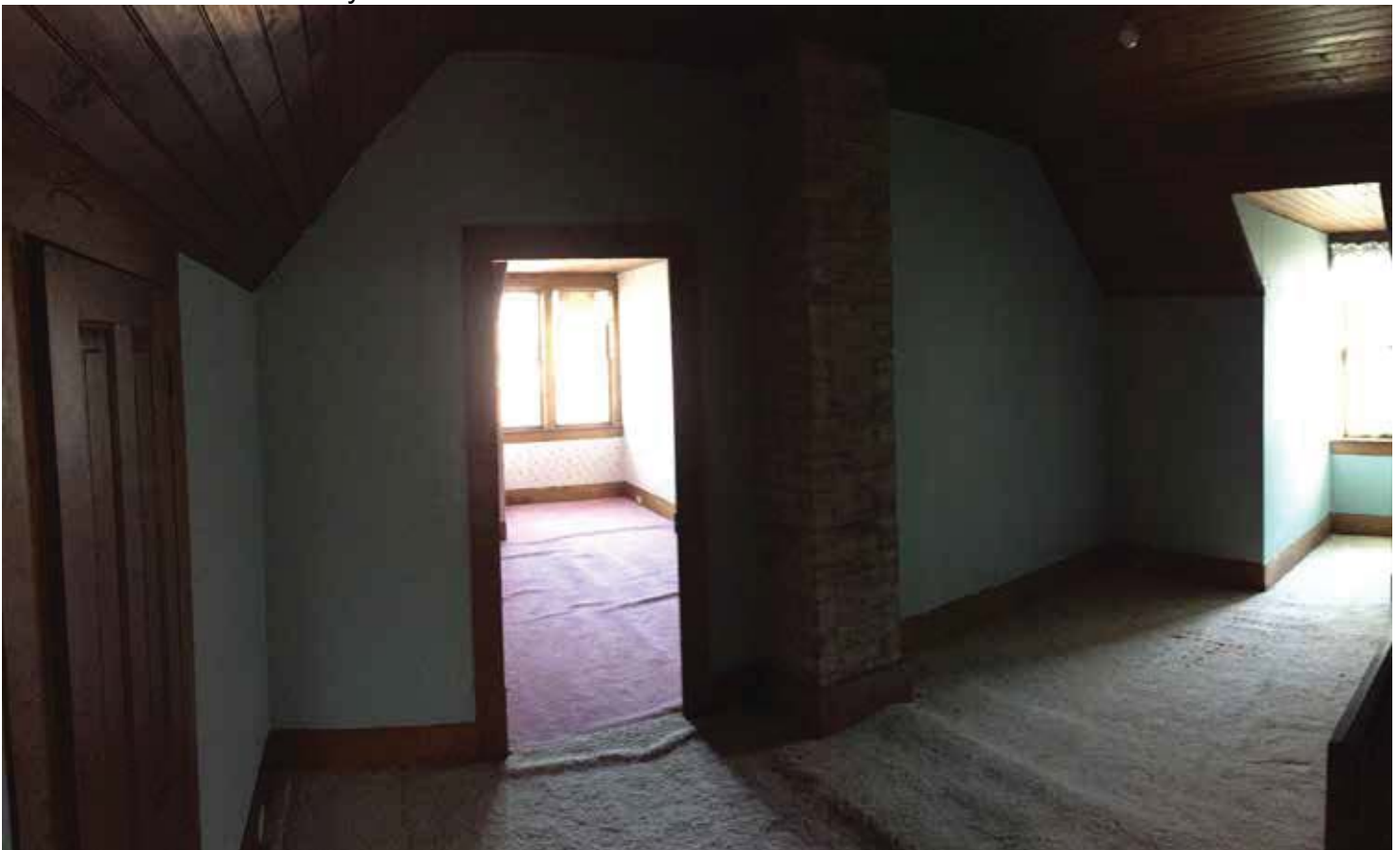
Photo #22: Front Chimney On 2nd Floor
