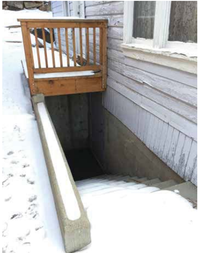
Photo #9: Added Concrete Stair
