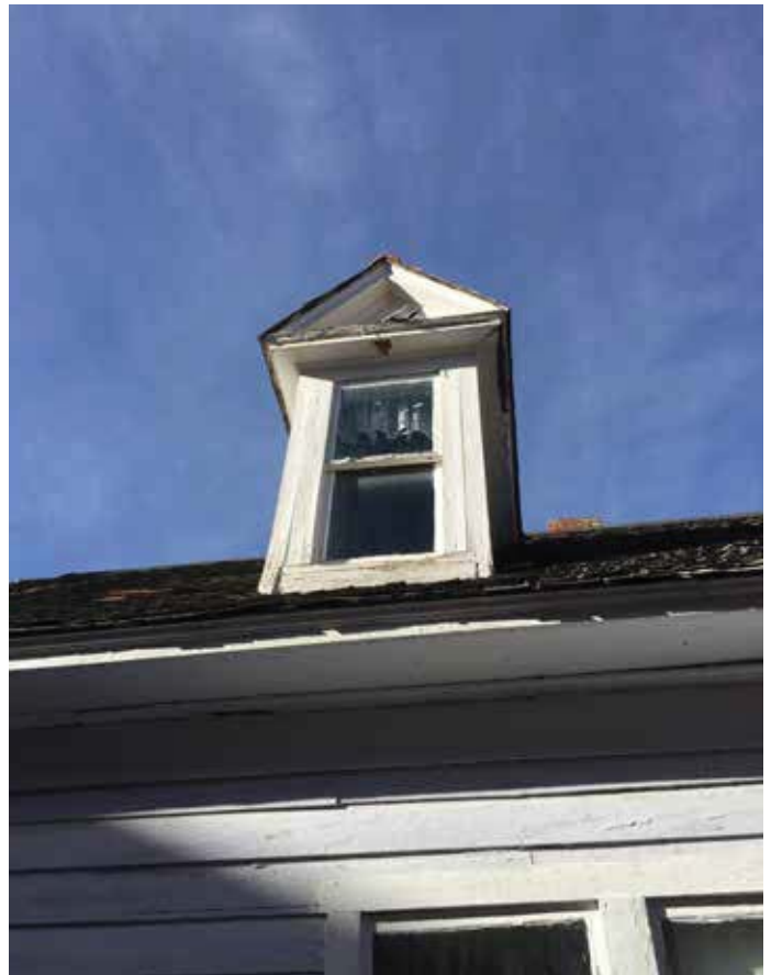
Photo #17: Side Facade Dormer
