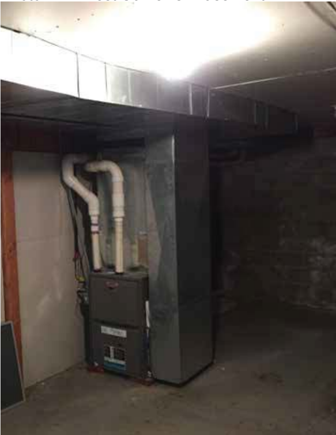
Photo #74: West Corner Of Basement
