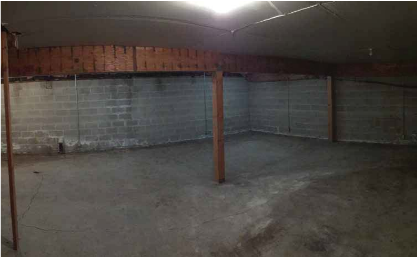
Photo #10: Basement Level Slab With New Beam and Columns Holding Main Level Floor
