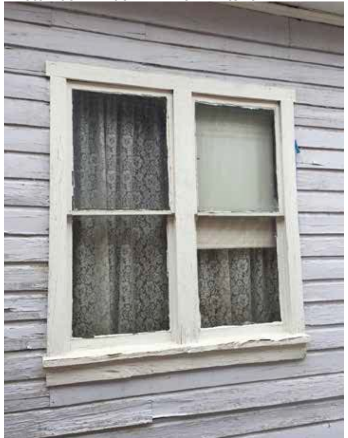
Photo #63: Window #4 From Exterior
