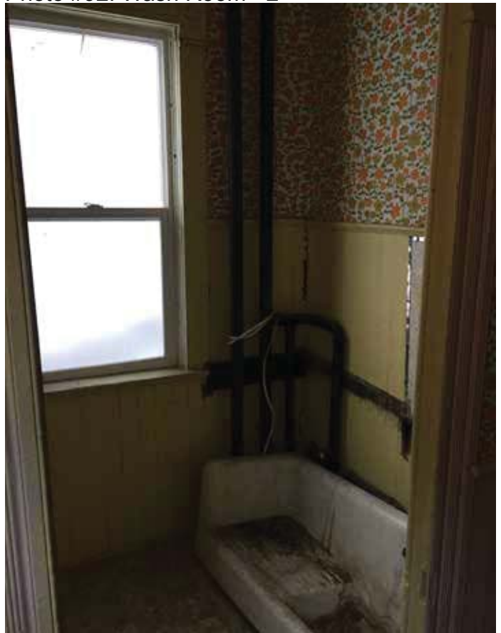
Photo #92: Wash Room - 2
