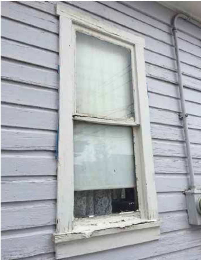
Photo #62: Window #3 From Exterior
