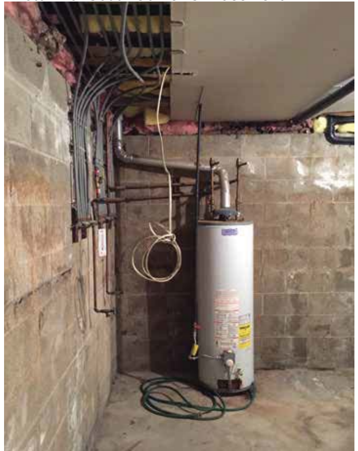
Photo #75: South Corner Of Basement
