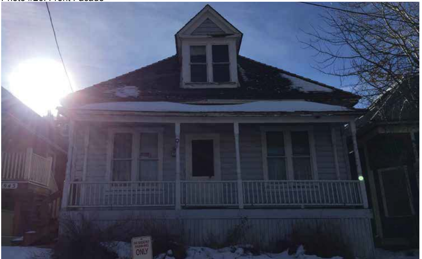
Photo #26: Front Facade
