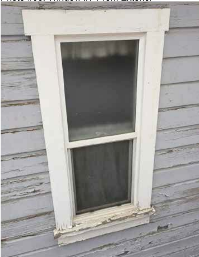
Photo #66: Window #7 From Exterior
