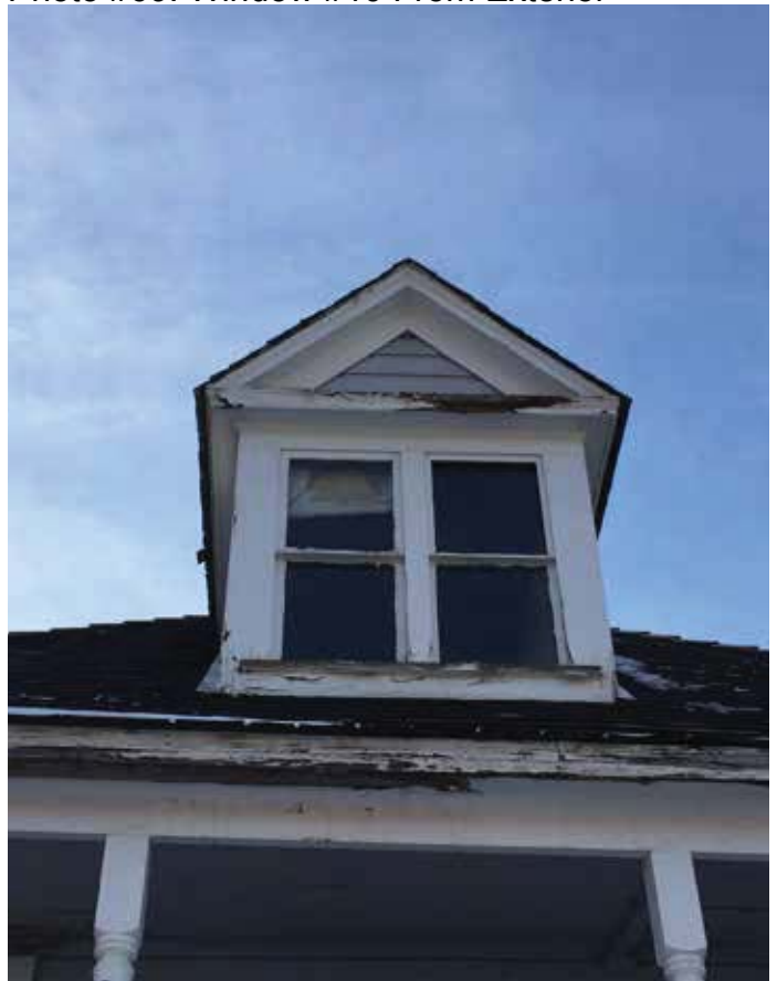
Photo #69: Window #10 From Exterior
