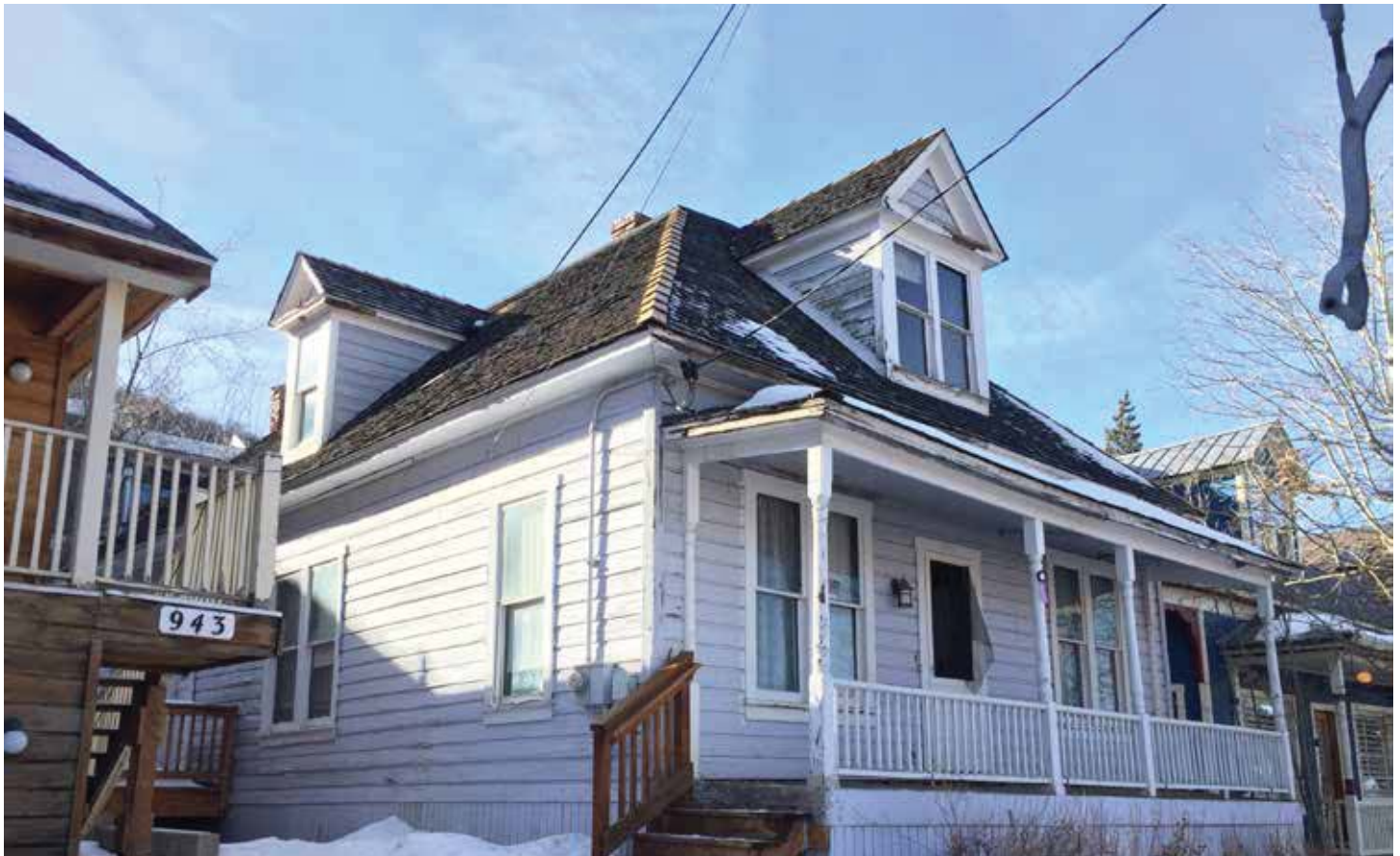
Photo #13: Roof From Northeast Corner
