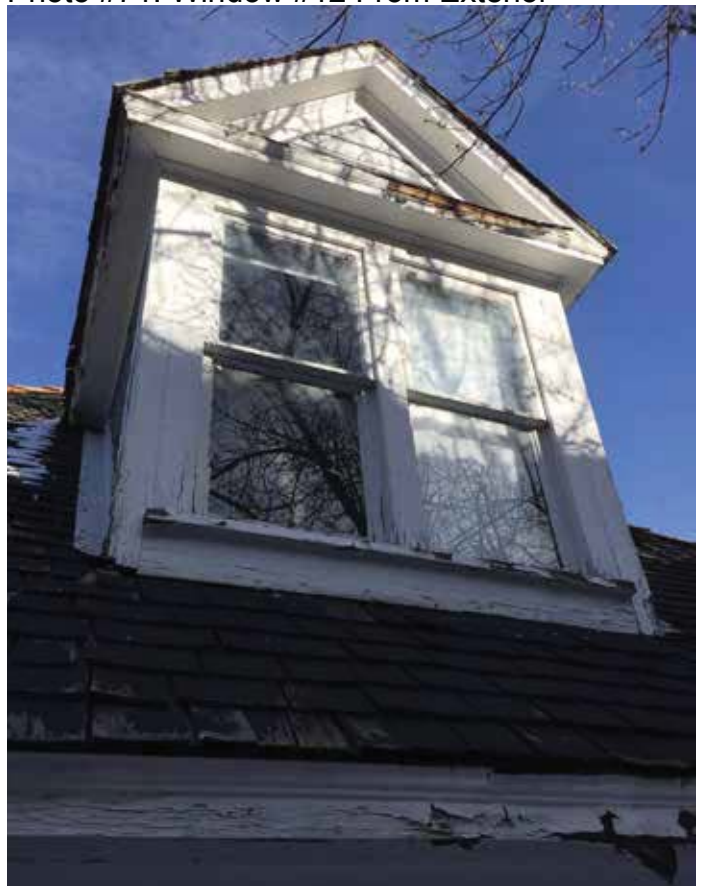
Photo #71: Window #12 From Exterior
