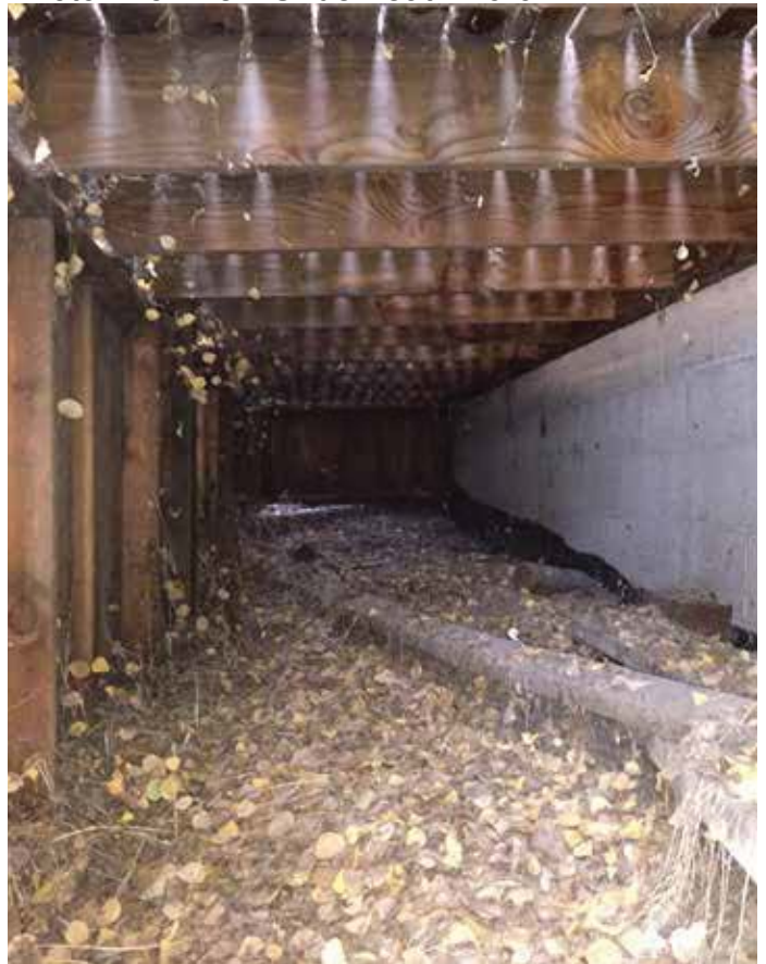
Photo #45: View Underneath Porch
