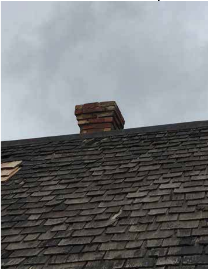
Photo #20: Exterior w/ Front Chimney
