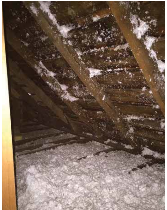
Photo #15: Attic Space Roof Construction
