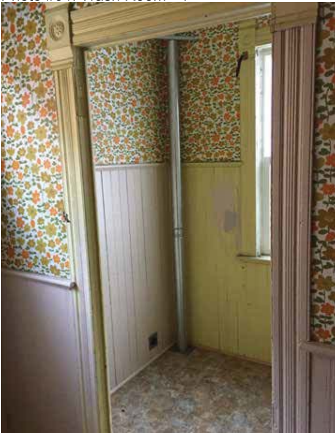
Photo #91: Wash Room - 1
