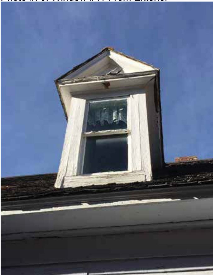
Photo #70: Window #11 From Exterior
