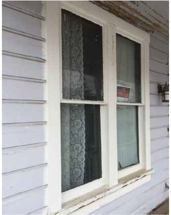
Photo #61: Window #2 From Exterior
