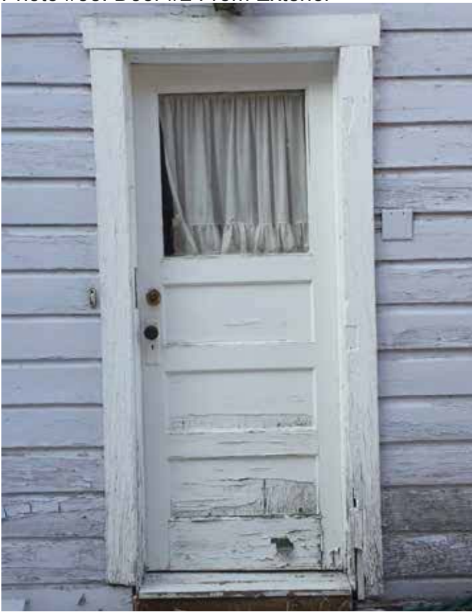
Photo #58: Door #2 From Exterior
