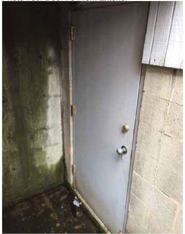
Photo #59: Door #3 From Exterior
