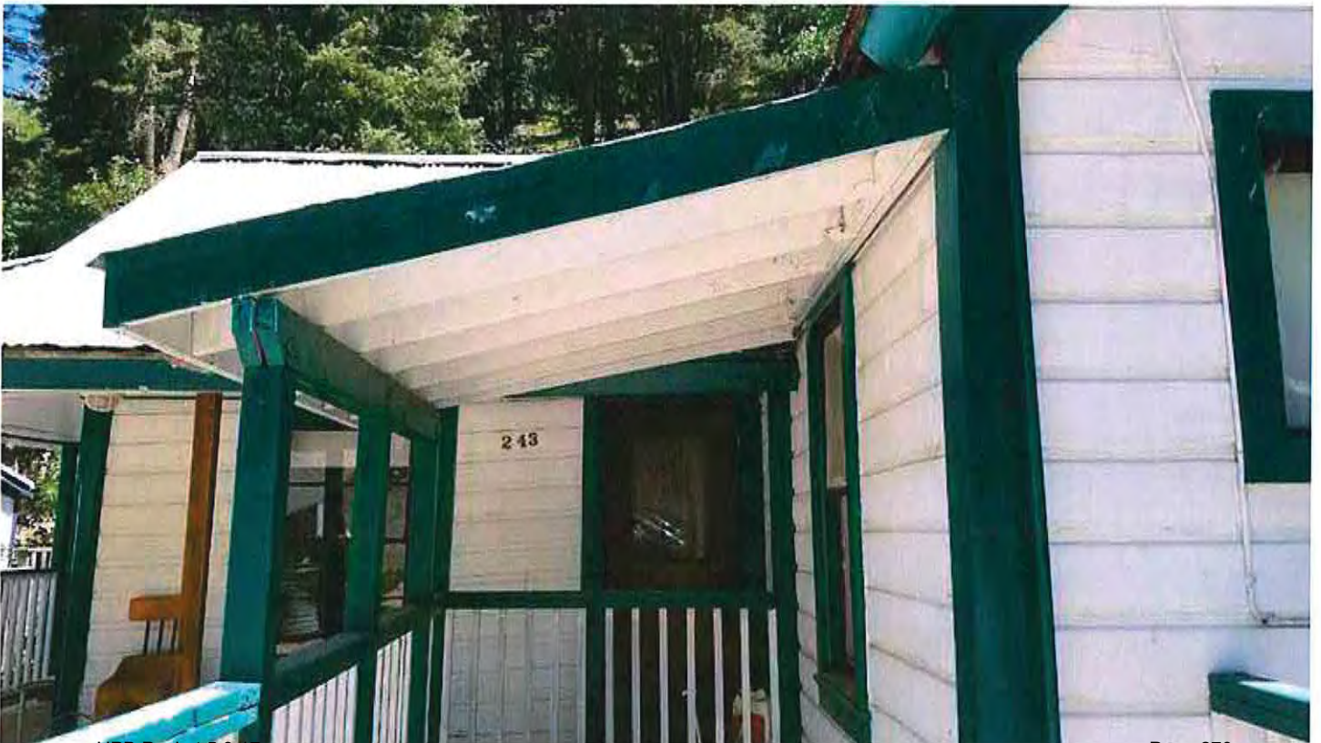
Photo #16: Patio Roof Structure
