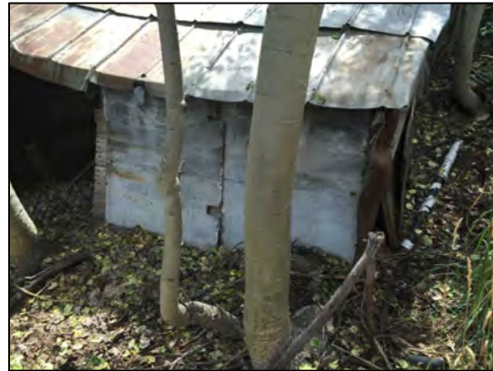
NORTH ELEVATION DETAIL
