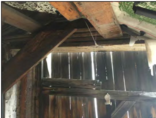
INTERIOR CEILING DETAIL
