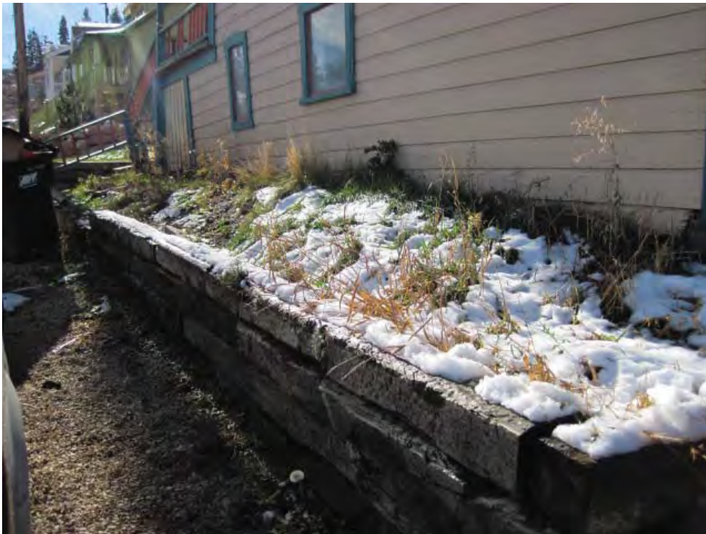
Photo #1: Wood tie retaining wall
