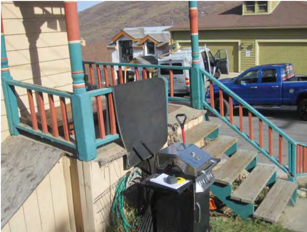
Photo #2: Southeast entry stairs & railing
