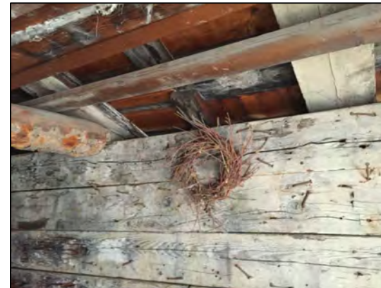
INTERIOR BEAM & WALL DETAIL
