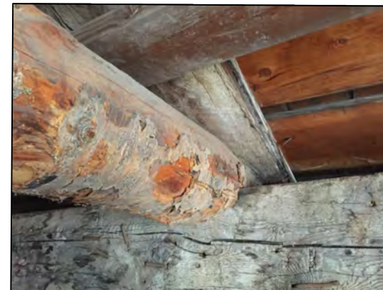
INTERIOR BEAM & WALL DETAIL
