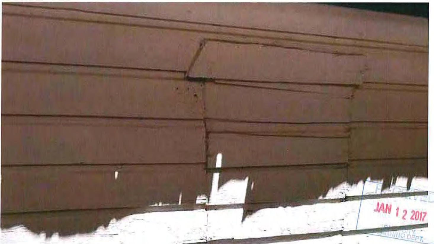
Photo #6: Infilled Window
