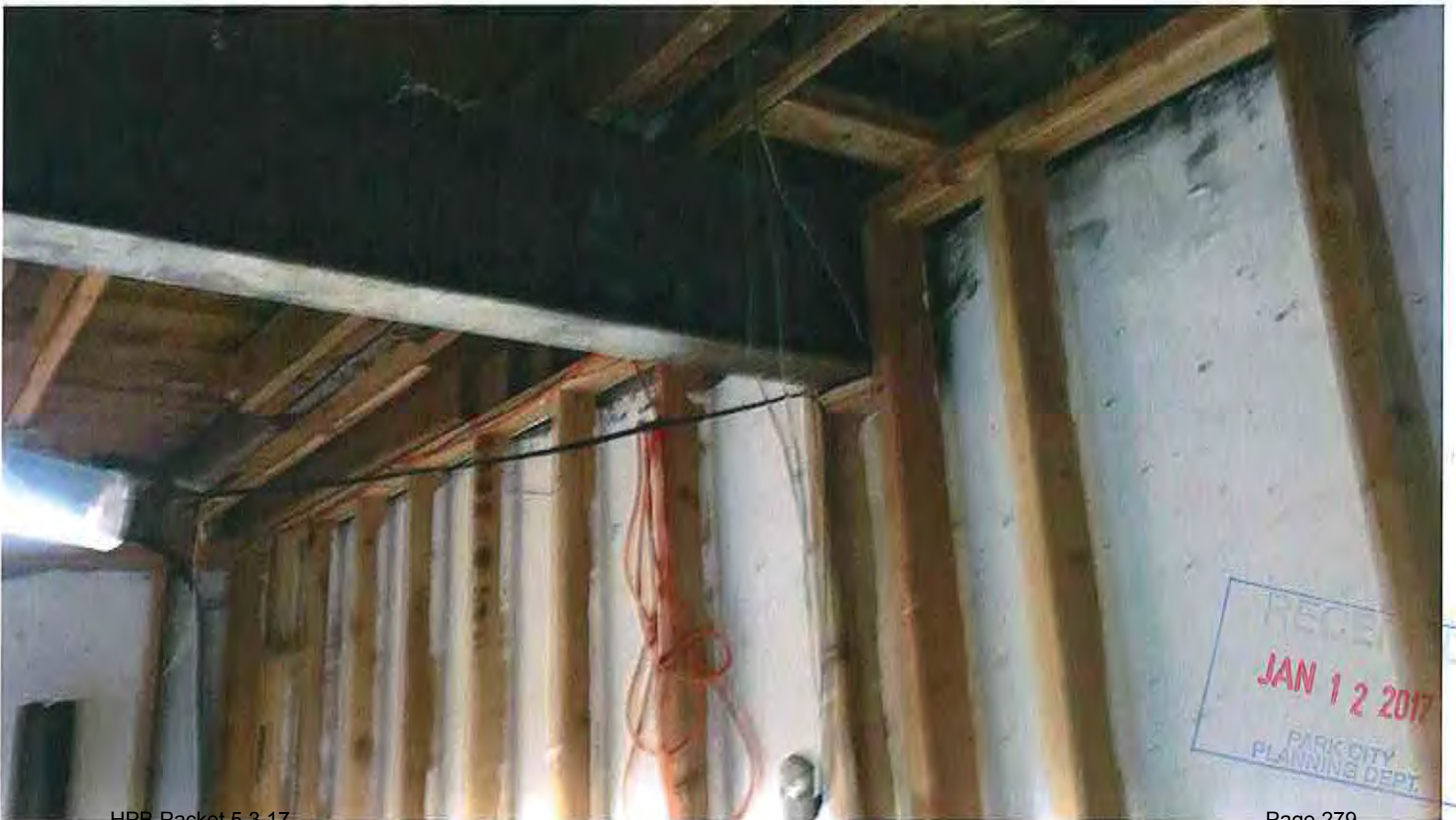
Photo #34: Basement Steel Beam to Foundation Connection
