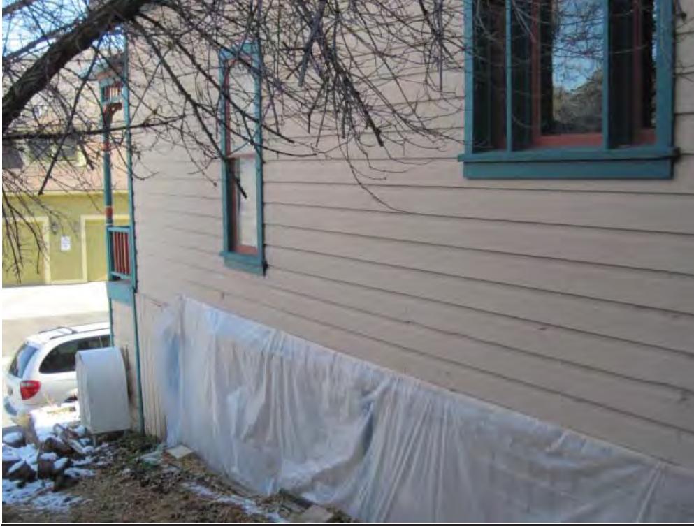
Photo #24: North elevation
