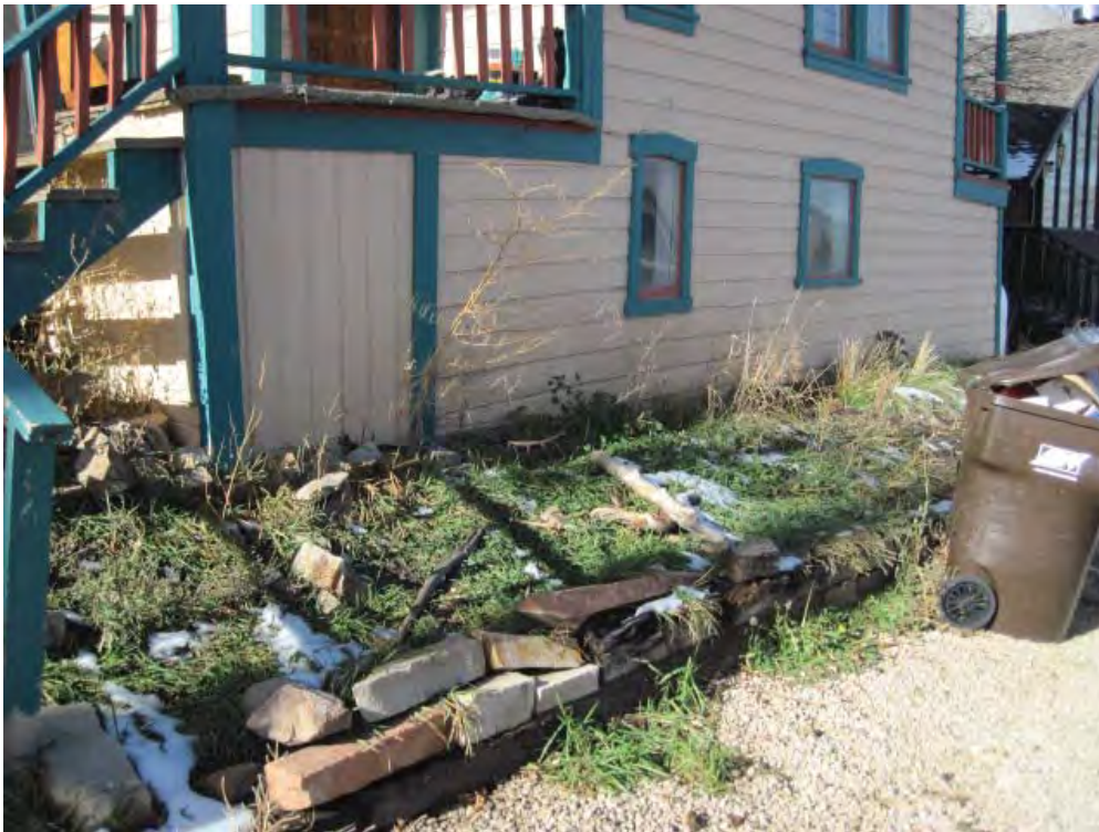
Photo #1A: Wood tie retaining wall
