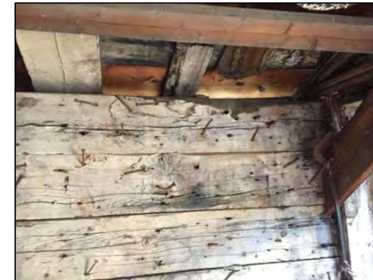
INTERIOR CEILING DETAIL
