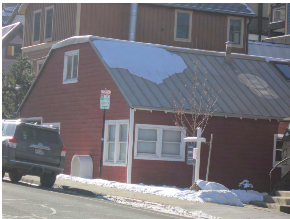
819 Park Avenue. Northeast oblique. November 2013.
