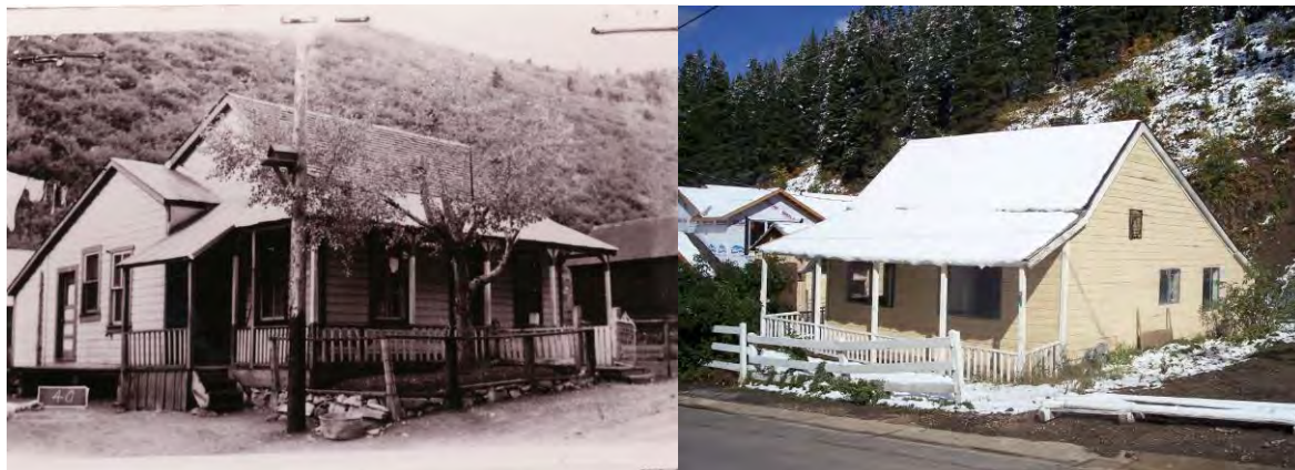
309 Daly Avenue: Window and door configuration has been dramatically changed, altering the historic integrity of the structure.
