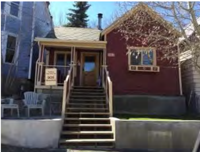
905 Woodside Avenue. Too much of the foundation is exposed. Historically, this house had a stacked stone foundation.
