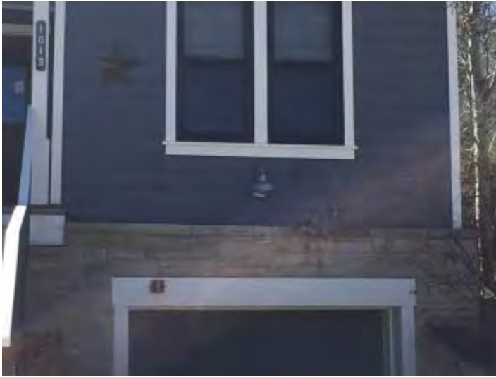
1013 Woodside Avenue. New foundations should not be proud of the historic wall plane.
