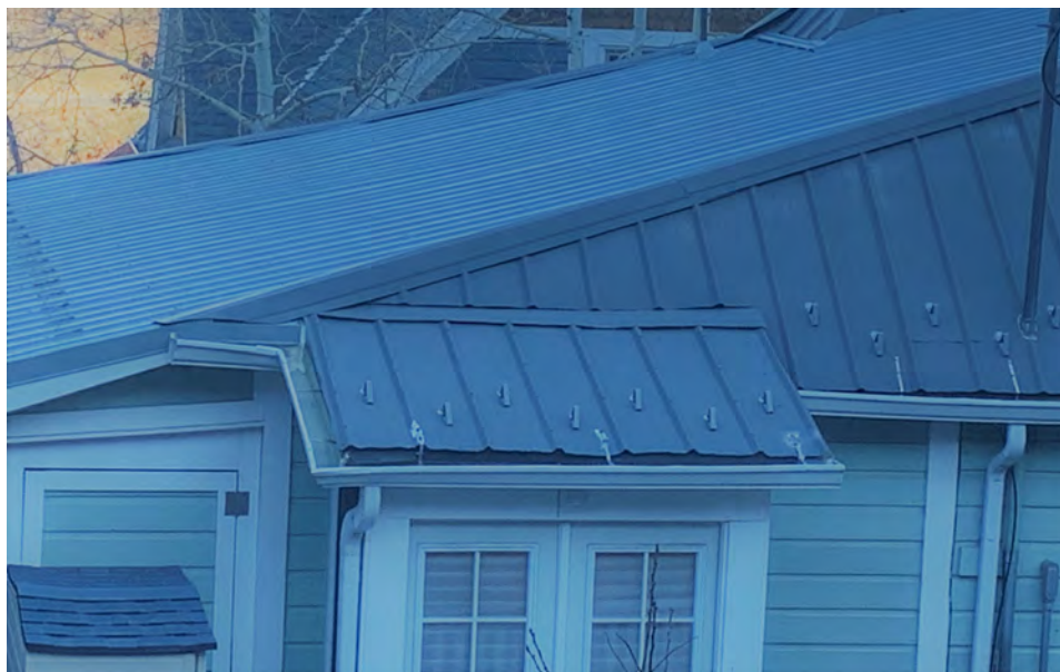
Photo #6: Roof detail
