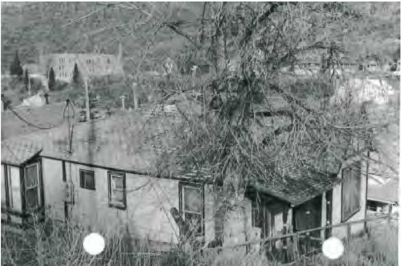
1982 Photo showing West facade & historic bay window
