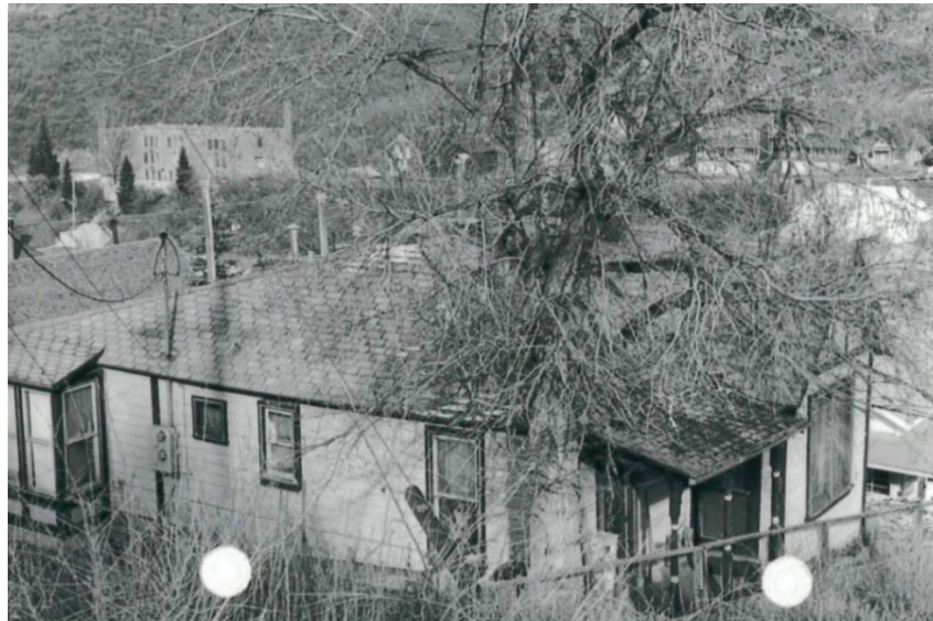
Photo 4: 316 Woodside Avenue in 1982 (Historic Architectural Survey, 1982) From HSI
