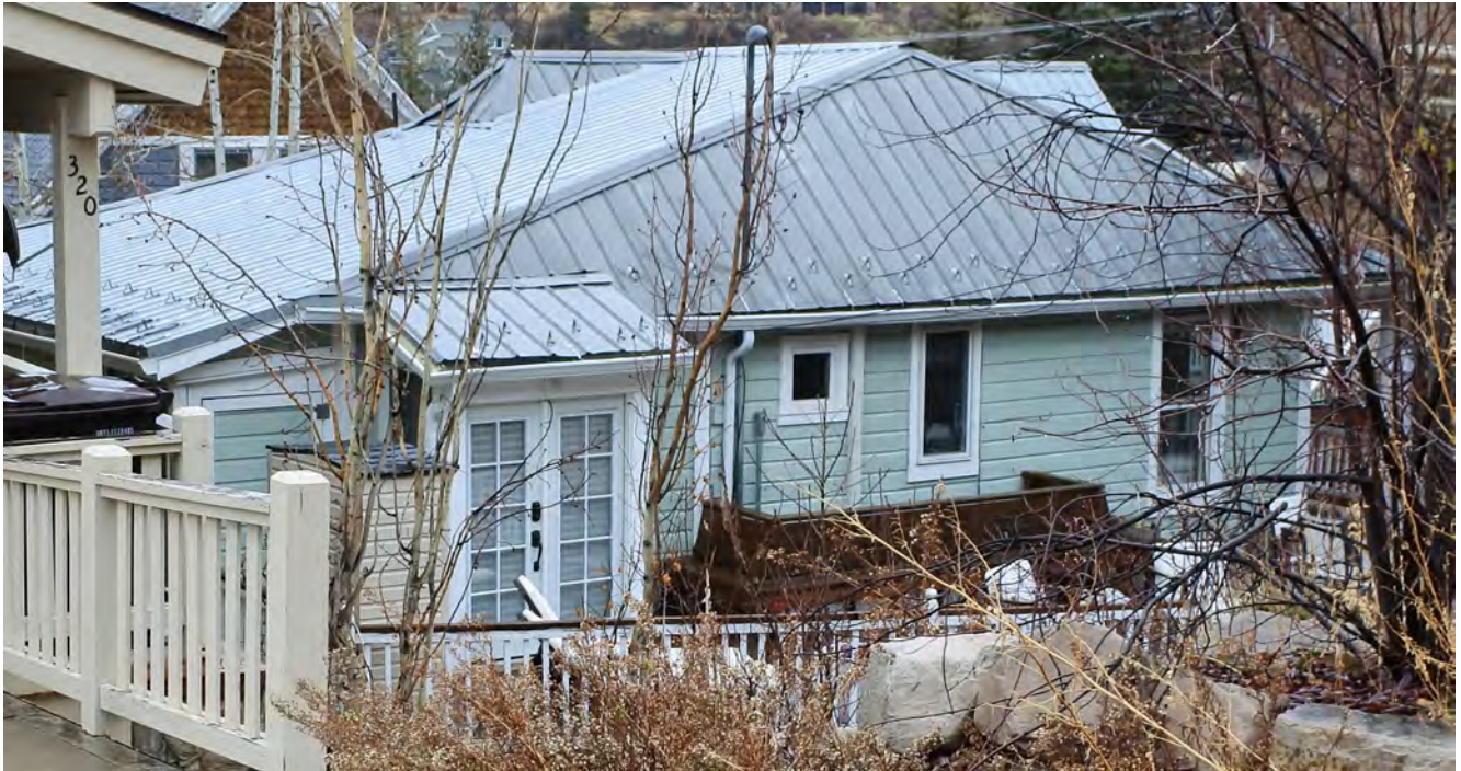
Photo #5: 316 Woodside - Roof
