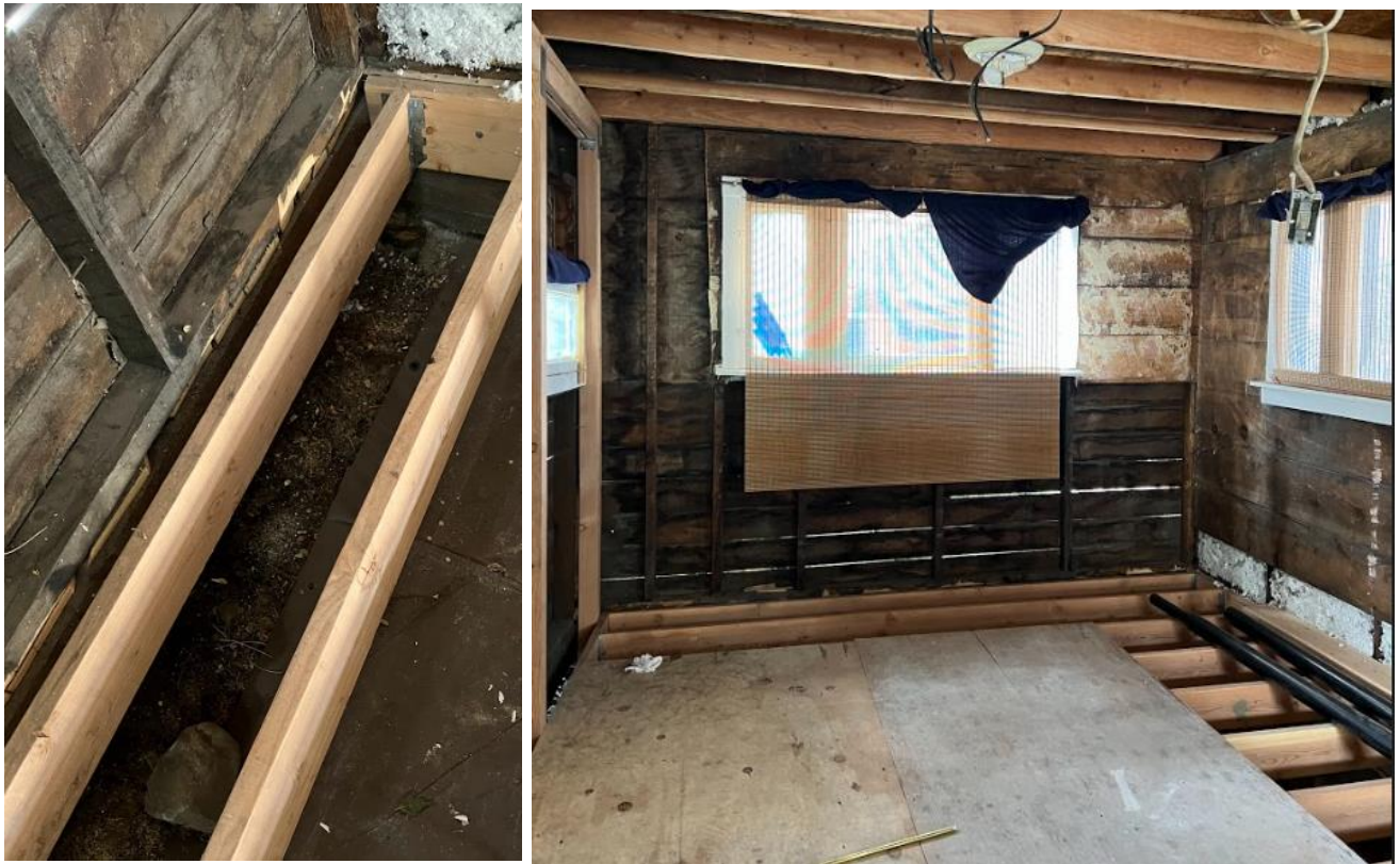
Figure 5 & 6. Existing Conditions, April 26, 2022
